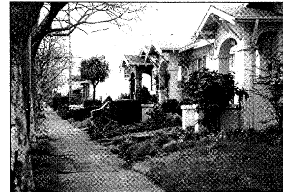
Buildings should address and "enliven" the street with awnings, entries, windows, porches and other special features.
