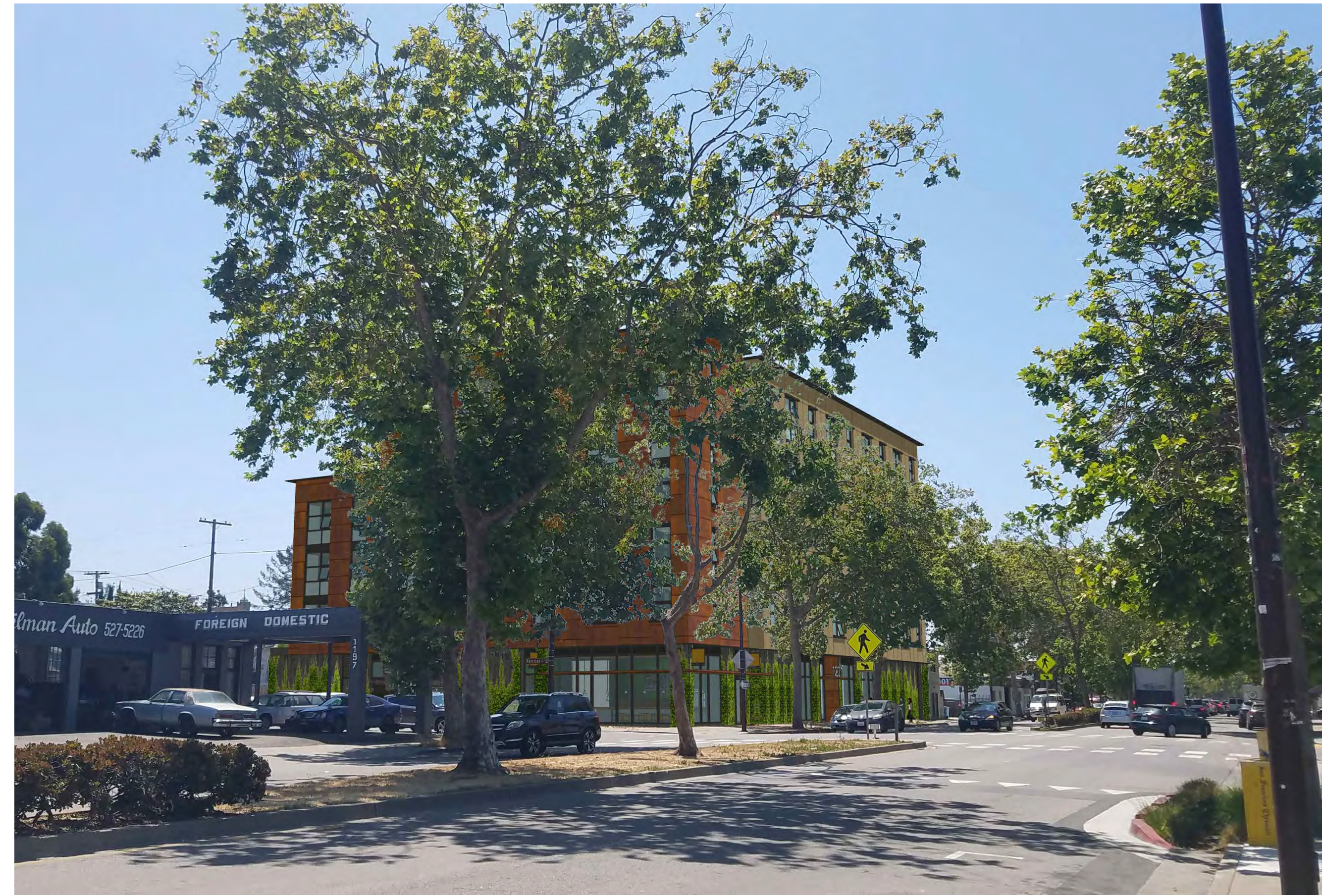
2 SAN PABLO LOOKING SOUTH - AFTER
