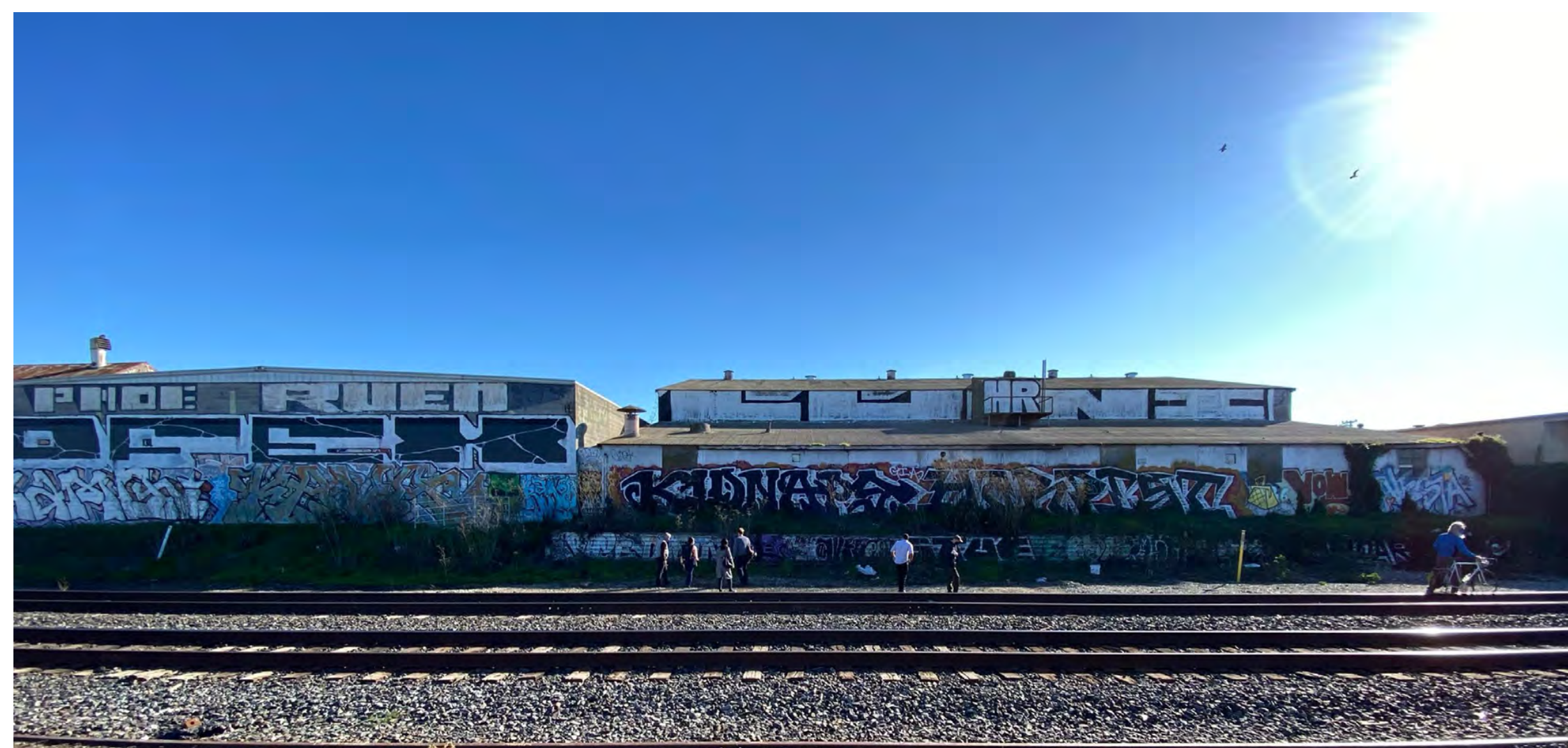
VIEW FROM RAILROAD CROSSING: EXISTING
