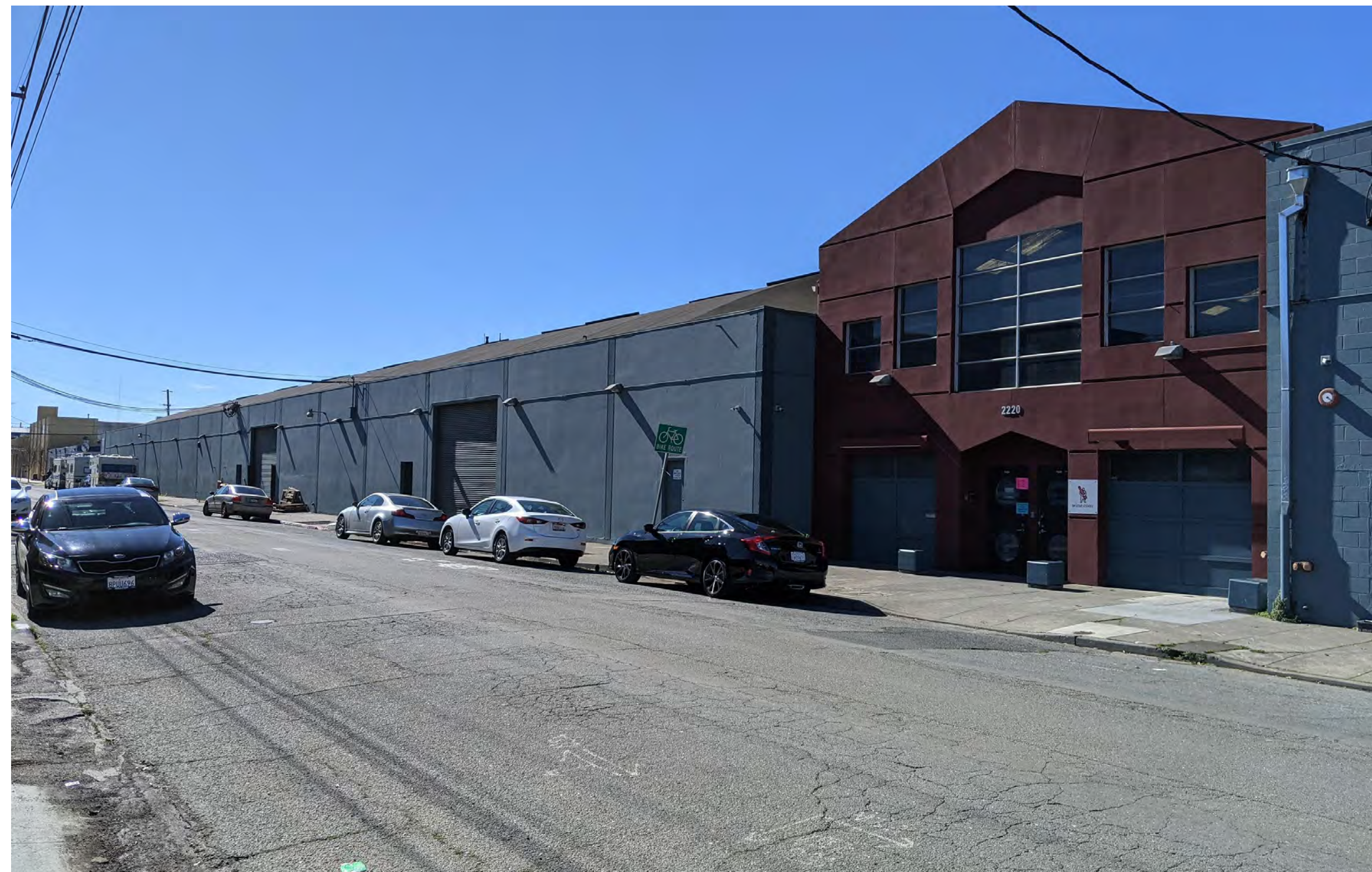
VIEW FROM 4TH STREET: EXISTING
