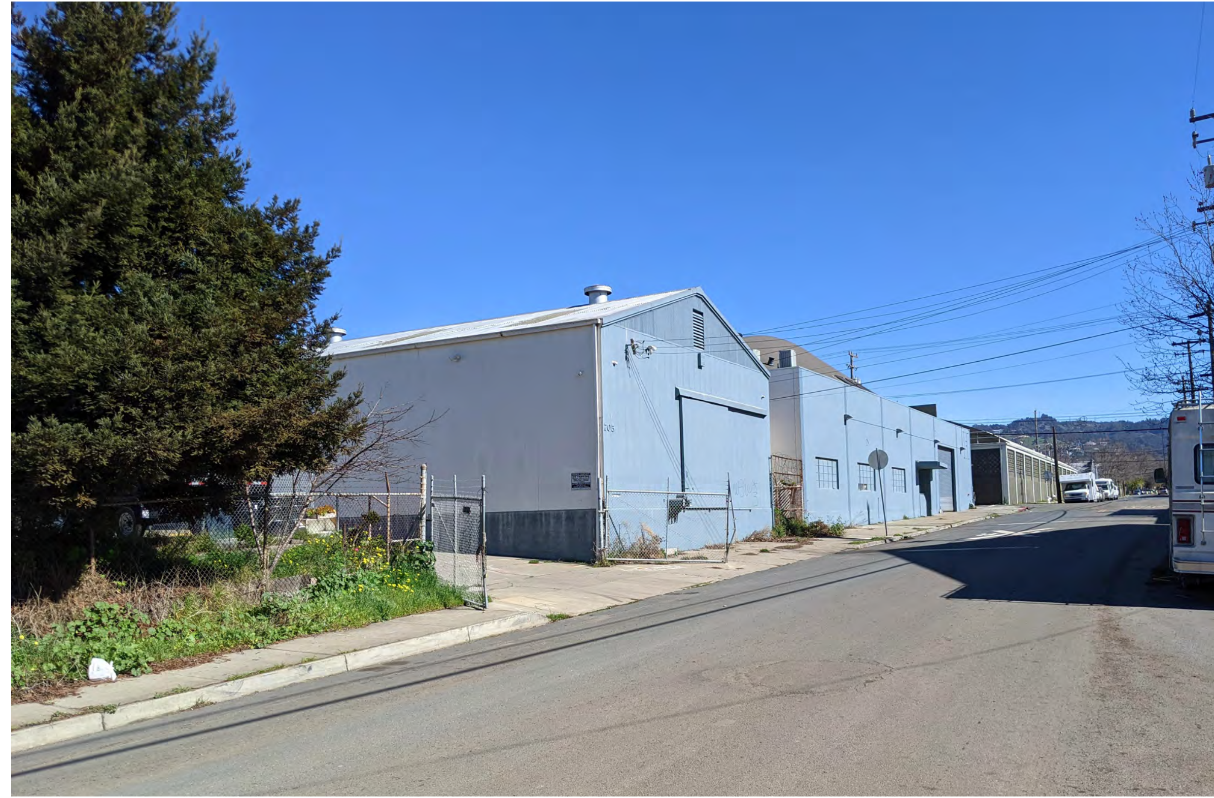
VIEW FROM BANCROFT WAY: EXISTING
