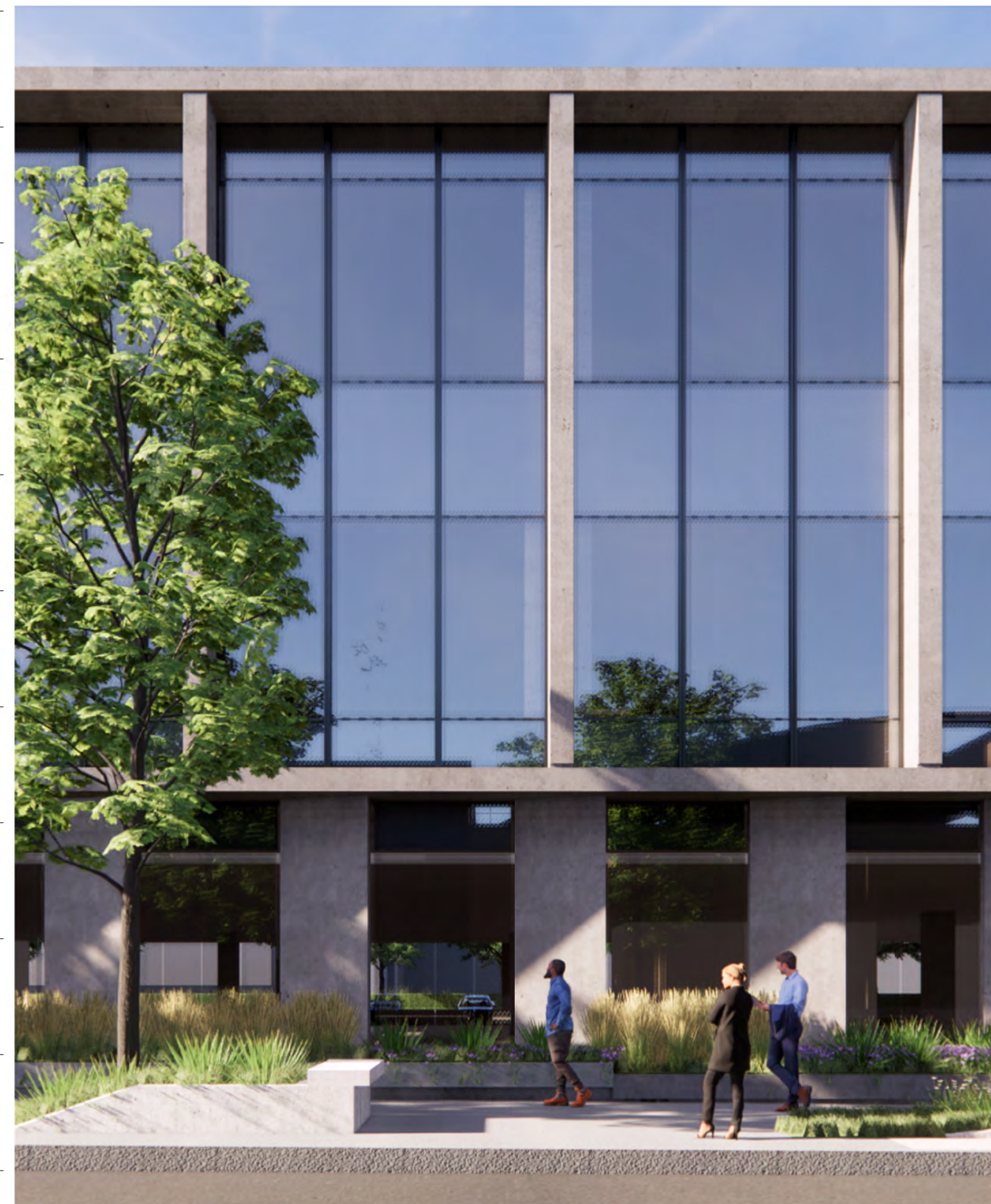
EXTERIOR VIEW AT TYPICAL FACADE (4TH STREET)
