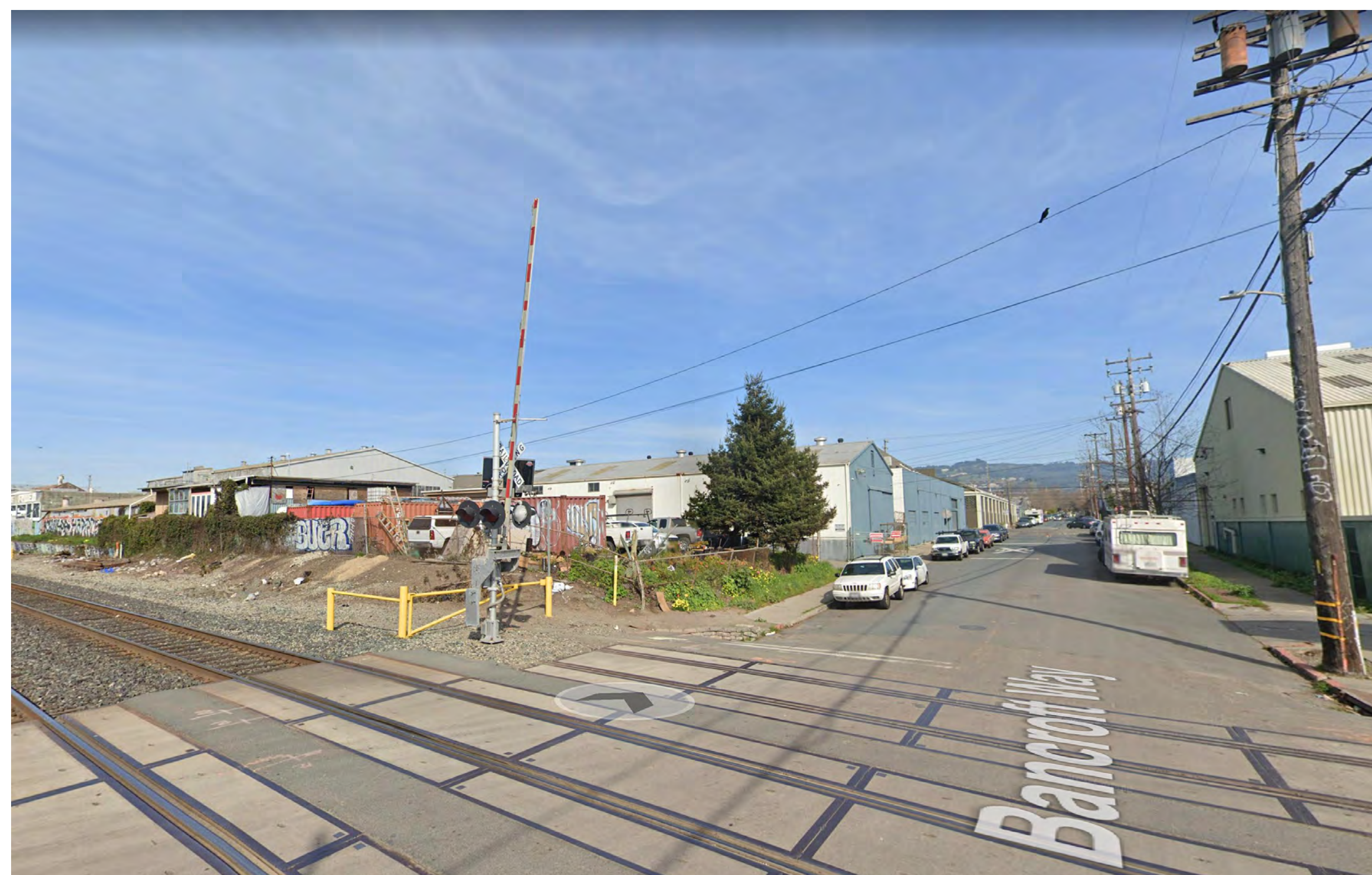
VIEW FROM RAILROAD CROSSING: EXISTING
