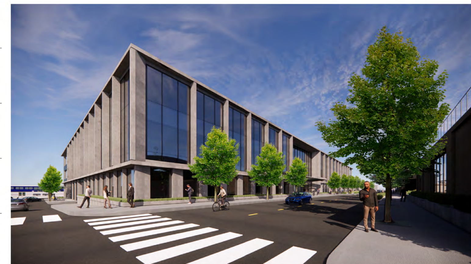
EXTERIOR VIEW AT SE CORNER
