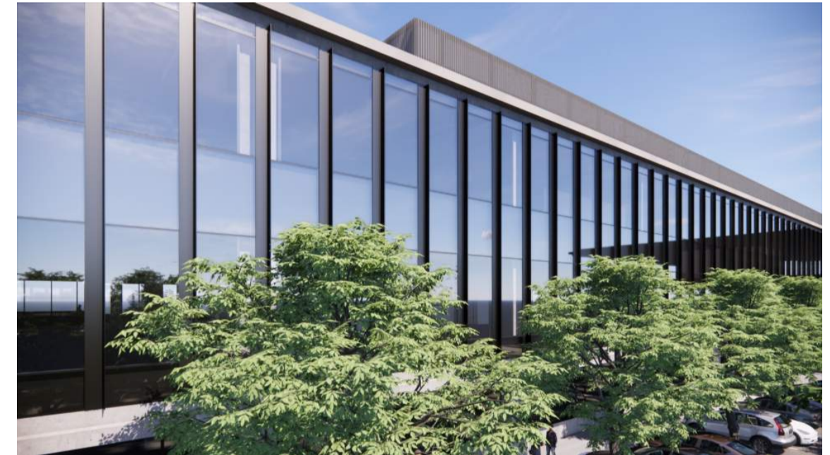
2: Inner West facade solid metal panels and decorative fins
