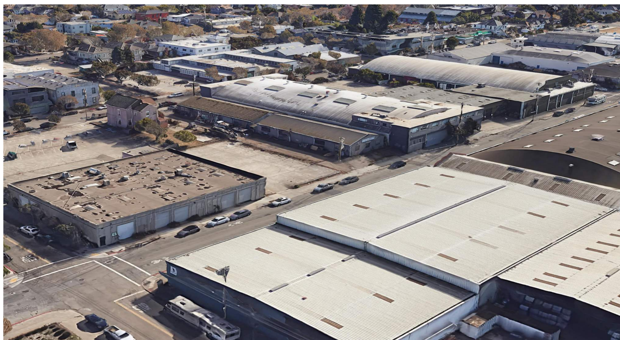
EXISTING AERIAL VIEW FROM NORTHWEST
