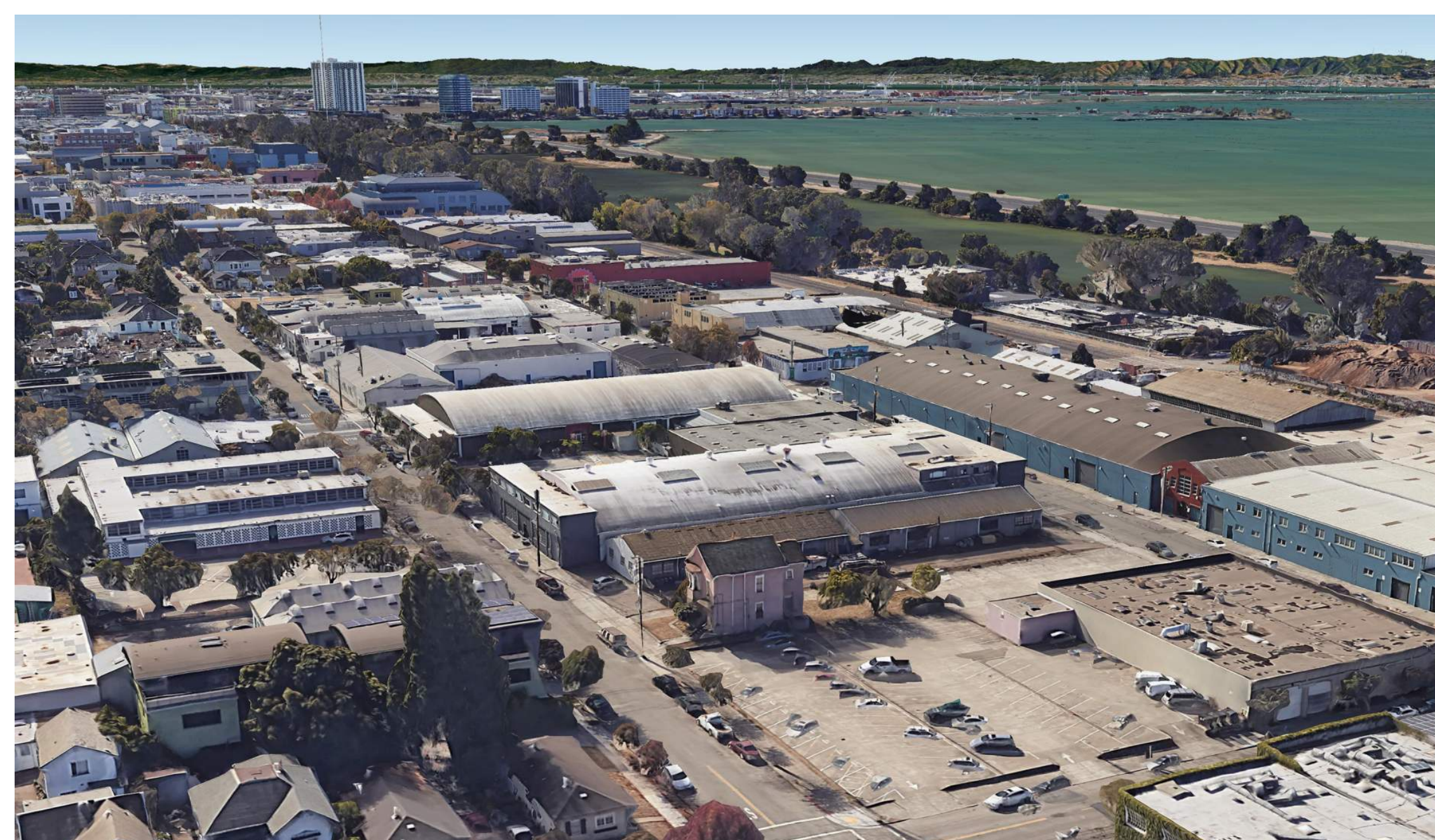
EXISTING AERIAL VIEW FROM NORTHEAST
