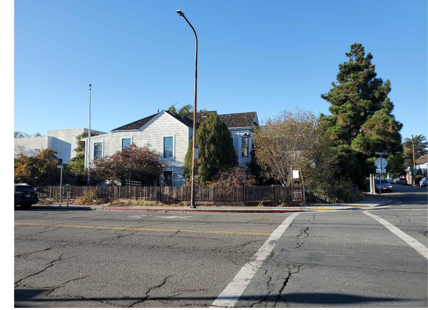
5 HEARST AVE VIEW LOOKING NORTH
