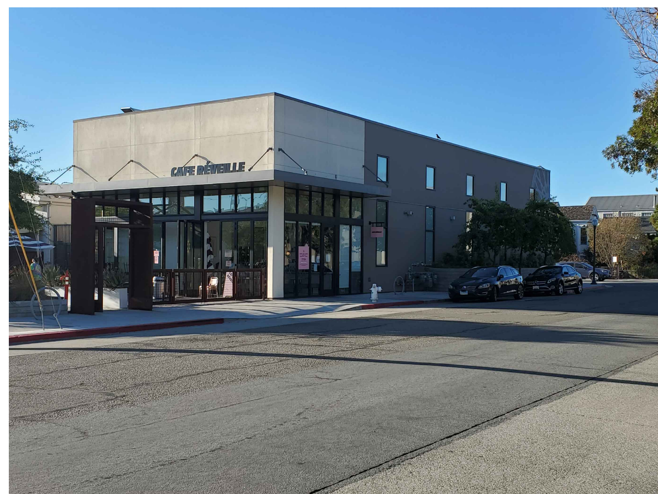
3 FIFTH STREET VIEW LOOKING NORTH
