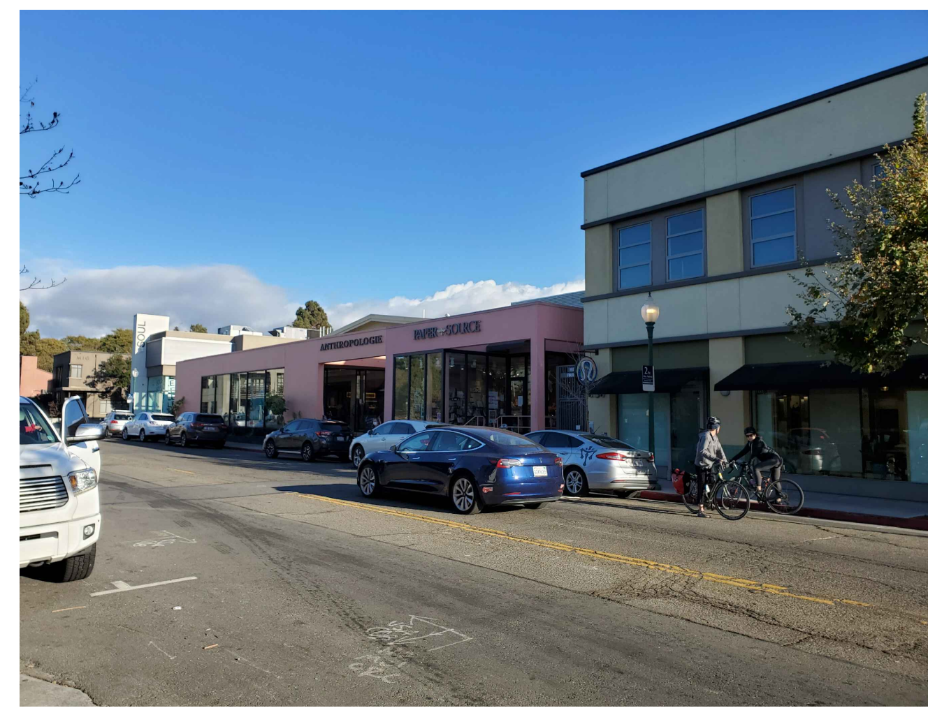
9 HEARST AVE VIEW LOOKING SOUTHEAST
