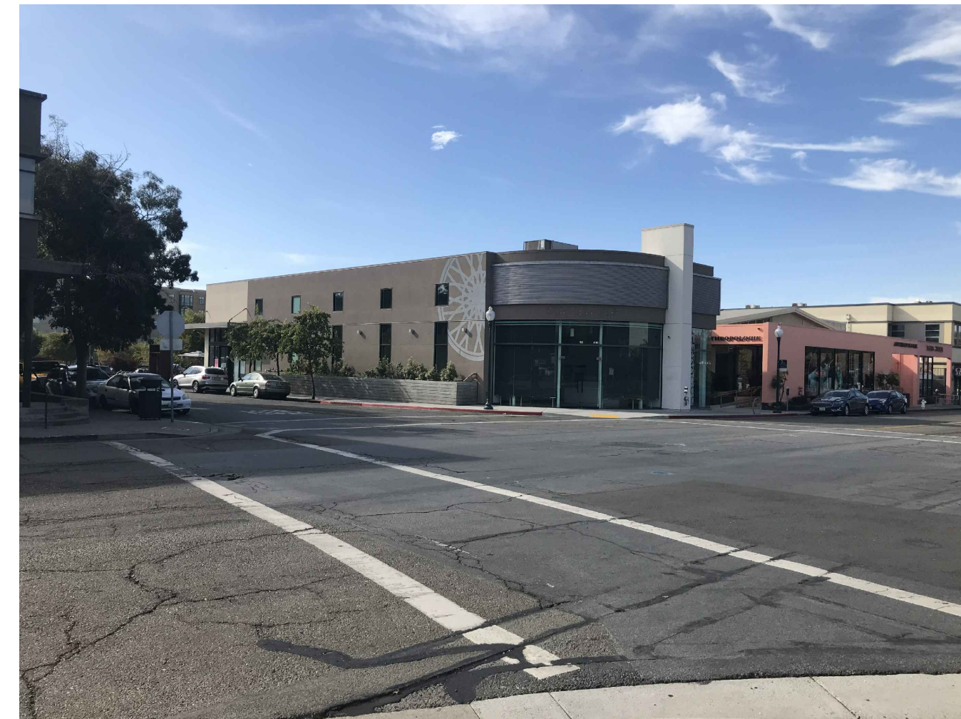
2 FIFTH & HEARST VIEW LOOKING SOUTHWEST
