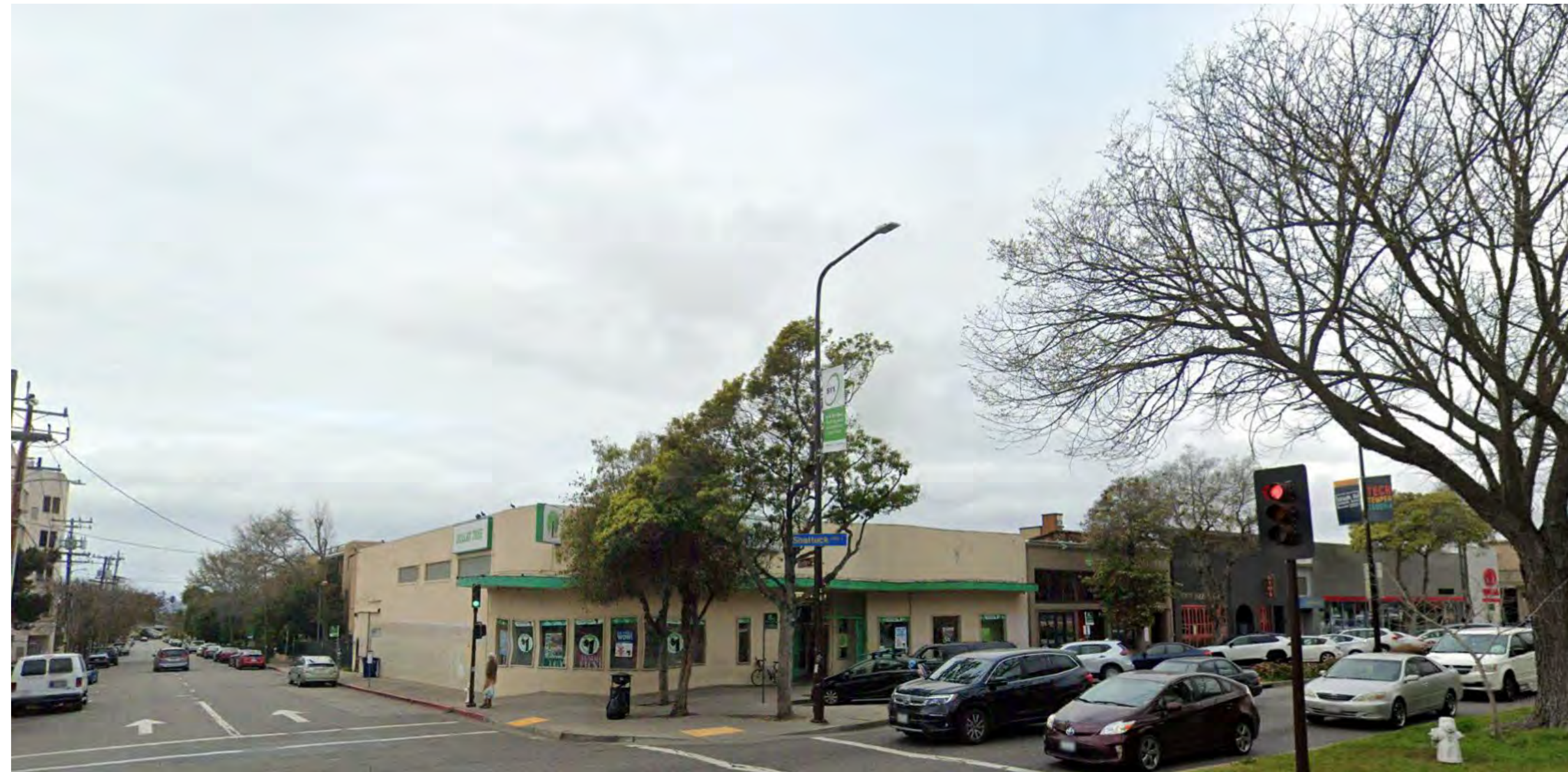
View from Shattuck Avenue looking Northwest
