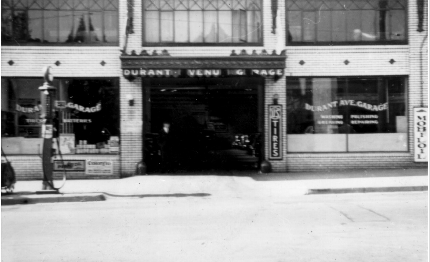
Image of portion of front (south) facade of Durant Avenue Garage; date unknown, before alteration. (BAHA)
