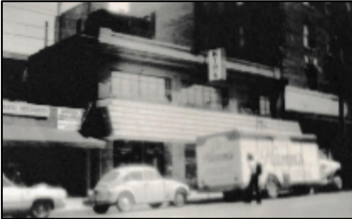
Figure 5: Subject Property – South Elevation, 1970s (Berkeley Architectural Heritage Association Survey Form)
