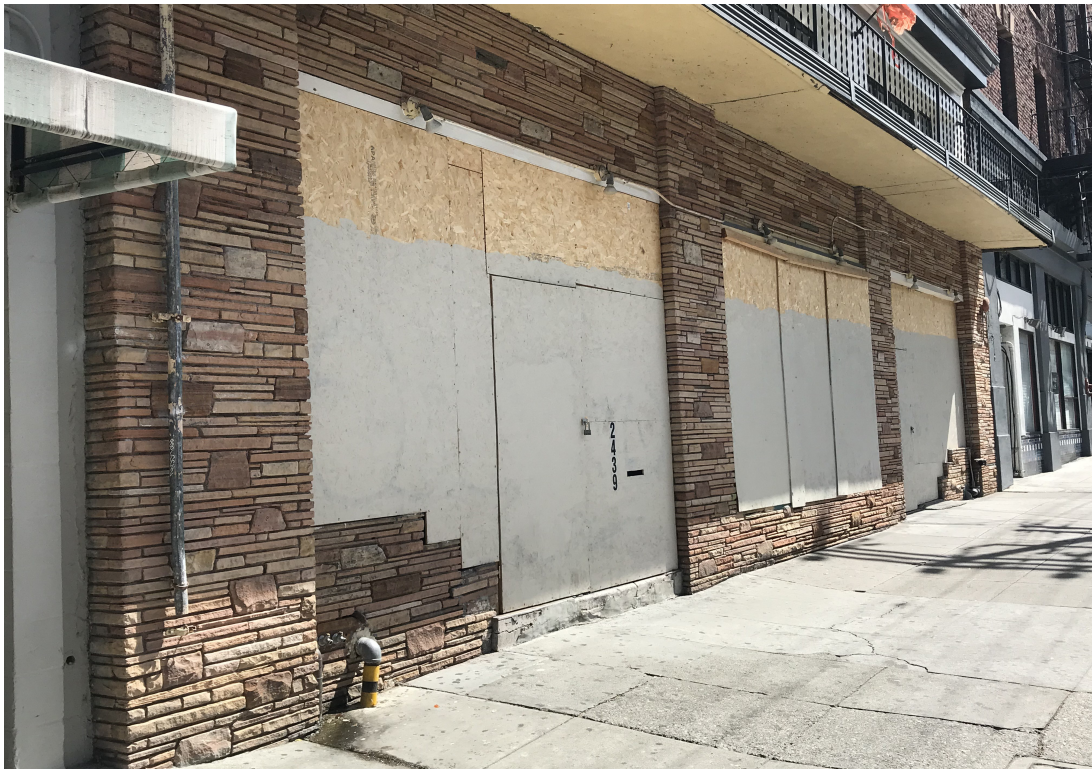
Primary facade, first story, looking northeast.
