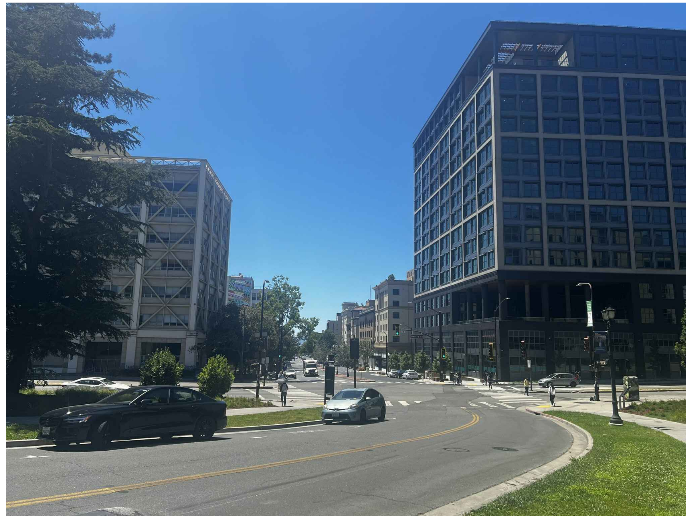
1 UNIVERSITY LOOKING WEST - BEFORE A3.6
