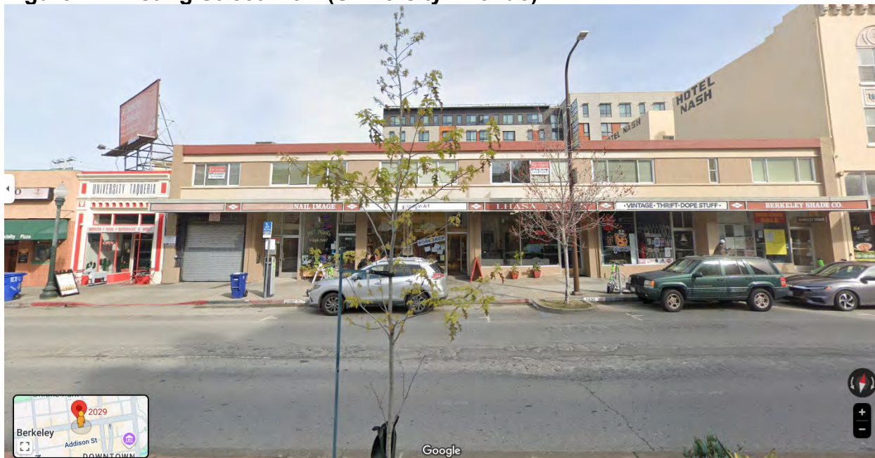
Figure 2: Existing Street View (University Avenue)
