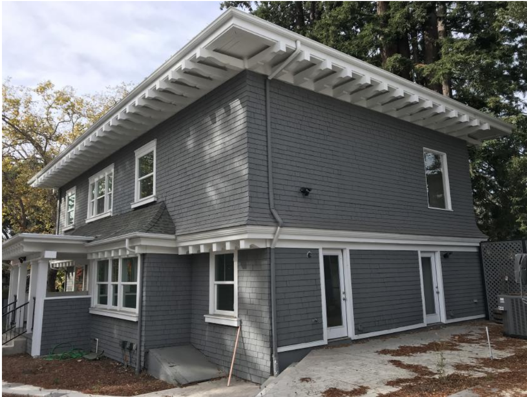
View of primary (east) and north facade from yard, looking southwest.
