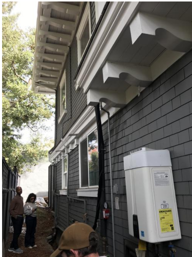
View of north side of rear (west) facade, looking north.
