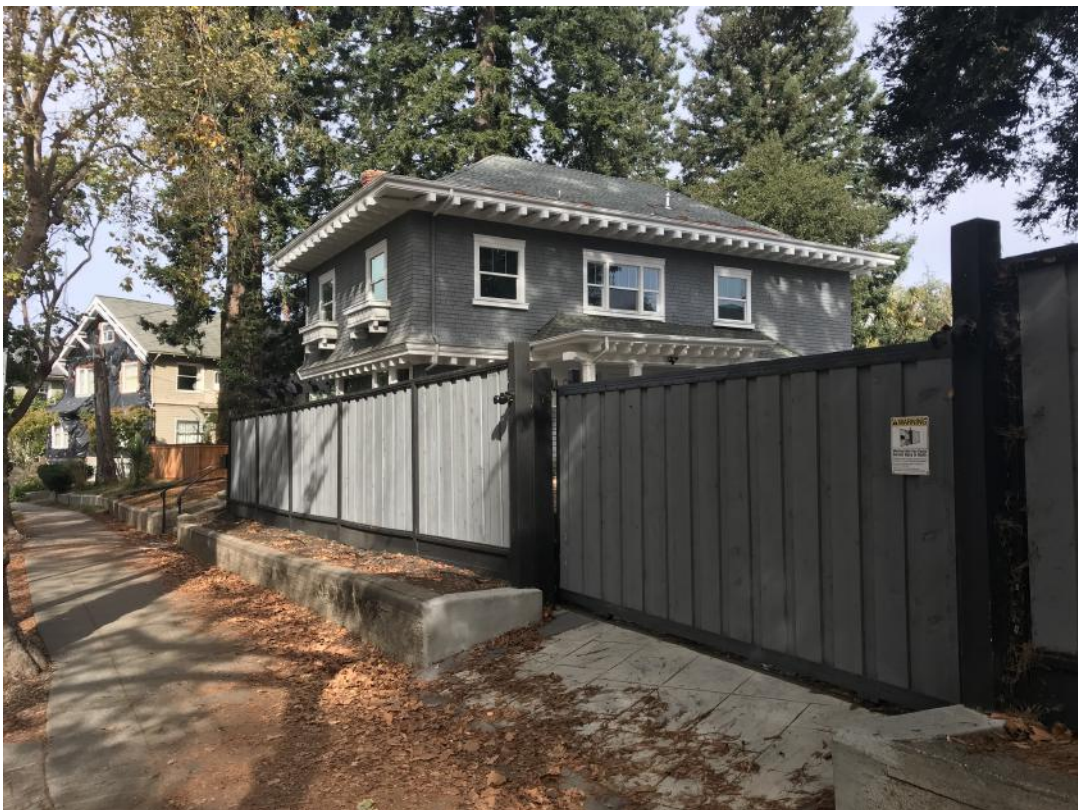
View of south and primary (east) facades from Woolsey Street, looking northwest.
