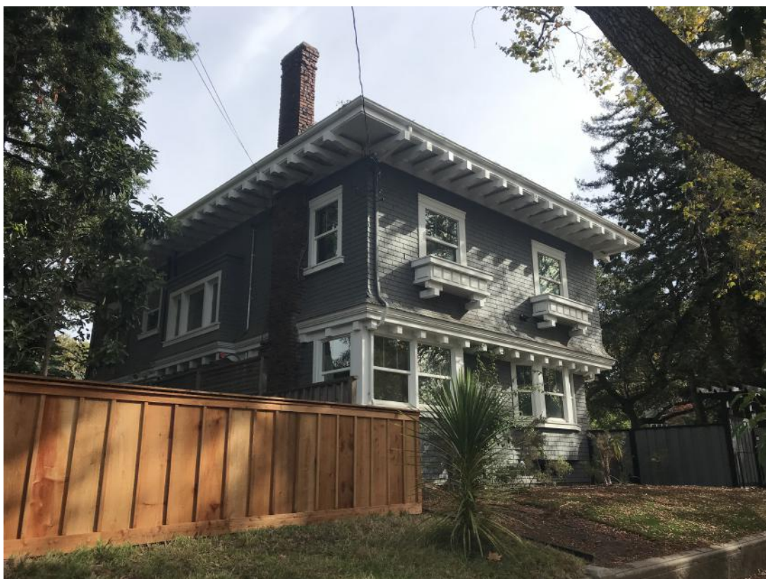
View of rear (west) and south facades from Woolsey Street, looking northeast.
