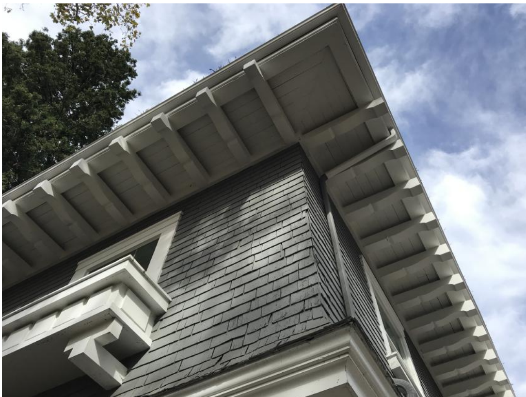
Detail of eaves, southeast corner of house.
