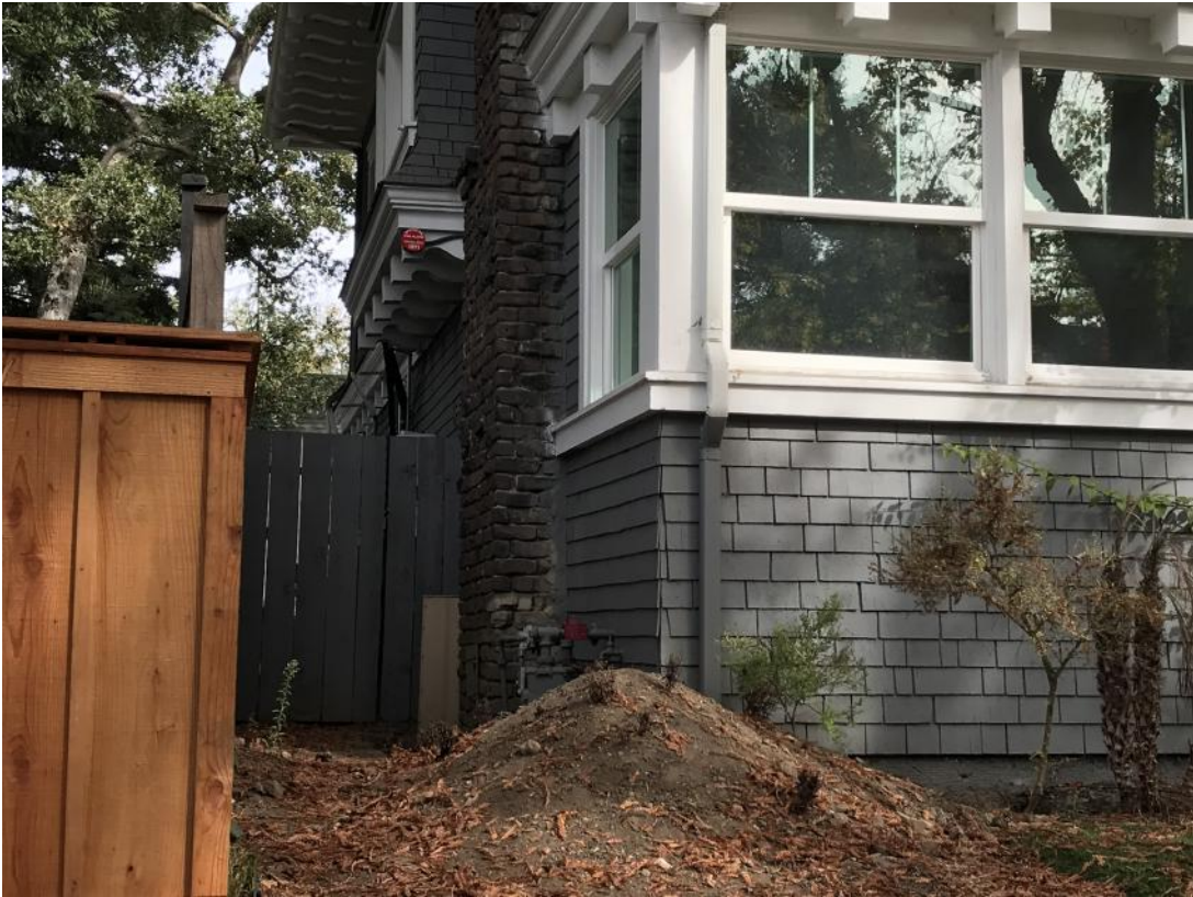
View along rear facade from southwest corner of house, looking north.
