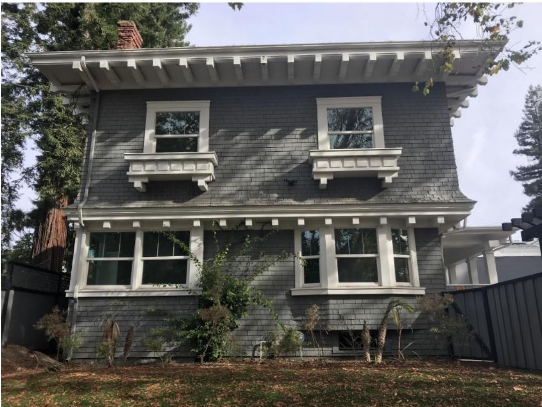
View of south facade from Woolsey Street, looking north.
