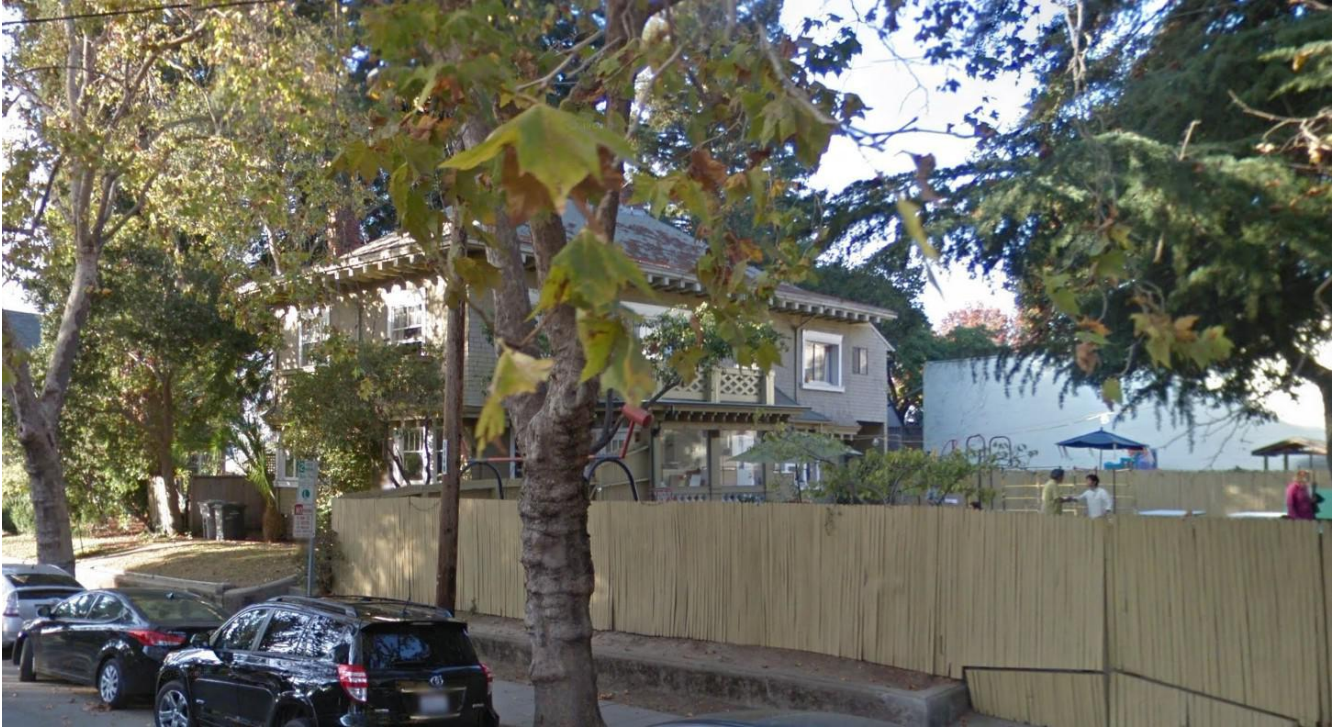
2845 Woolsey St. south and east facades, looking northwest from Woolsey St., ca. 2014. Note original balcony opening (glazed) and later northern addition at right side of second story. (Google Streetview)
