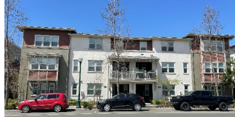
Decorative eave detailing, window lintels, and railings.
