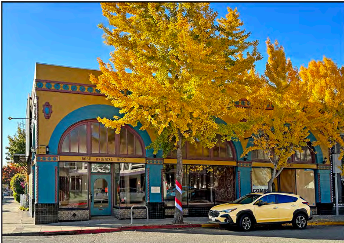
The Wilson-Tulanian Building, 2992 College Avenue. Anthony Bruce, 2025.
