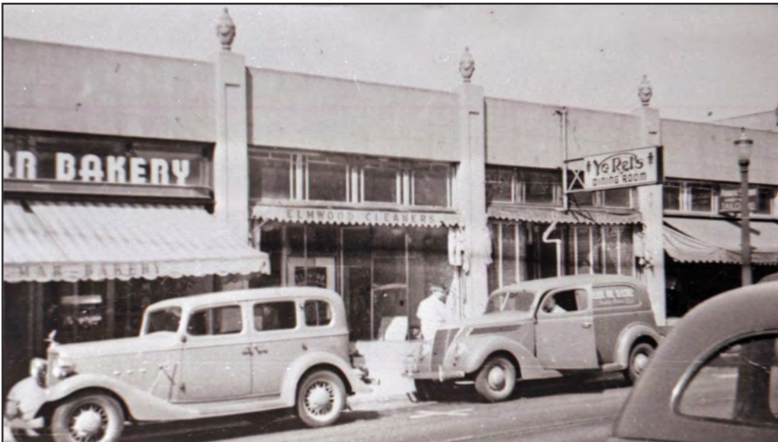
The Bischoff Shop Building No. 3. Shops in 1939: August Schaidt Tailor; Yo-Rel's Dining Room; Elmwood Cleaners; Wil-Mar Bakery. Ormsby Donogh, 1939, Donogh Real Estate File, BAHA.
