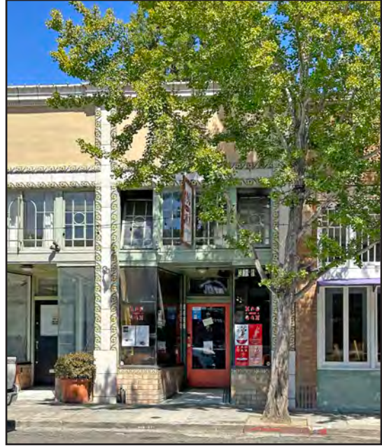
Morris Building, southernmost shopfront. Anthony Bruce, 2025.
