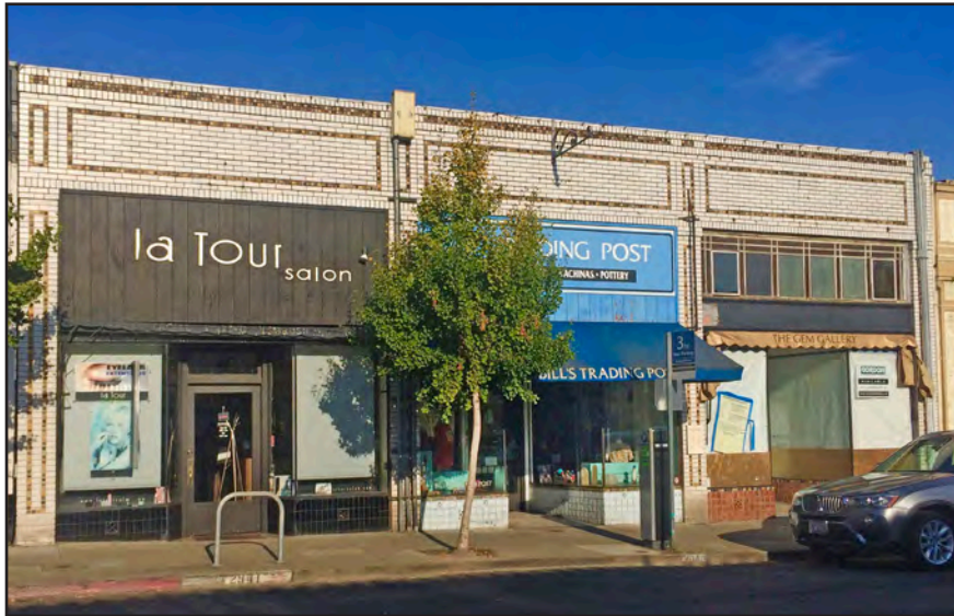
The Cianciarulo Building. Anthony Bruce, 2020.
