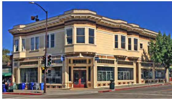
Figure 18: 2956 College Avenue – Present-day
