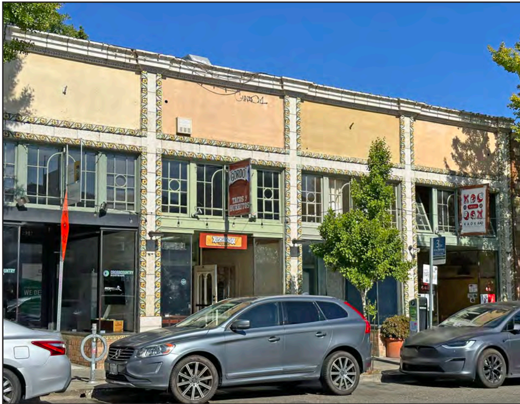
Morris Building, 2985–93 College Avenue. Note the plain stucco panels, once filled with floral relief work. Anthony Bruce, 2025.
