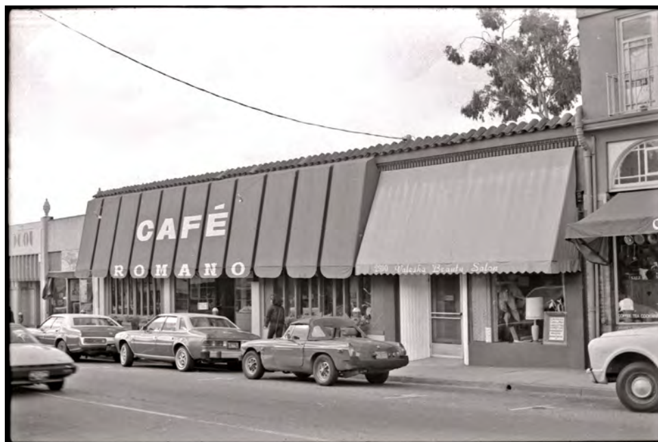
The Bischoff Shop Building, No. 2. Anthony Bruce, 1982.
