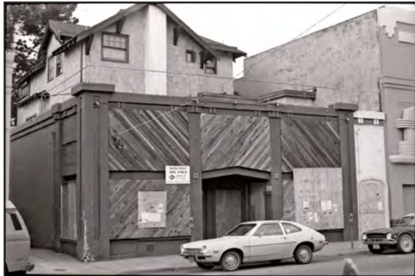
The vacant Nevin House and Nevin shopfronts after the Berkeley Repertory Theater had moved out. Anthony Bruce, 1982.
