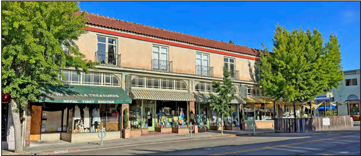
The Bischoff Building, view looking northwest. Anthony Bruce, 2025.
