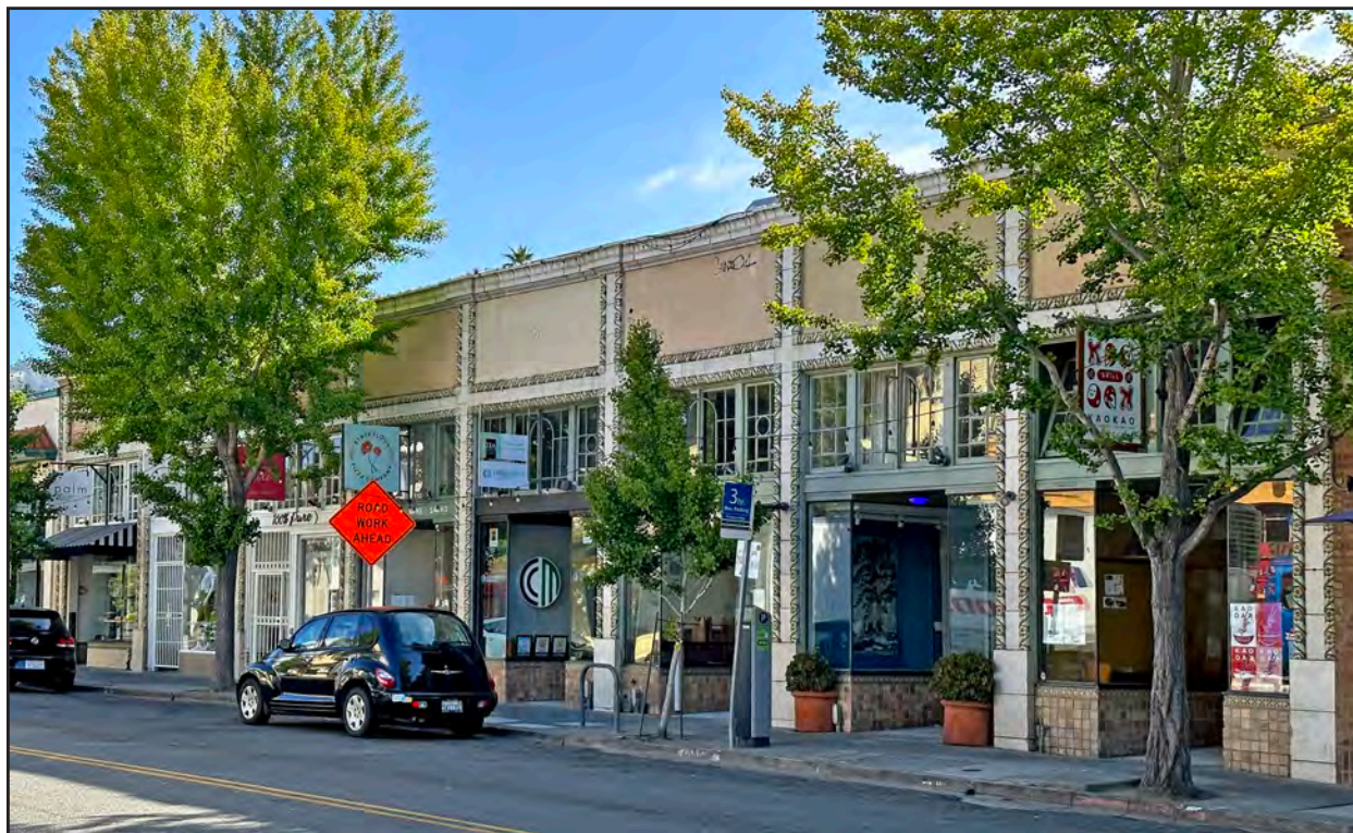
The Morris Building, 2993 College Avenue. Anthony Bruce, 2025.
