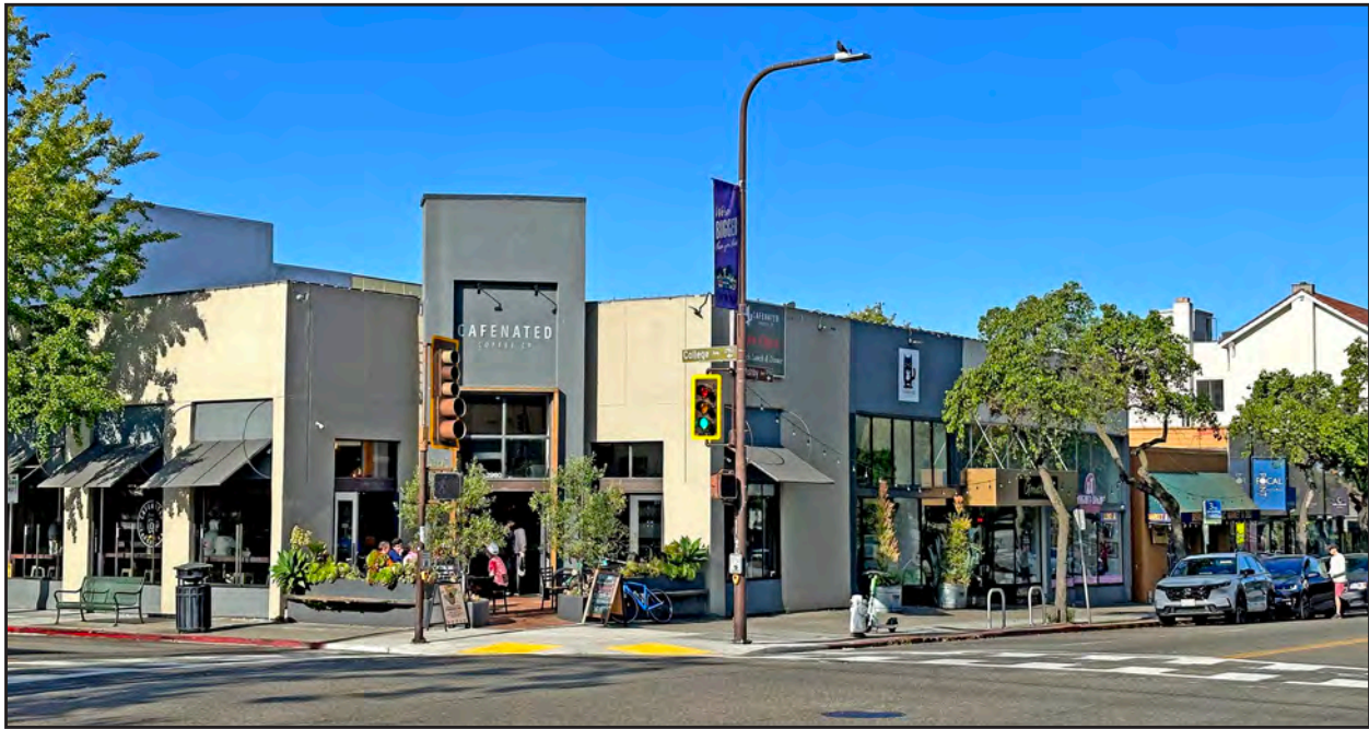
The Scott Building, 2960 College Avenue. Anthony Bruce, 2025.
