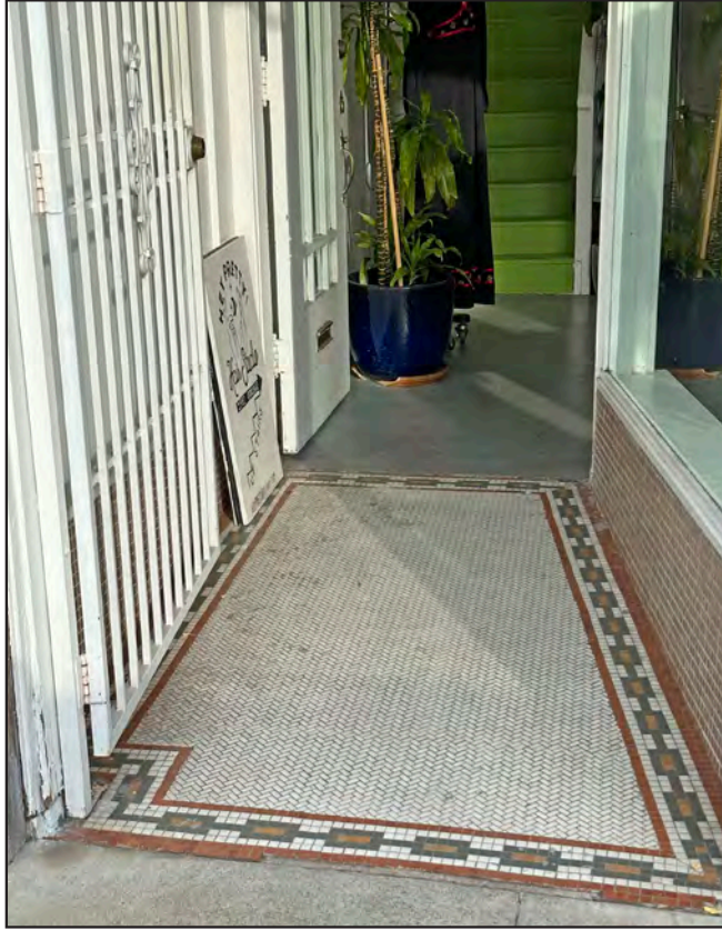
Mosaic tile entry paving at 2979 College Avenue in the Sager Building. It dates from a 1930 alteration to the shopfront. Anthony Bruce, 2025.
