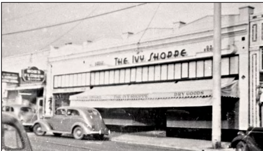
The Curry Building with the decorative parapet still intact. Ormsby Donogh, 1939, Donogh Real Estate File, BAHA.
