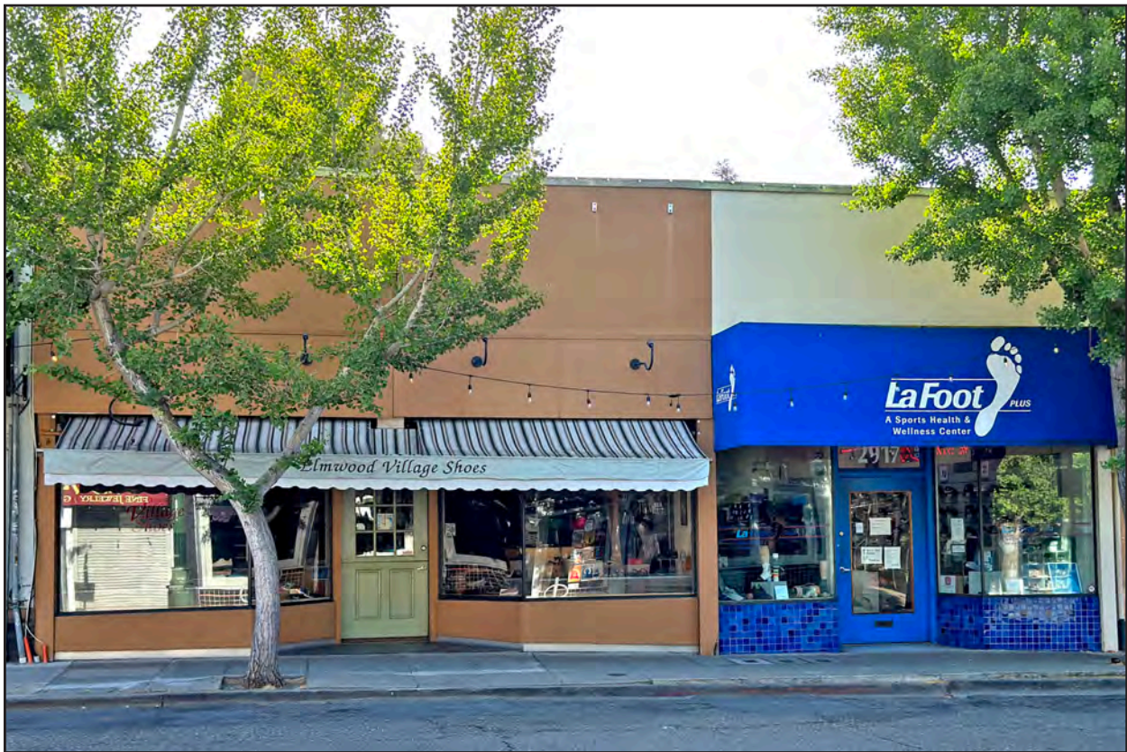
The McCullough Building, 2917 College Avenue. Anthony Bruce, 2025.
