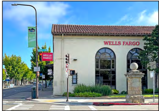
Mercantile Trust Company, side view from Ashby Avenue. Anthony Bruce, 2025.
