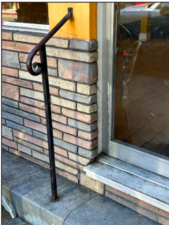
Simulated ledge rock bulkhead at the Conwell Building, 2942 College Avenue. Anthony Bruce, 2025.
