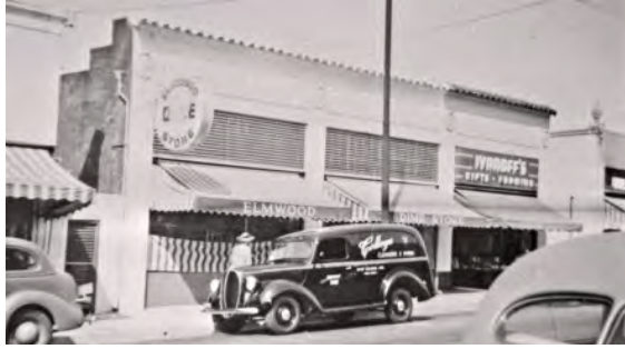
Figure 13: 2936-2940 College Avenue – 1936 - Twentieth Century Commercial Building with Mediterranean Revival Elements
