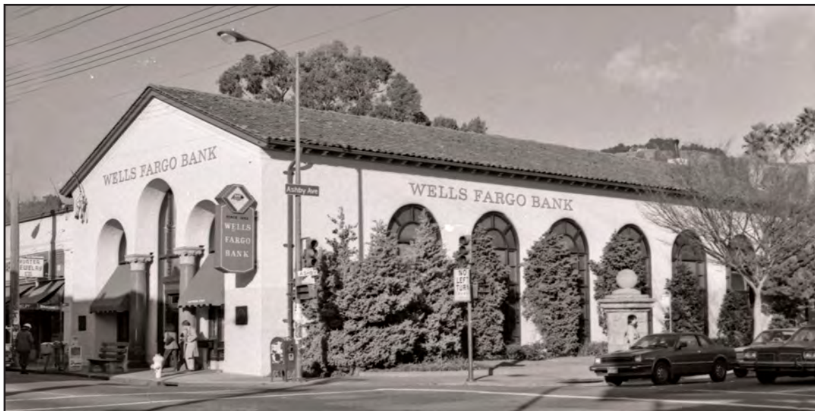
Mercantile Trust Company, showing both College Avenue and Ashby Avenue frontages. Anthony Bruce, 1982.
