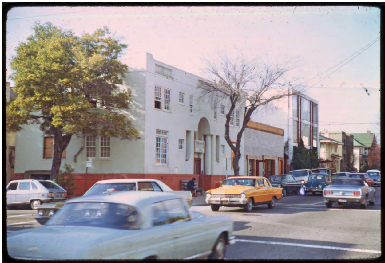
The Bischoff apartment house undergoing remodeling, 1973. BAHA archives.
