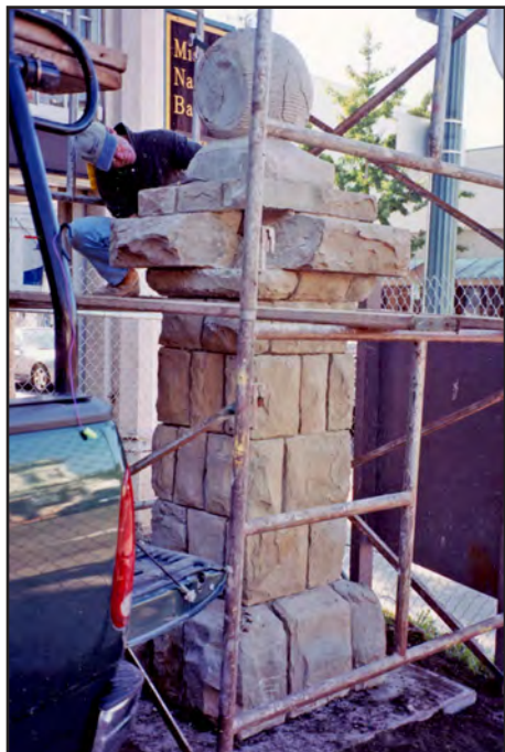
above and below: North and south pillars undergoing restoration.
