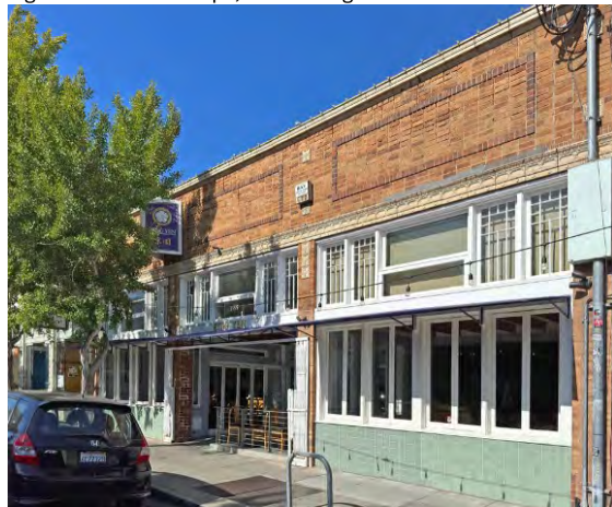
Figure 8: Midgley-Jennings Building, 2997 College Avenue
