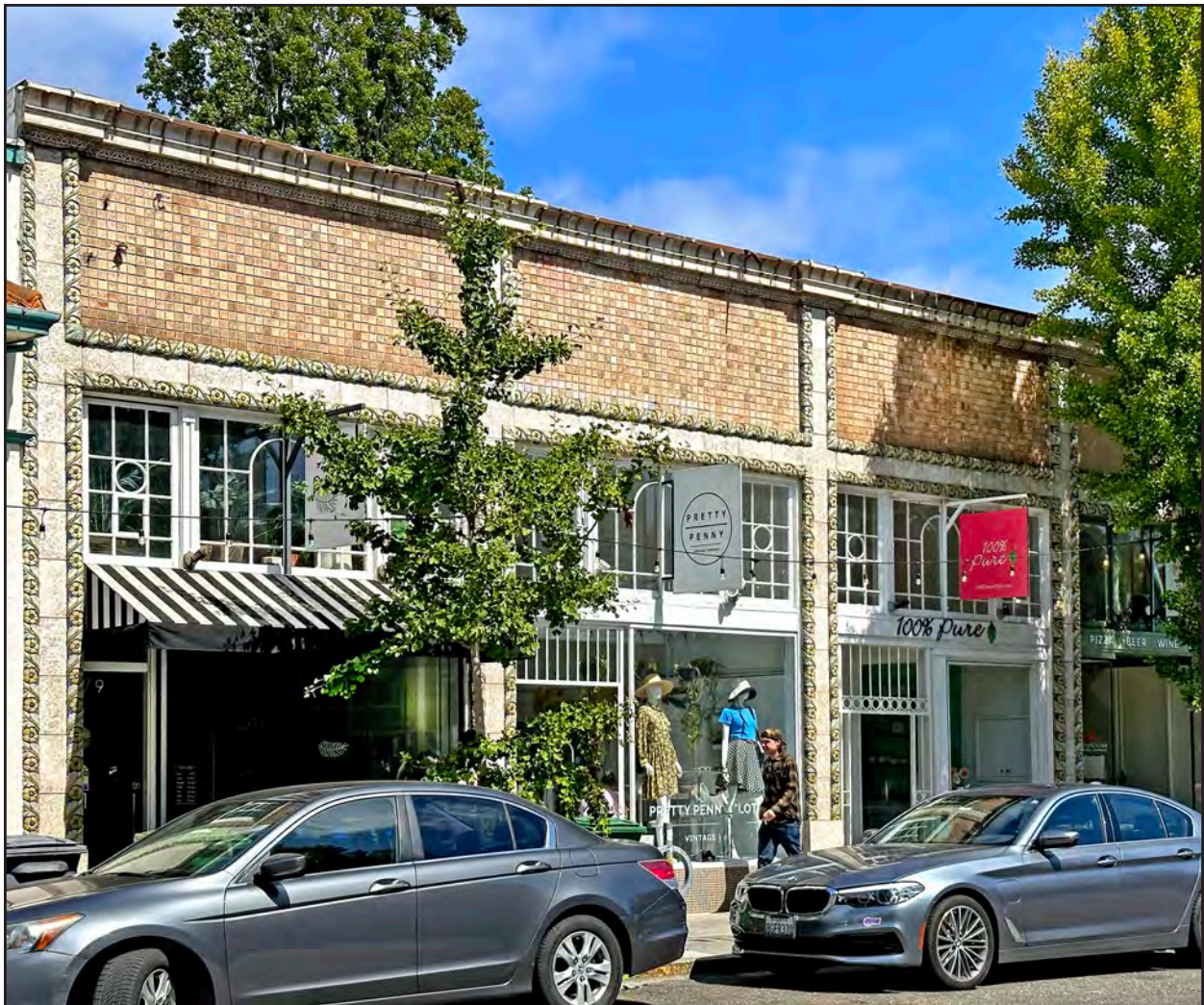
The Sager Building at 2979 College Avenue. Anthony Bruce, 2025.
