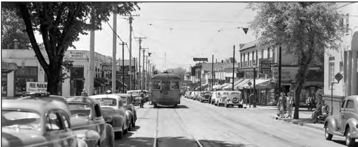
Looking south on College from the Safeway store in 1944. Many retractable awnings and telephone poles—and even a streetcar—are visible. Found on-line.
