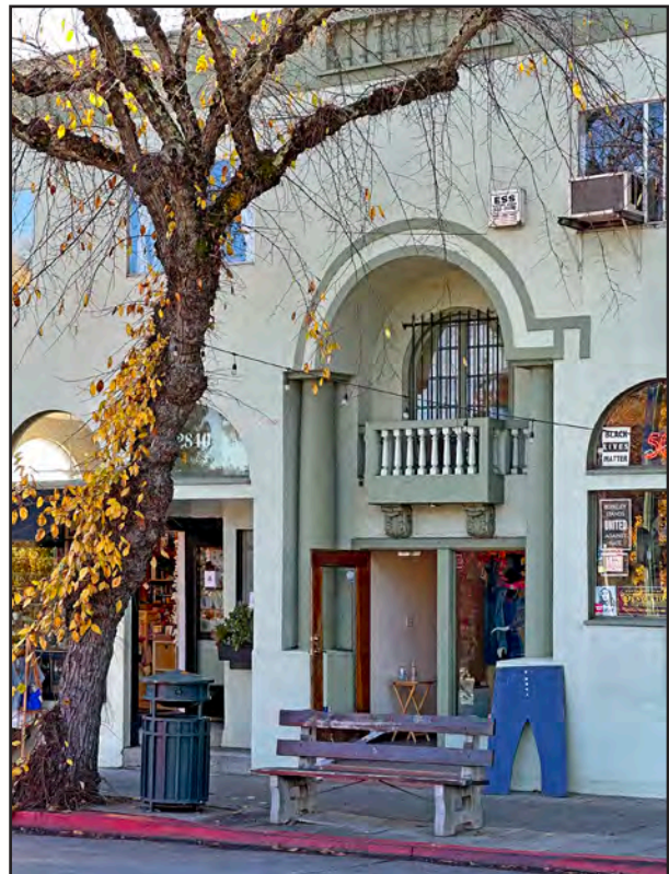
The Bischoff apartment house, entrance. Anthony Bruce, 2025.
