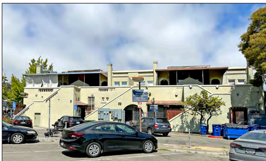
Bischoff Building, rear, viewed from parking lot. There are four arched entrances to apartments on the second floor. Anthony Bruce, 2025.
