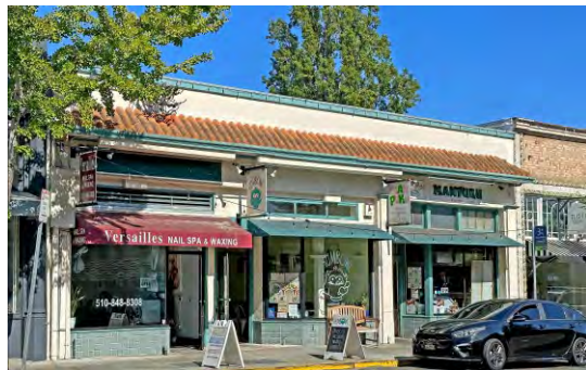
Figure 20: 2973 College Avenue – Present-day
