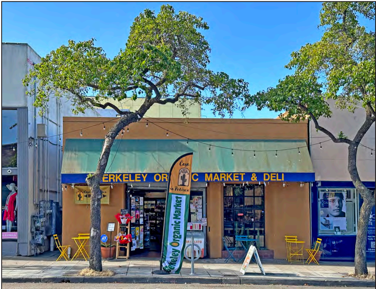
The Gallardo Building, 2642 Ashby Avenue. Anthony Bruce, 2025.
