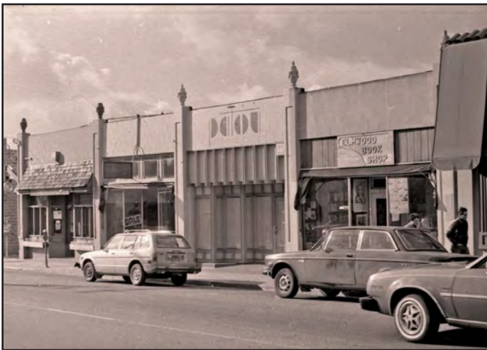
The Bischoff Shop Building No. 3. Anthony Bruce, 2025.
