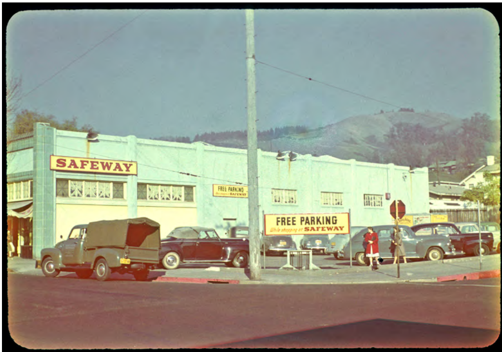
The Safeway Building, showing the value of the parking lot's "open space" to give a clear view of Dwight Way Hill from the Elmwood commercial district. Byron Bolfig, November 1947, Berkeley Historical Society.
