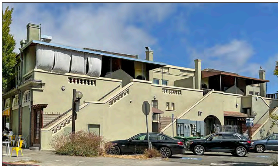
Bischoff Building, rear, viewed from Russell Street, showing grand balustraded stairway and two secondary stairs. Anthony Bruce, 2025.
