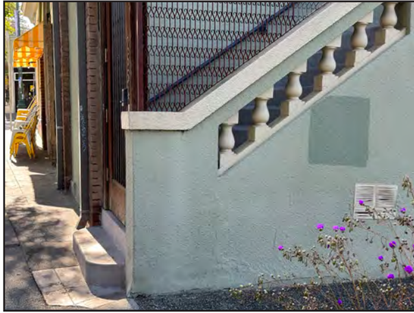
Bischoff Building, grand stairway to apartment level on Russell Street. Anthony Bruce, 2025.
