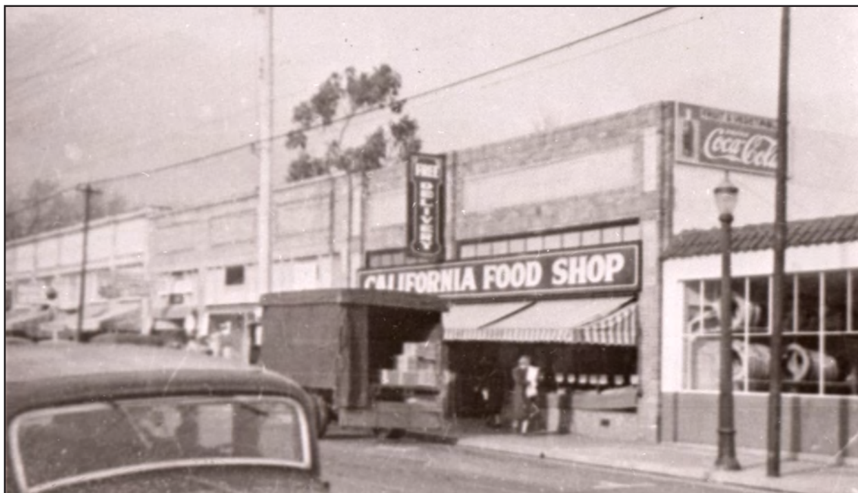
The Midgley Building, showing the original brick façade. Ormsby Donogh, 1939, Donogh Real Estate File, BAHABA/
