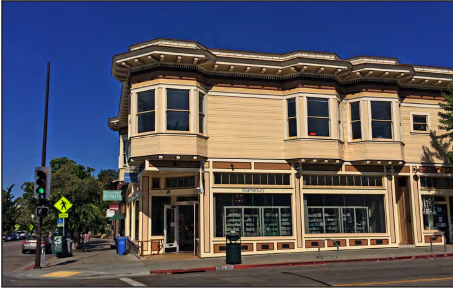
Koerber Building, 2956 College Avenue; College Avenue frontage. Anthony Bruce, 2020.
