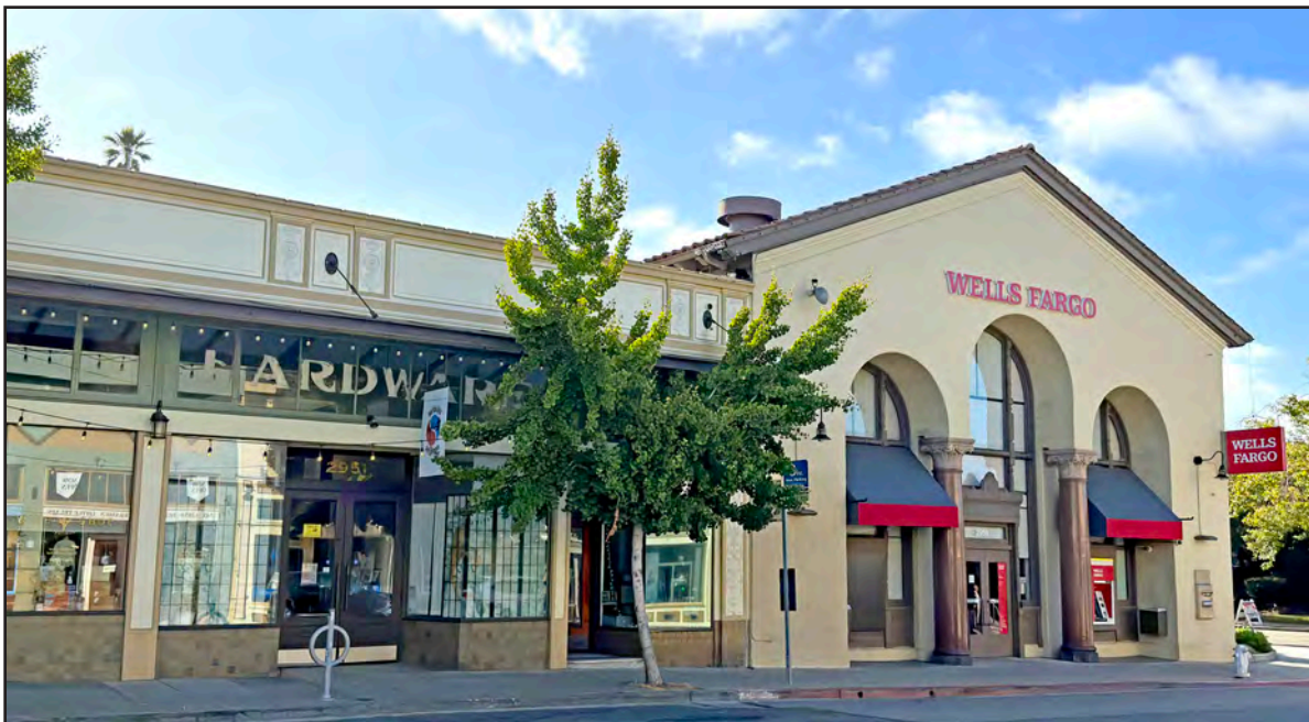
Mercantile Trust Company. in its setting on College Avenue. Anthony Bruce, 2025.
