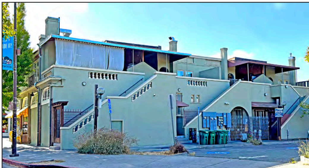
Bischoff Building, rear, viewed from Russell Street, showing stairways. Anthony Bruce, 2025.
