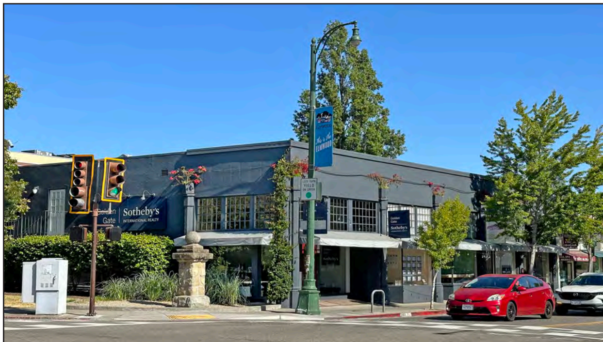
The Romie Building, 2961 College Avenue. Anthony Bruce, 2025.
