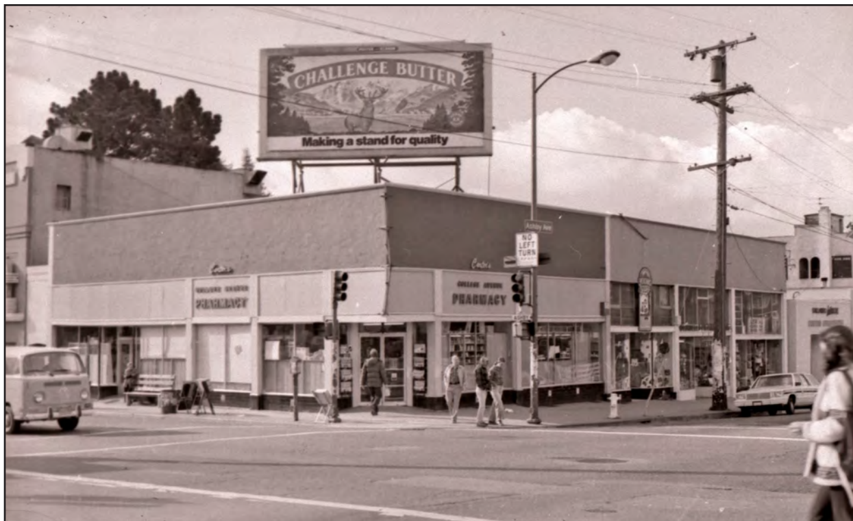
The Scott Building, showing the mass of the 1910 structure intact before the 1988 fire. Anthony Bruce, 1982,
