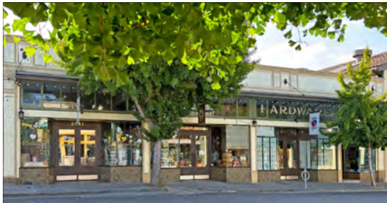
Figure 9: Stover Building, 2947 College Avenue
