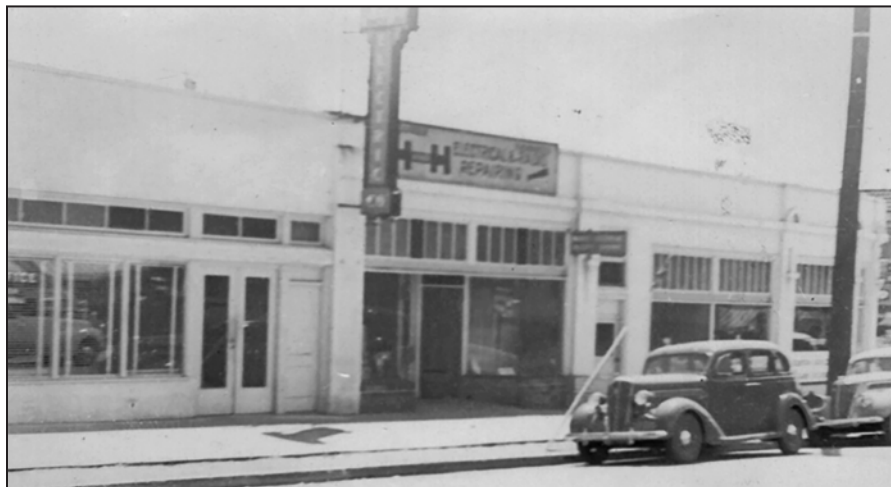
Dondero Building, Russell Street frontage, showing the now-missing center shopfront. Ormsby Donogh, 1939, Donogh Real Estate File, BAHA..
