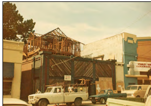
Construction, or deconstruction, beginning. Betty Marvin, 1982.
