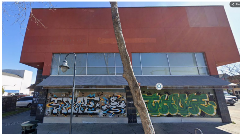
Image 2: San Pablo Avenue Side Facade (West)
