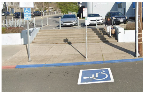
Before: On-street accessible parking with blocked sidewalk access, creating barriers for wheelchair users and pedestrians.
