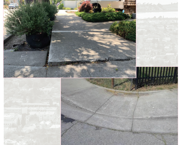
Above Images: Examples of changes in level (elevations) on sidewalks that require improvements
