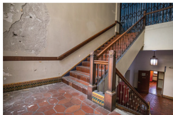
Repair and Improvements to Veterans Building
