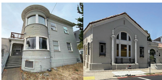
Before: Aging, inaccessible facility with limited capacity
