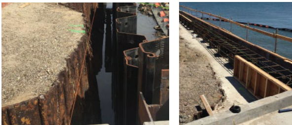
After: New, resilient seawall with sheet pile wall and enforcement structures
