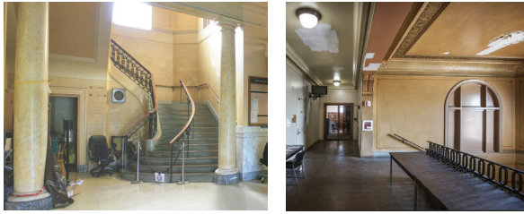
Before: Seismically vulnerable historic Old City Hall
