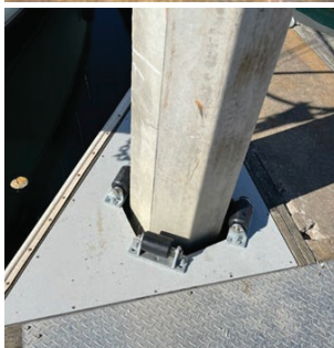
After: New long-life concrete piles
