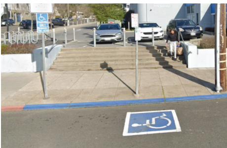
Before: On-street accessible parking with blocked sidewalk access, creating barriers for wheelchair users and pedestrians.
