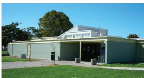
Before: Aging Facility, Current State of Frances Albrier Community Center (FACC)
