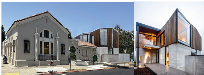
After: Safer, new clinic with expanded treatment and group space (concept rendering)
