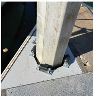
After: New long-life concrete piles
