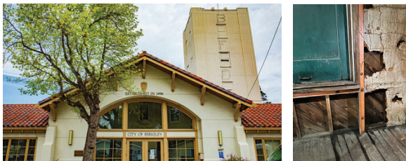
Before: Constrained, outdated training site, including water damage (right image)
