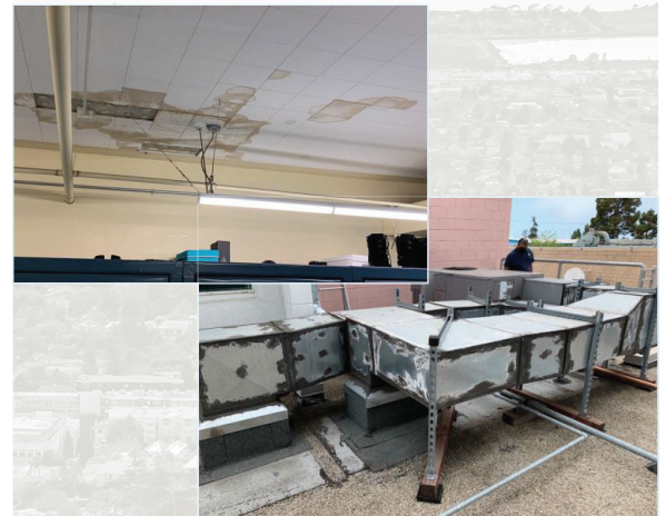
Above Images: Water damage from roof leaks at PSB (top left) and failing HVAC at Fire Station 5 (bottom right).
