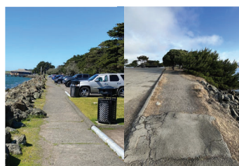
Repair and Improvements to Berkeley Waterfront Bay Trail
