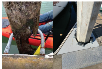
Repair and Improvements to Marina Docks Timber
