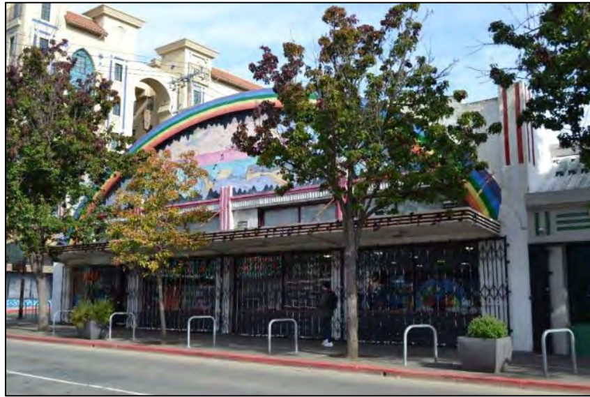
Figure 3. Primary (west) façade of 2455 Telegraph Avenue, viewed facing northeast Source: ARG, November 2024
