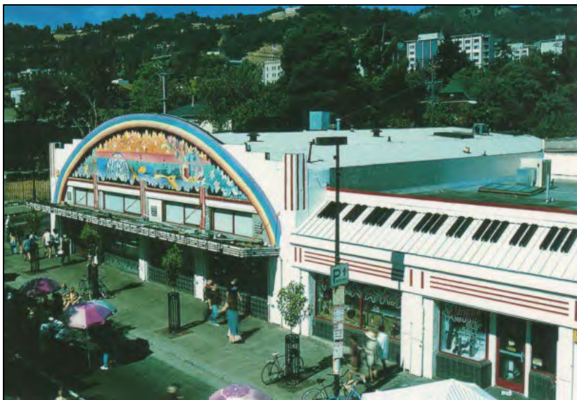
Figure 38. 2455 Telegraph Avenue (left) and 2465 Telegraph Avenue (right), photographed in the 1990s Source: Berkeley Public Library
