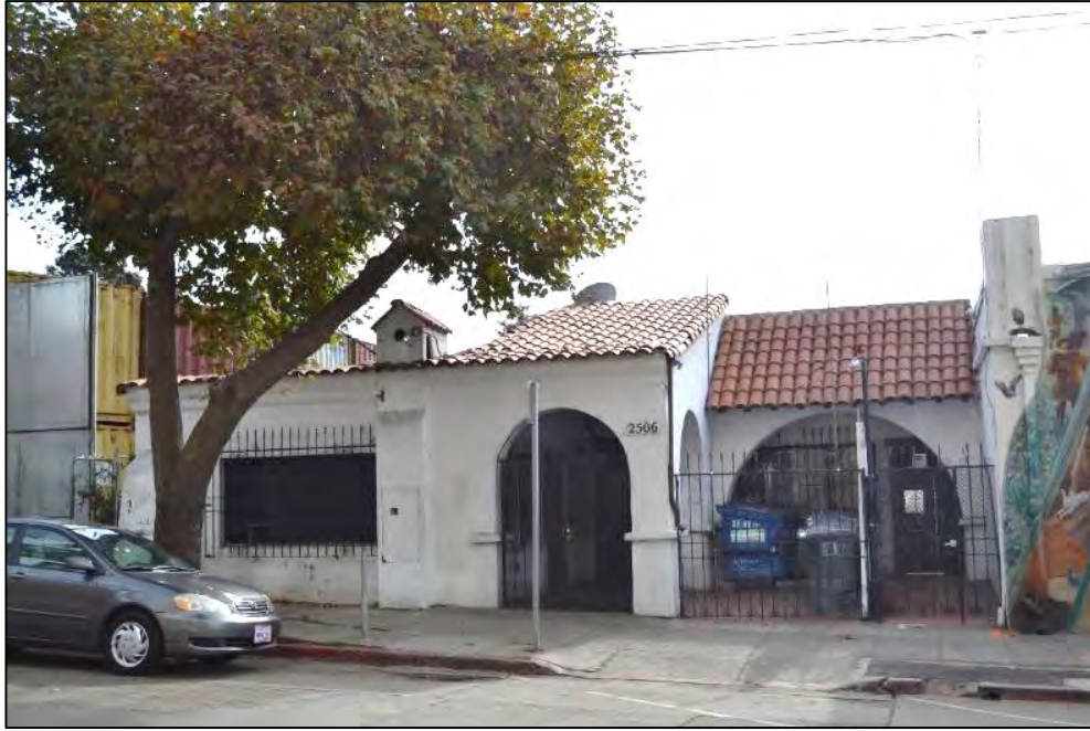
Primary (north) façade of 2506 Haste Street, viewed facing south
