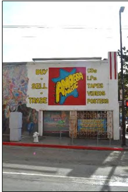
West end of north façade, featuring a mural advertising Amoeba Music, viewed facing south
