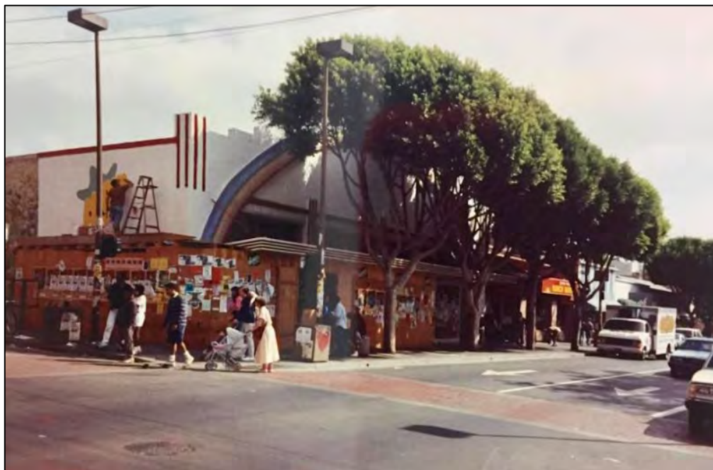
The building at 2455 Telegraph Avenue amidst improvements for Amoebe Music, September 1990
