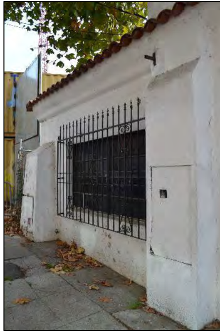
Window and security grate at the north façade of 2506 Haste Street, viewed facing southeast
