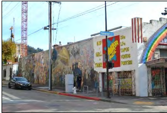
Figure 9. North façade viewed facing southeast from Haste Street
