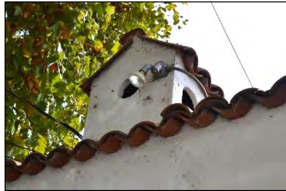
Figure 19. Spanish-inspired chimney cap along the front façade Source: ARG, November 2024
