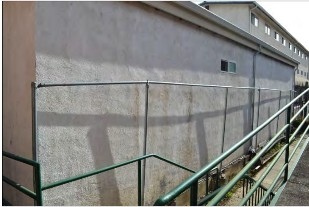
West wall of the south addition of 2506 Haste Street, viewed facing southeast from the rear pedestrian alley
