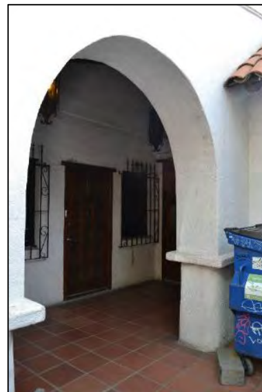
Figure 21. West-facing door and windows in the front vestibule Source: ARG, November 2024
