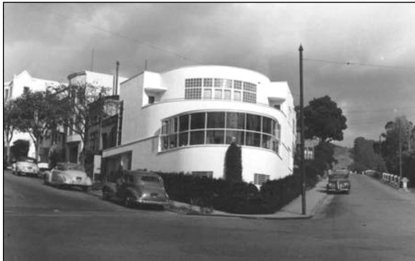
Figure 44. Streamline Modern residence located at the intersection of Hearst Avenue and LeConte in Berkeley, photographed c.1955 Source: Berkeley Public Library
