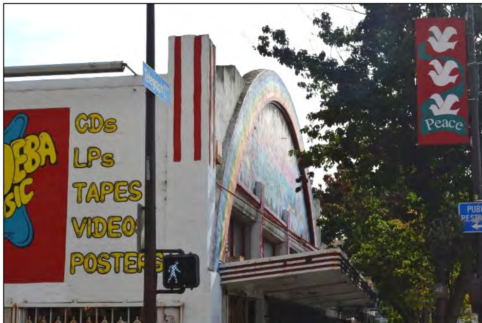
Northwest corner pier, arched frame, and marquee, viewed facing south from Haste Street
