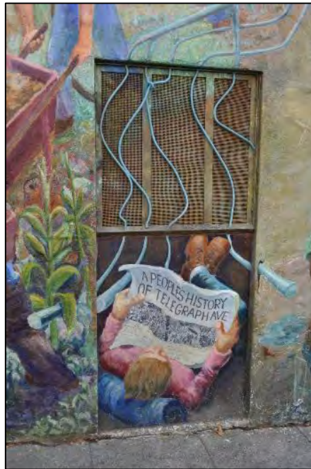
Door opening covered with an infill panel and metal screen, located at the center of the north façade
