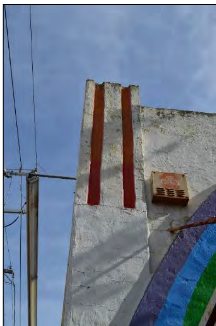
Detail of the fluted pier at the northwest corner of 2455 Telegraph Avenue
