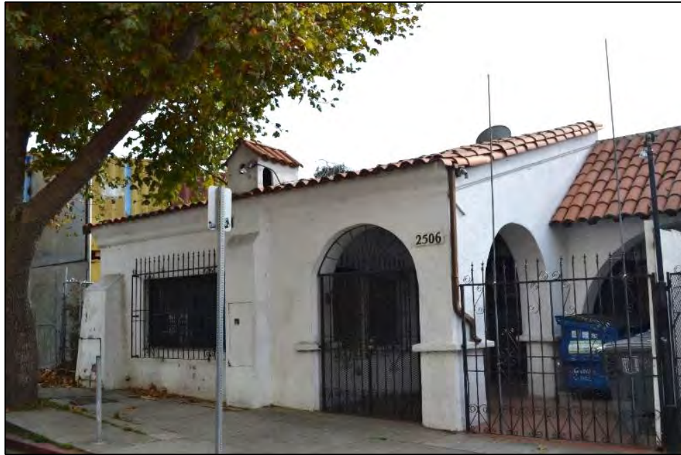
Projecting portion of 2506 Haste Street, viewed facing southeast
