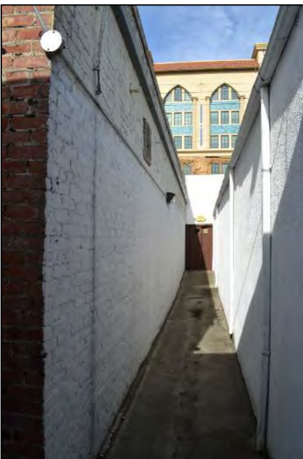
Rear pedestrian alley, viewed facing north; rear the rear (east) wall of 2455 Telegraph Avenue is at left, and the west wall of 2506 Haste Street is at right
