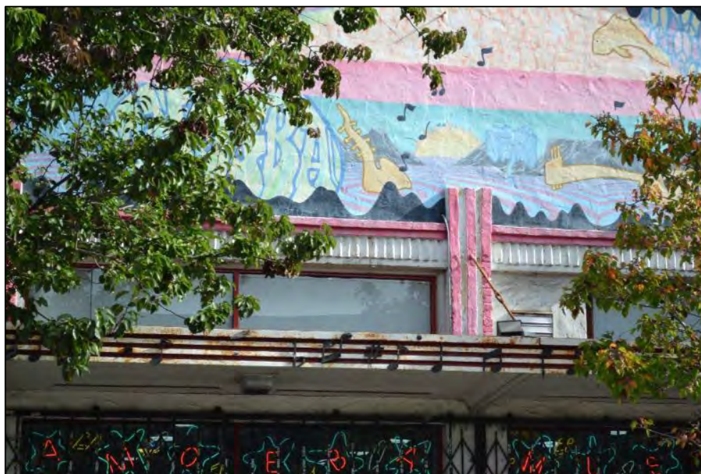
Detail of clerestory window band, chevron frieze, and fluted pilaster above the front marquee
