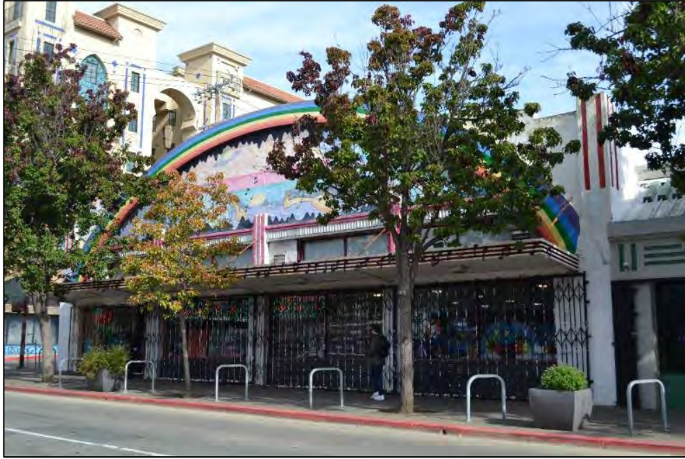
Primary façade of 2455 Telegraph Avenue, viewed facing northeast from Telegraph Avenue
