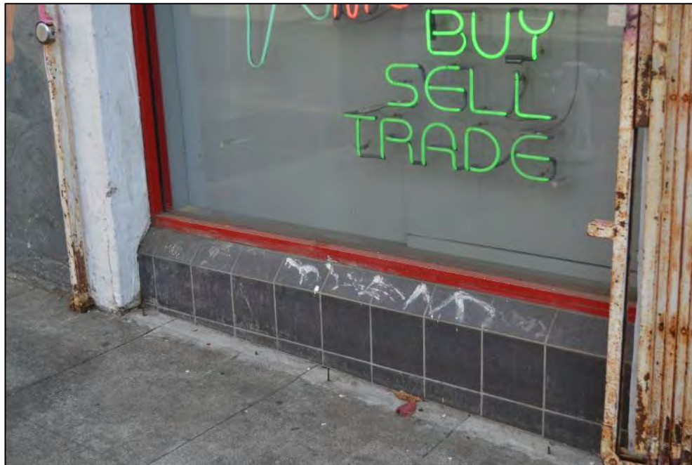
Detail of non-historic tiled bulkhead at the north façade
