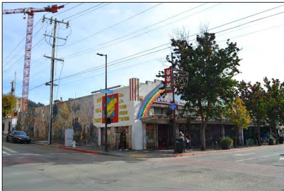
North façade (at left) and primary/west façade (at right), viewed facing southeast
