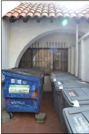
Figure 22. Arched opening recessed wall in the front service area Source: ARG, November 2024
