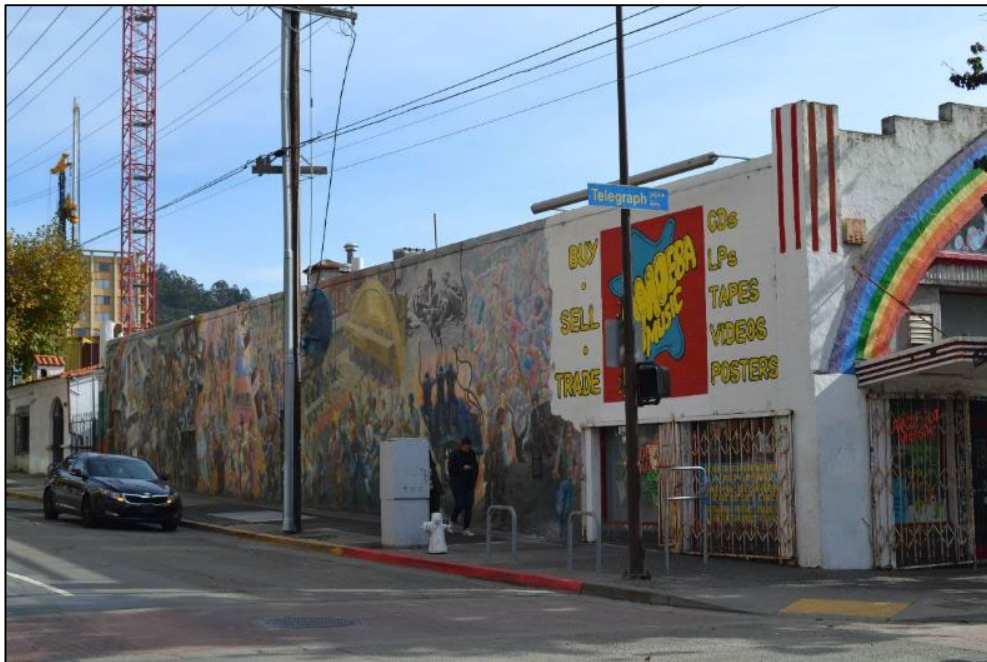
North façade along Haste Street, viewed facing southeast
