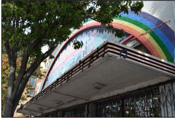
Figure 6. View of the grooved edges of the front marquee at the front façade Source: ARG, November 2024
