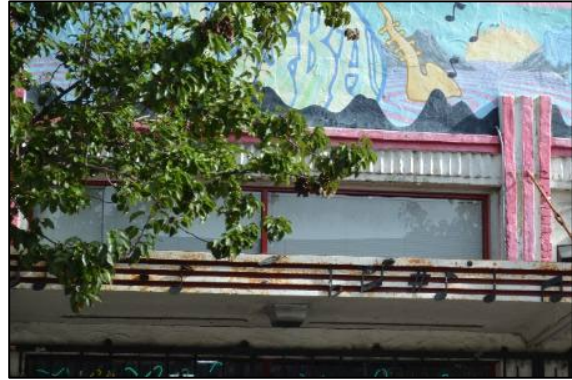
Figure 7. Detail view of clerestory windows and the molded stringcourse above the marquee Source: ARG, November 2024
