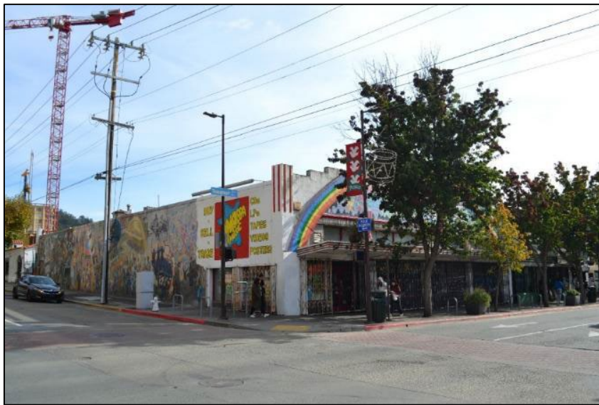
Figure 2. 2455 Telegraph Avenue, viewed facing southeast from the intersection of Telegraph Avenue and Haste Street
