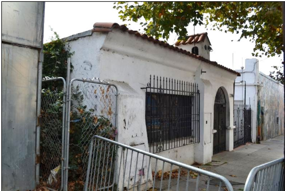
North façade of 2506 Haste Street, viewed facing southwest
