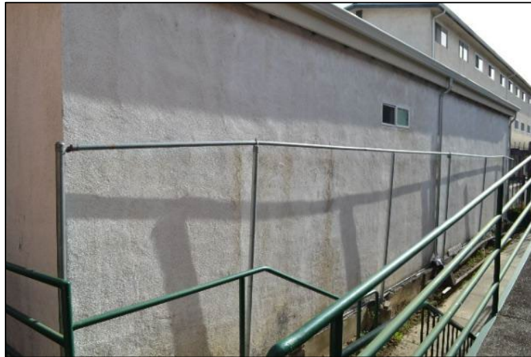
Figure 24. West wall of south addition, viewed facing southeast Source: ARG, November 2024
