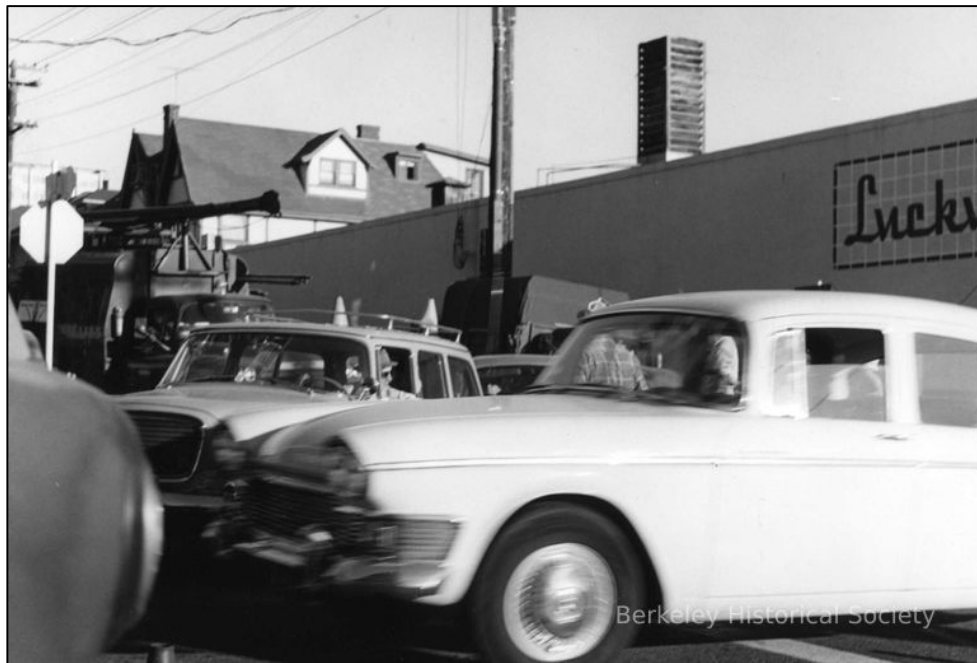
The north façade of 2455 Telegraph Avenue along Haste Street, photographed in the early 1960s Source: Berkeley Historical Society
