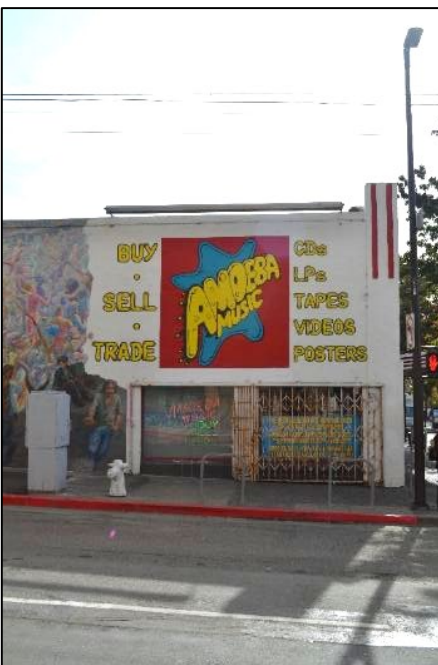
West end of north façade, featuring a mural advertising Amoeba Music, viewed facing south
