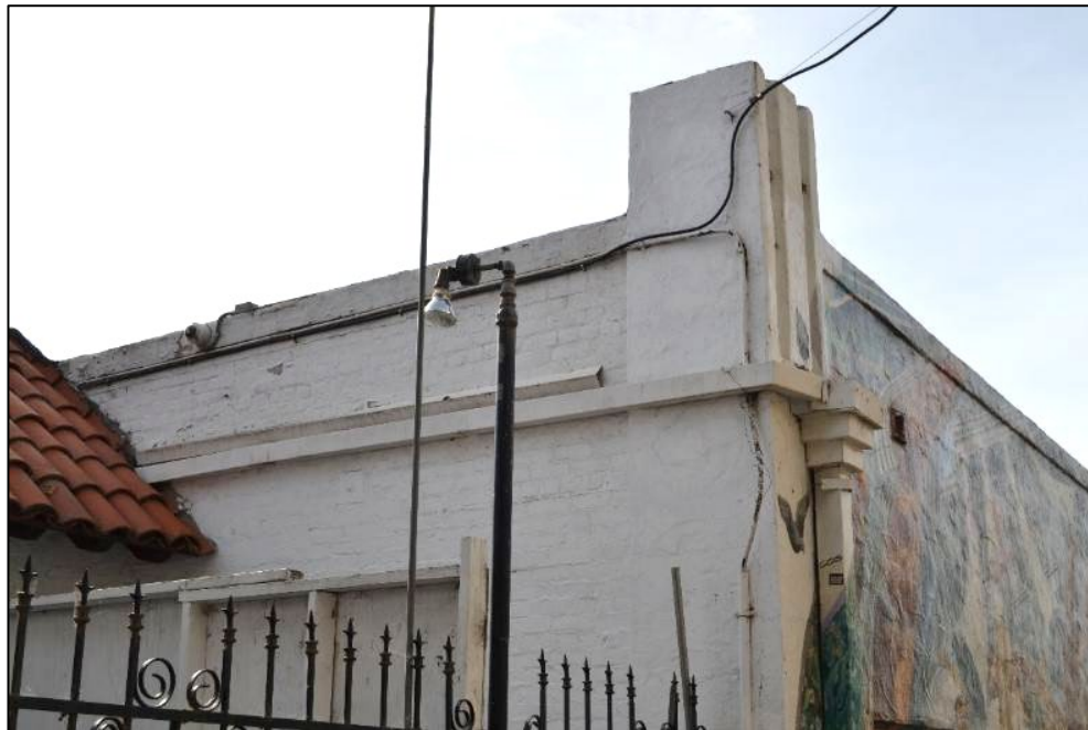
Northeast corner pier and exposed brick at the east façade of 2455 Telegraph Avenue
