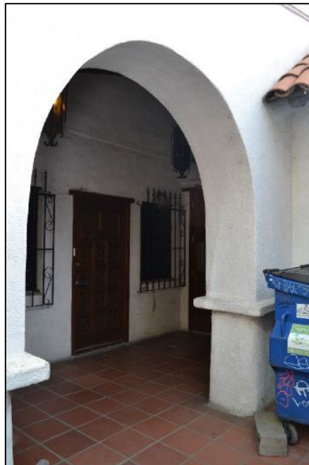
Door and windows within the vestibule at the center of 2506 Haste Street's north façade, viewed facing southeast
