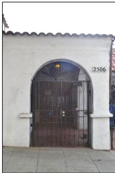
Figure 20. Arched opening at the center of the north façade Source: ARG, November 2024
