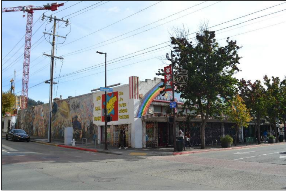
North façade (at left) and primary/west façade (at right), viewed facing southeast
