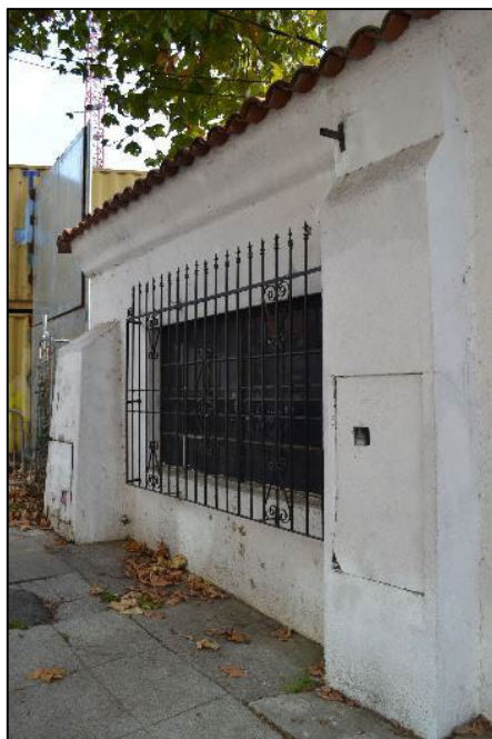
Window and security grate at the north façade of 2506 Haste Street, viewed facing southeast
