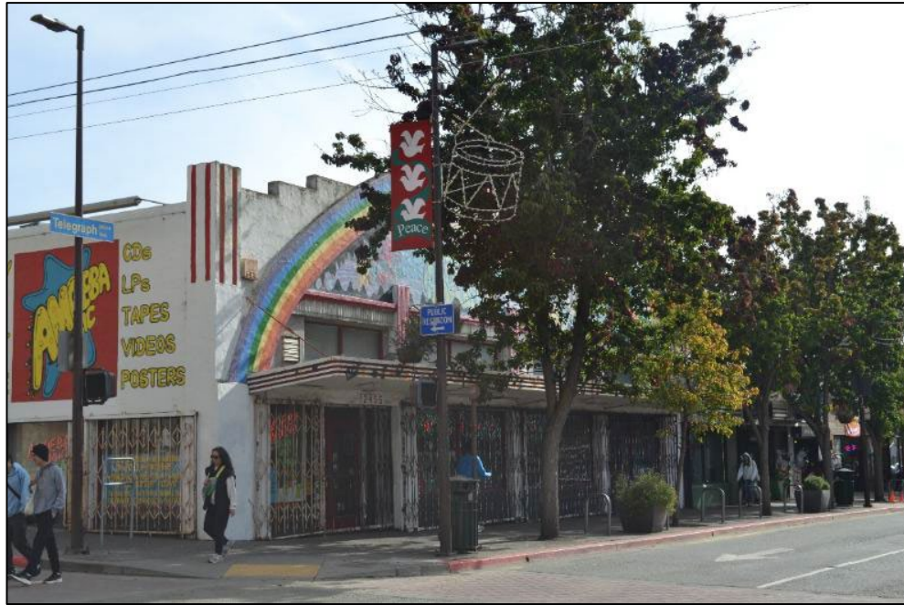
Primary façade, viewed facing southeast from the Telegraph-Haste intersection
