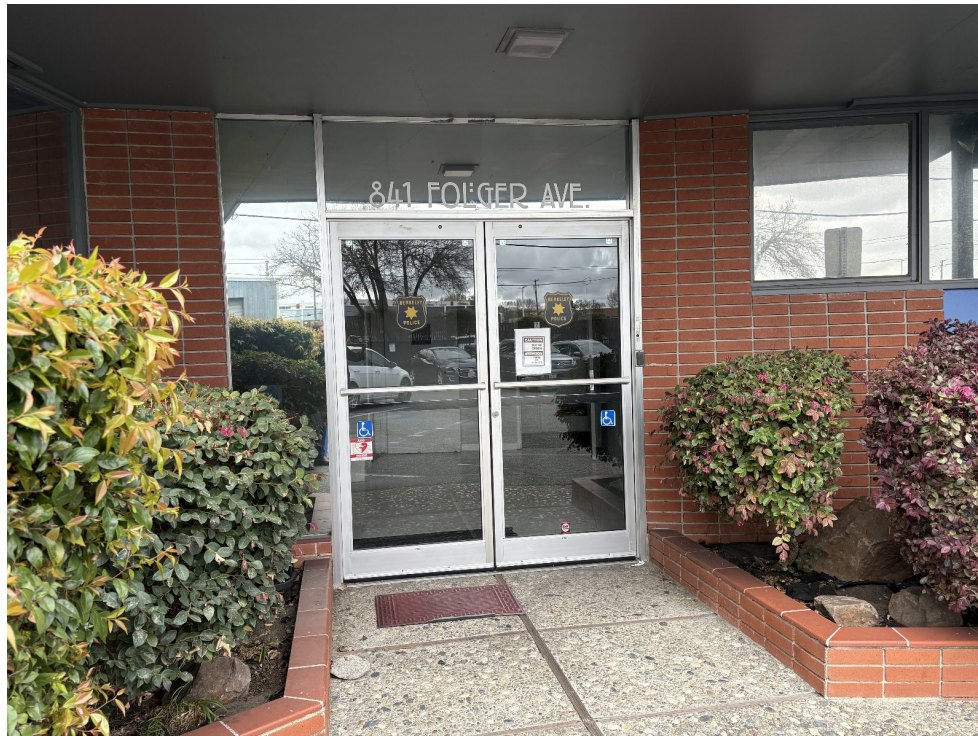
Lower primary (south) facade.
