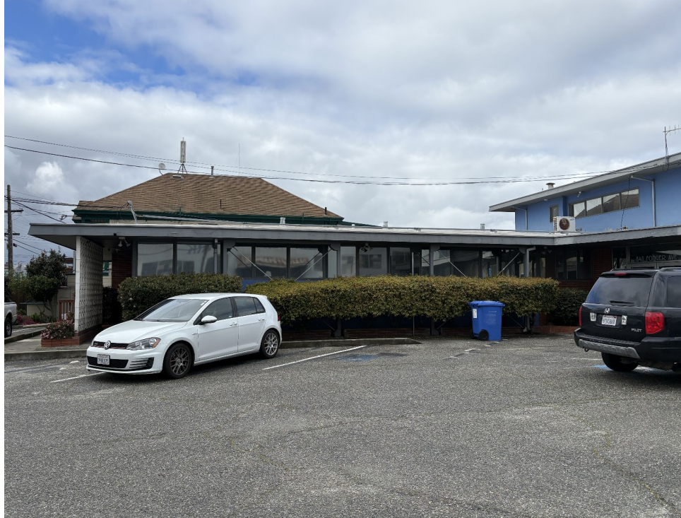
Primary (south) facade from Folger Avenue, looking north.
