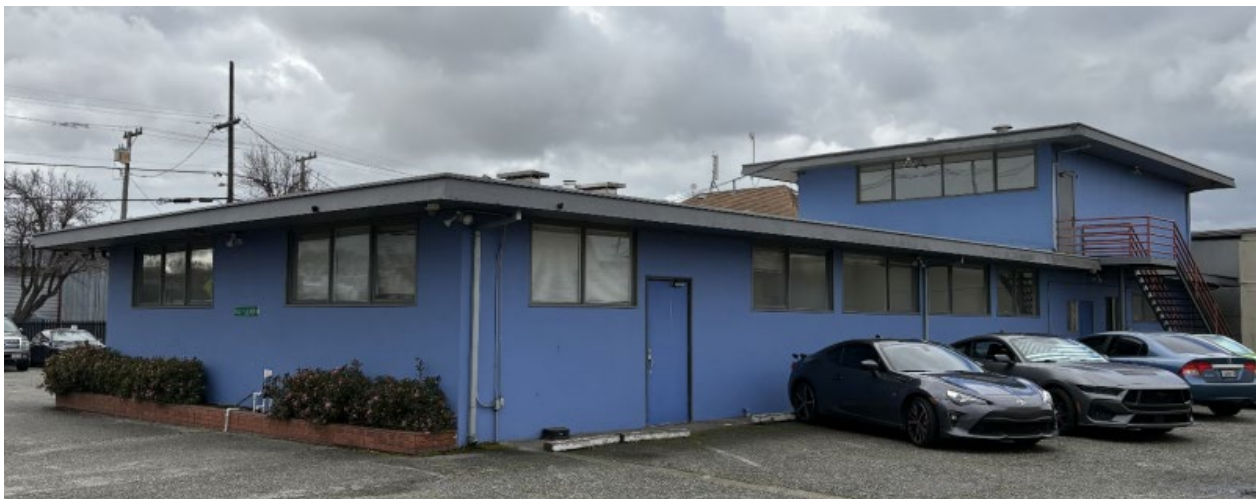
Figure 4: Rear Facade (North). Source: Historic Resource Evaluation
