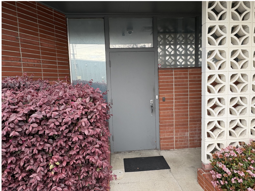
West facade, looking east.
