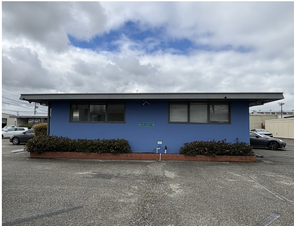
Detail of first story entry, right side of rear (north) facade.
