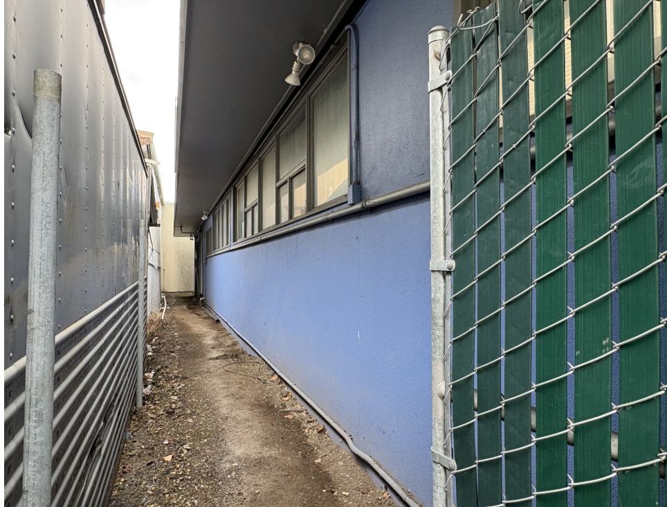
Rear (north) and west facades, looking southeast.
