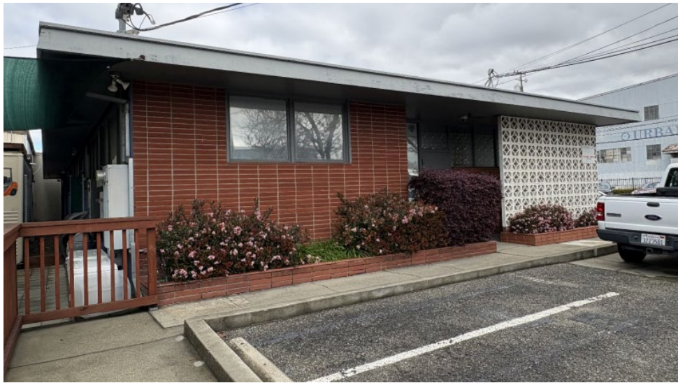
Figure 3: Second entrance along the south facade of the north-south wing. Source: Historic Resource Evaluation
