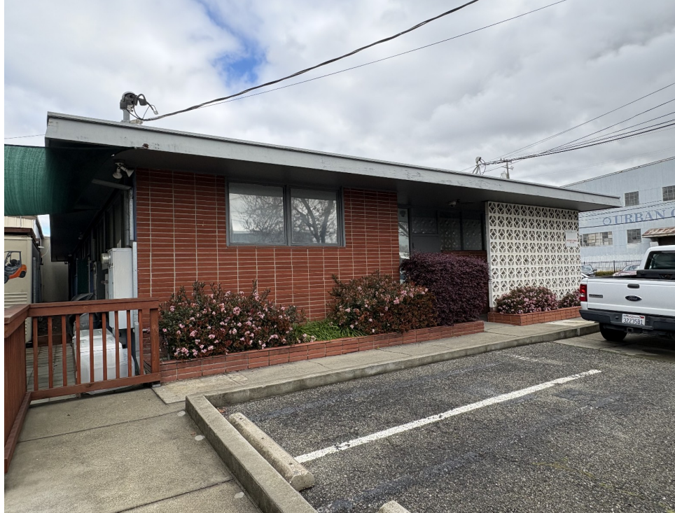
Upper primary (south) facade.
