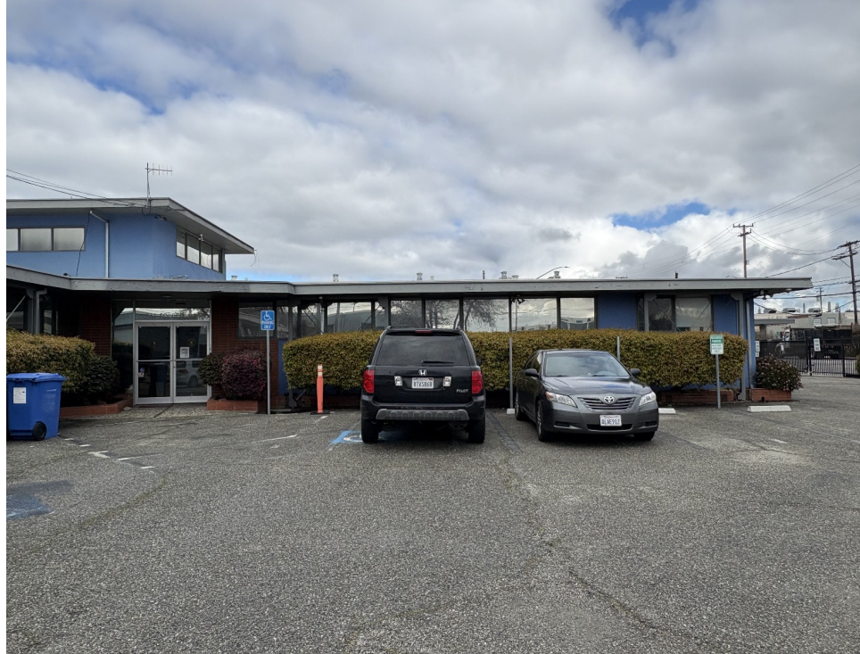
Concrete curb at front (south) of lot.
