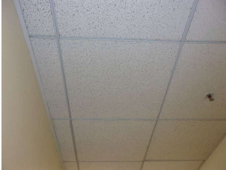
Photo 3 Second floor hallway: Ceiling tile.
