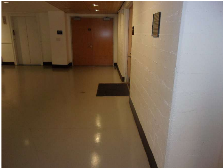
Photo 4 Basement hallway: Vinyl sheet flooring and baseboard mastic.
