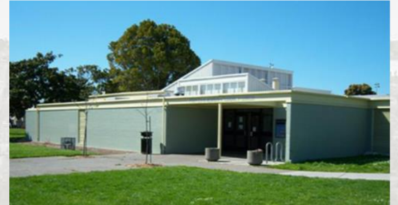
Before: Aging Facility, Current State of Frances Albrier Community Center
