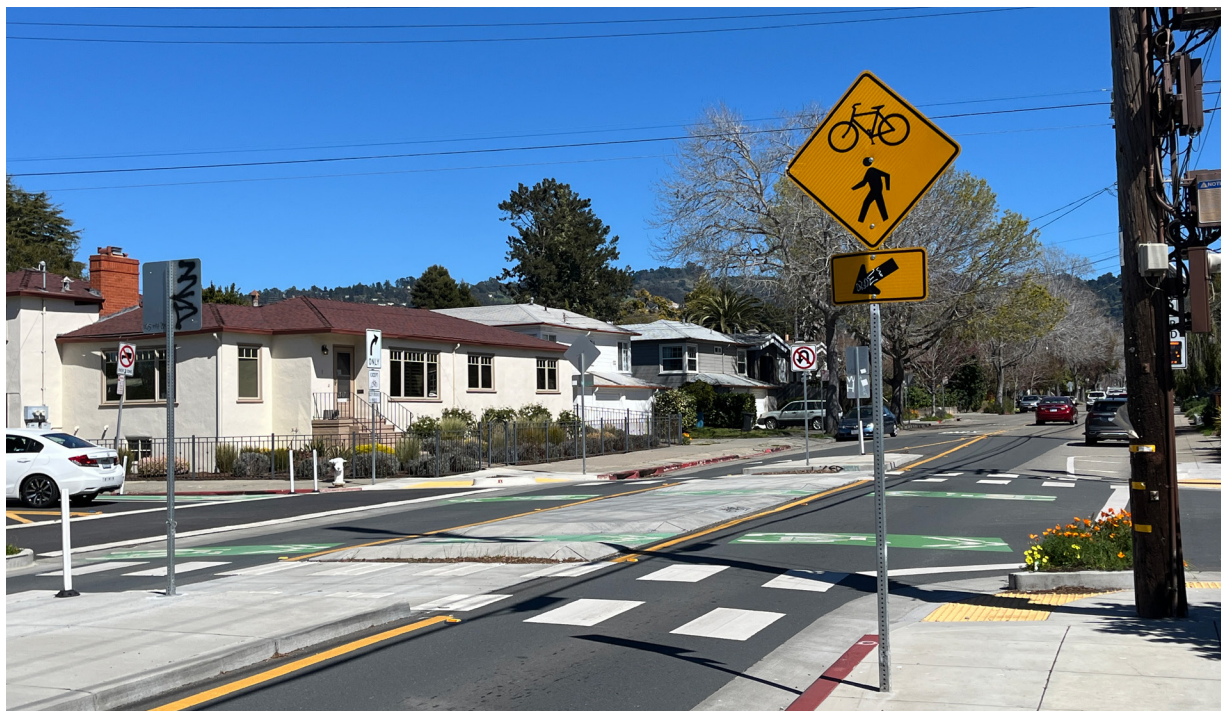
Median Islands at California Street and Dwight Way (Source: City of Berkeley)
