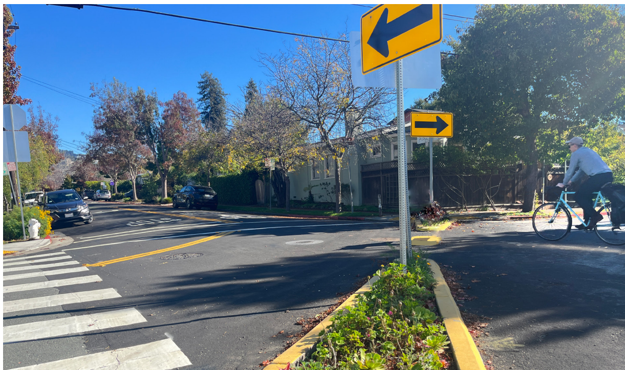
Newer Installation at Virginia and McGee (Source: City of Berkeley)
