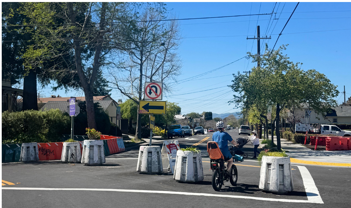
Older Installation at Virginia and Acton (Source: City of Berkeley)
