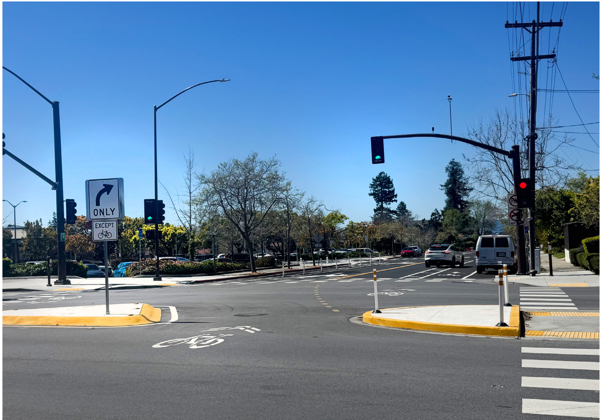
Traffic Signal with Diversion at Sacramento Street and Virginia Street (Source: City of Berkeley)
