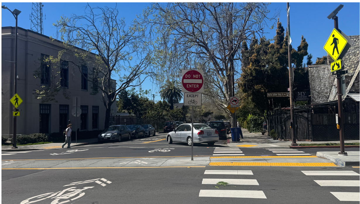
RRFB and a Median Island at MLK Jr. Way and Addison Street (Source: City of Berkeley)
