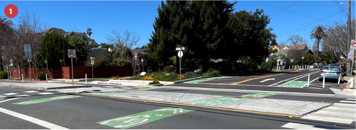
MEDIAN CROSSING on California Street at Dwight Way.
