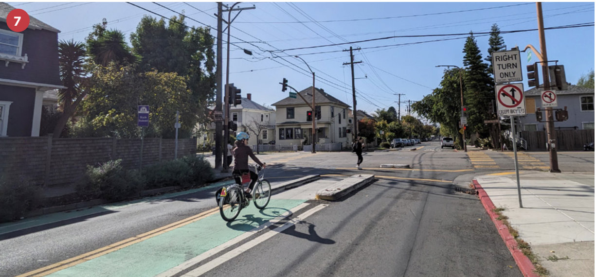
TRAFFIC SIGNAL CROSSING of MLK Jr. Way at Channing Way.
