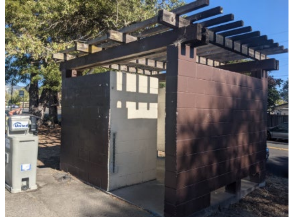
Park Restroom Replacement Project
