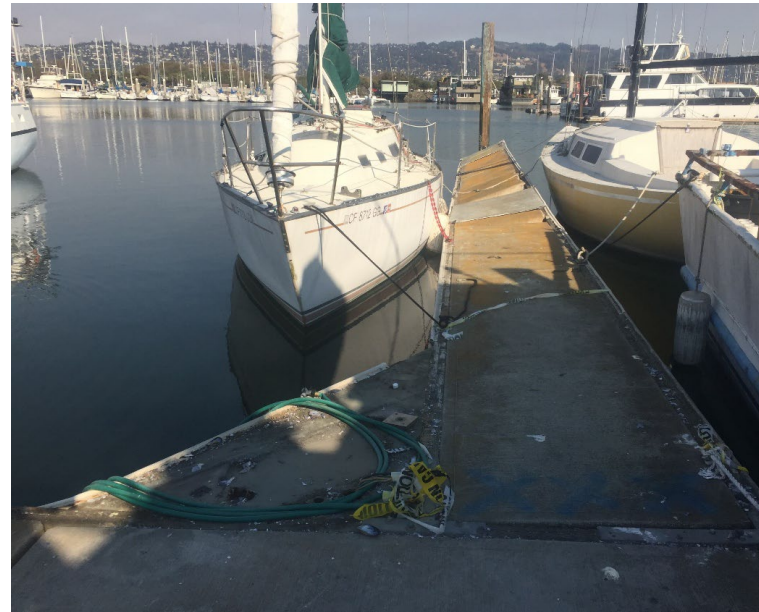
Finger Docks Replacement
