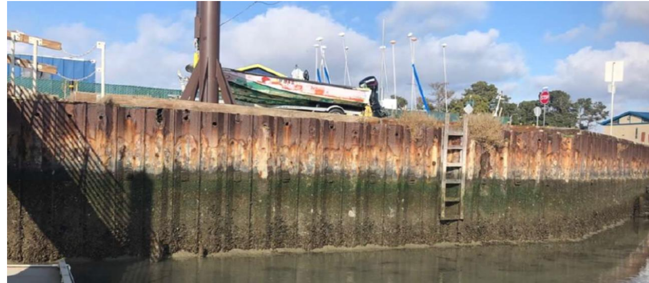
South Cove Seawall in Waterfront
