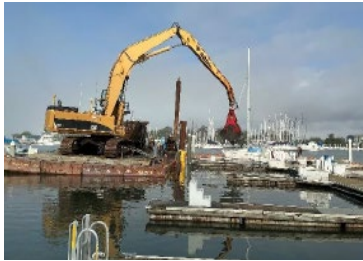
Marina Harbor Dredging
