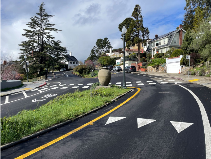
Street Rehabilitation and Surface Seals: Completion of the FY 2024 and FY 2025 Street Maintenance and Rehabilitation Projects at citywide locations identified in the 5 Year Paving Plan, totaling 30 lane miles of street paving and 14.5 lane miles of surface sealing.
