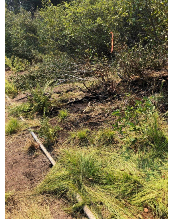
Echo Lake Water Intake Line
