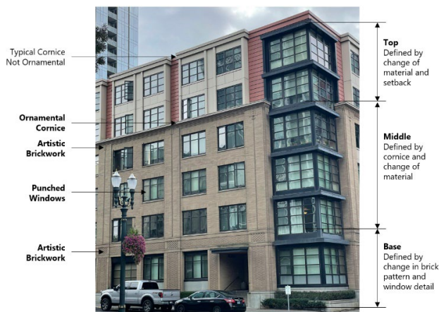
Figure 13. Example of Ornamental Façade
