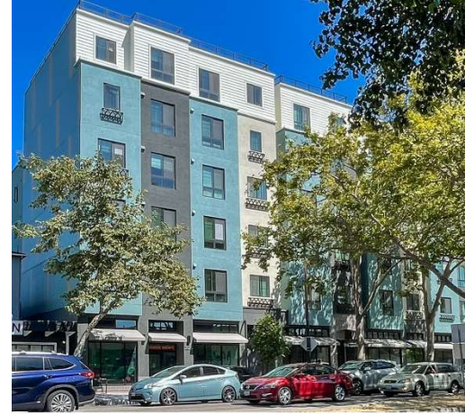
Figure 7. Building Façade with Articulation and Vertical Rhythm Photo by CD+A
