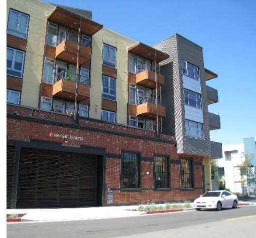
Figure 4. Parking Garage Entry Photo by AWP
