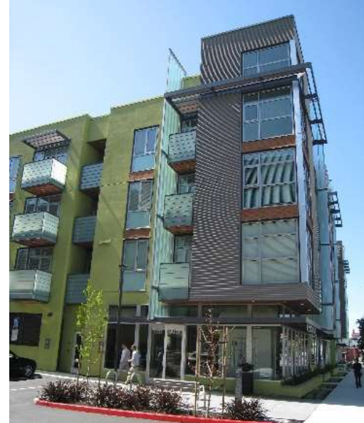
Figure 8. Building Corner with Façade Articulation
