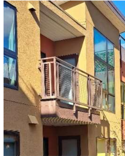
Figure 18. Balconies Photo by AWP
