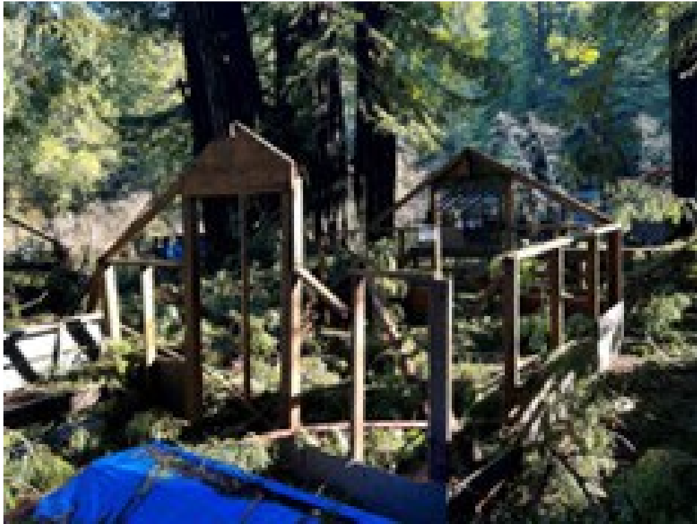
Cazadero Camp Storm Damage Recovery
