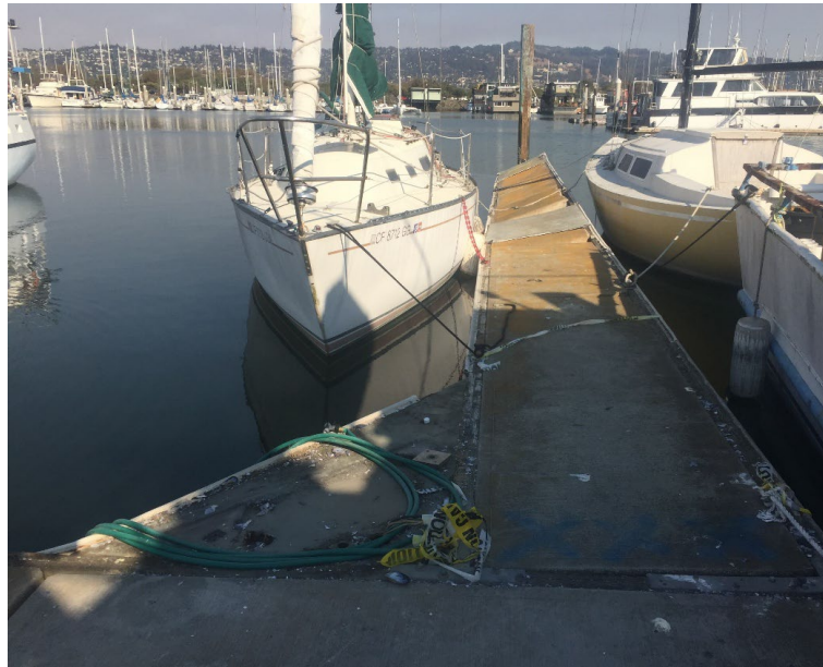
Finger Docks Replacement
