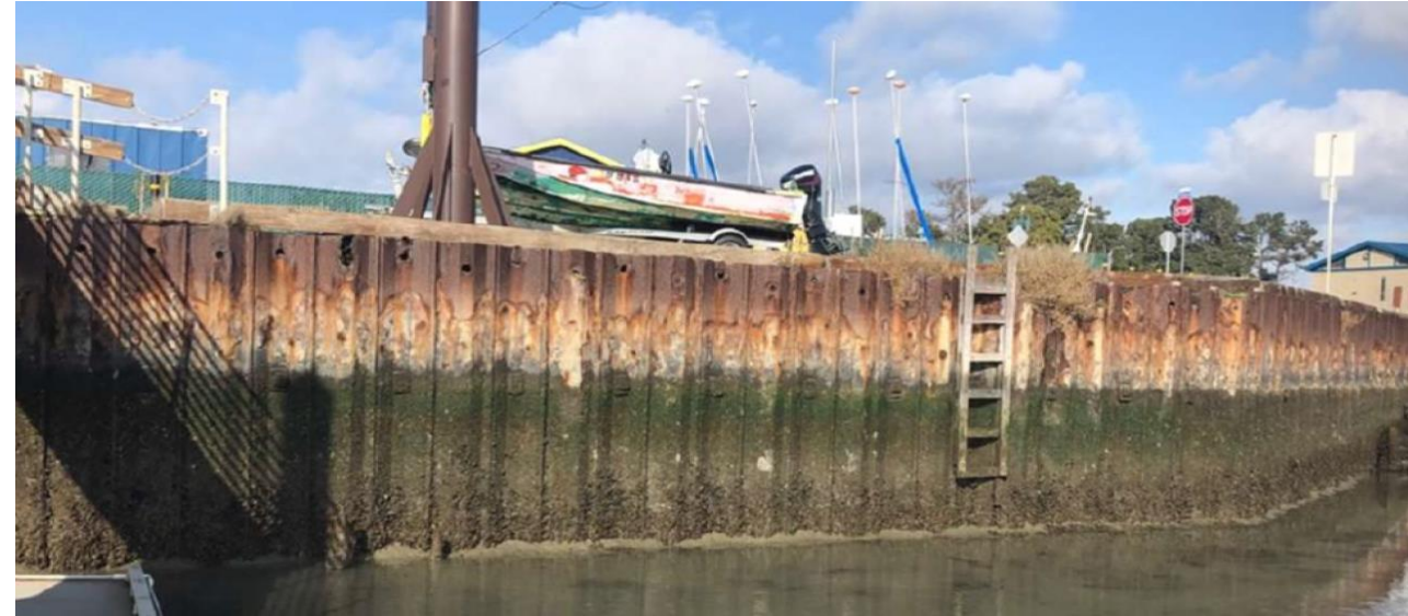
South Cove Seawall in Waterfront
