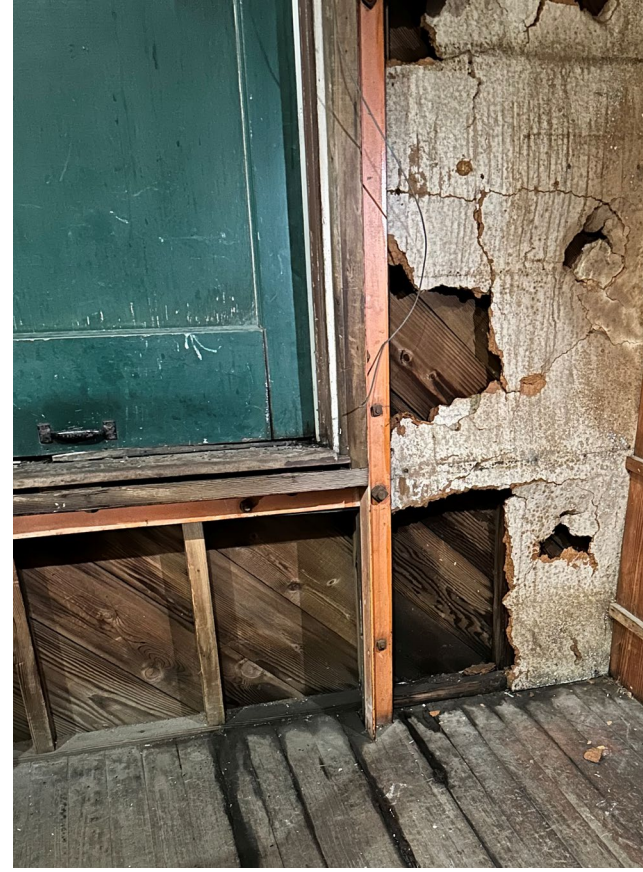
Berkeley Mental Health Services Building
