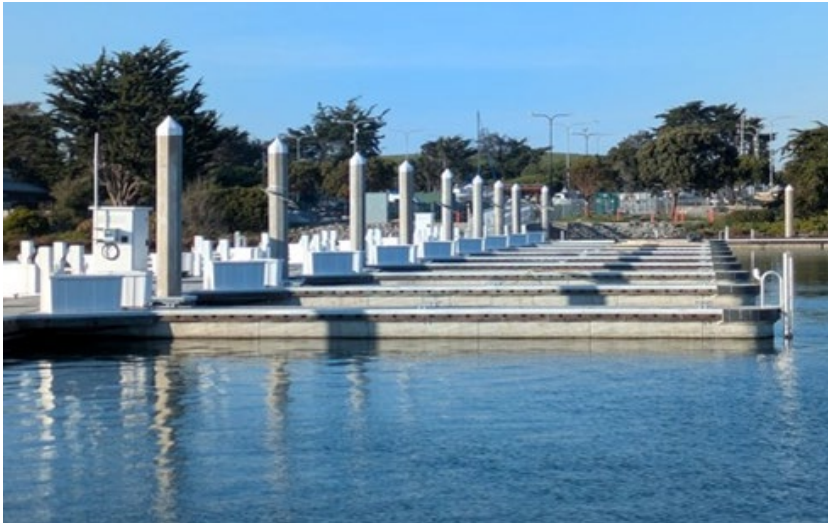
D&E Dock Replacement
