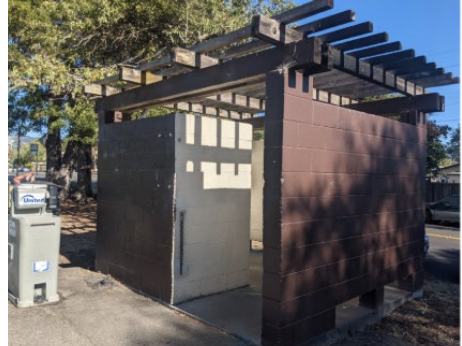
Park Restroom Replacement Project
