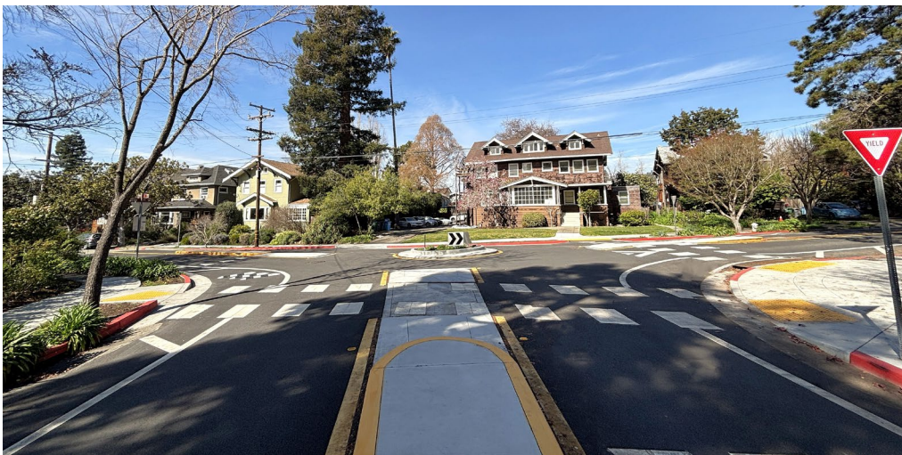
Woolsey-Eton Intersection Improvements
