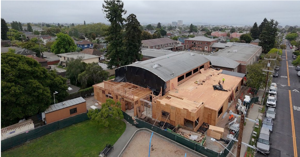
MLK YAP Renovation
