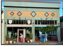
Koerber Building No. 3.
