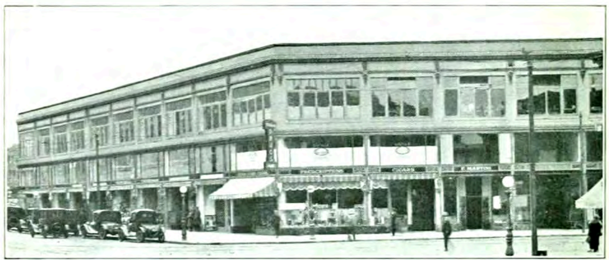
New Stores Erected by The Midgeley Company at 15th St. and San Pablo Ave.
