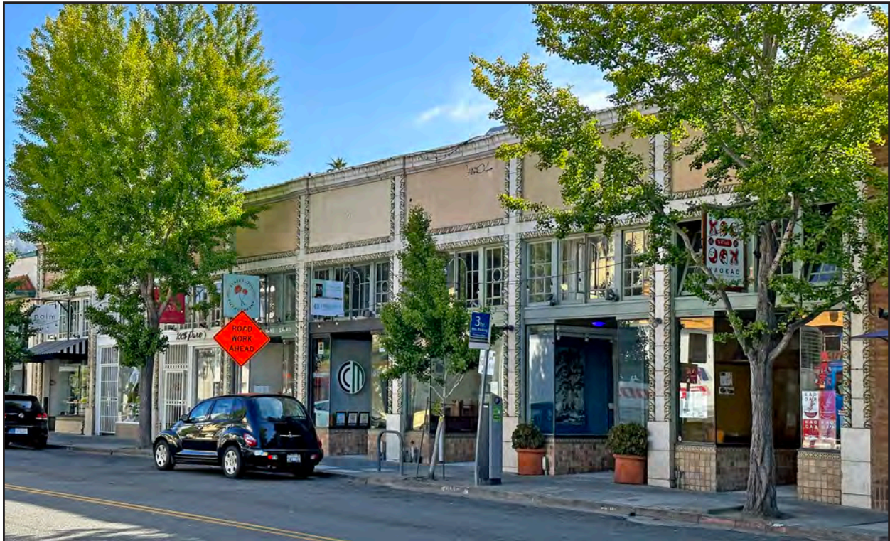
The Morris Building, 2993 College Avenue. Anthony Bruce, 2025.
