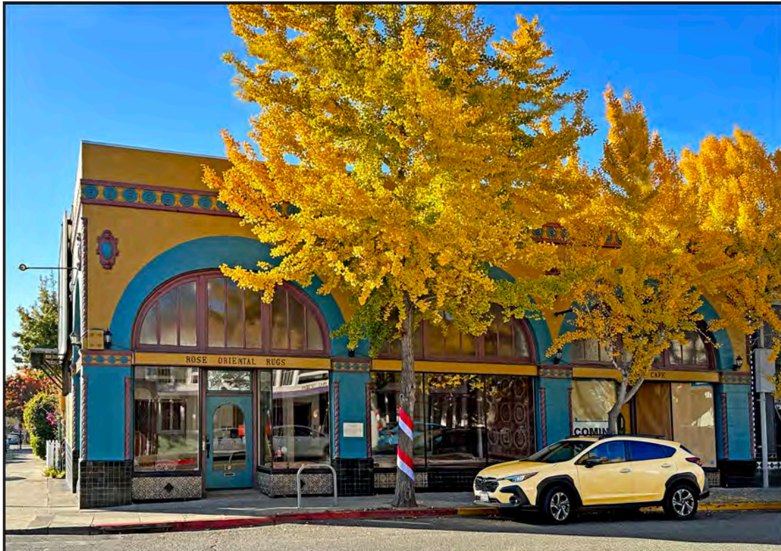
The Wilson-Tulanian Building, 2992 College Avenue. Anthony Bruce, 2025.
