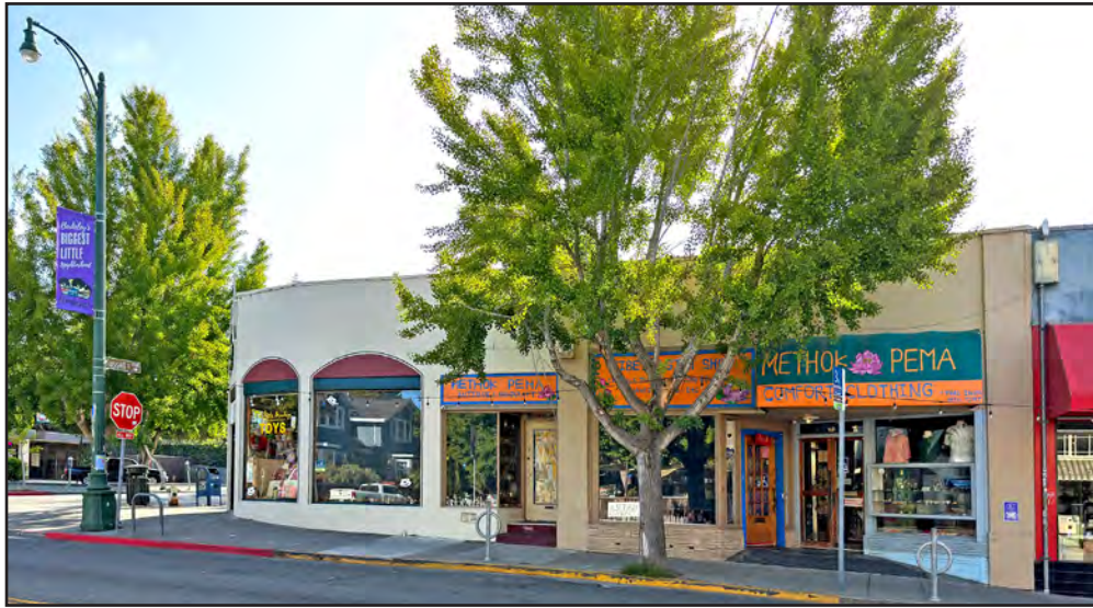
Dondero Building, College Avenue frontage. Anthony Bruce, 2025.
