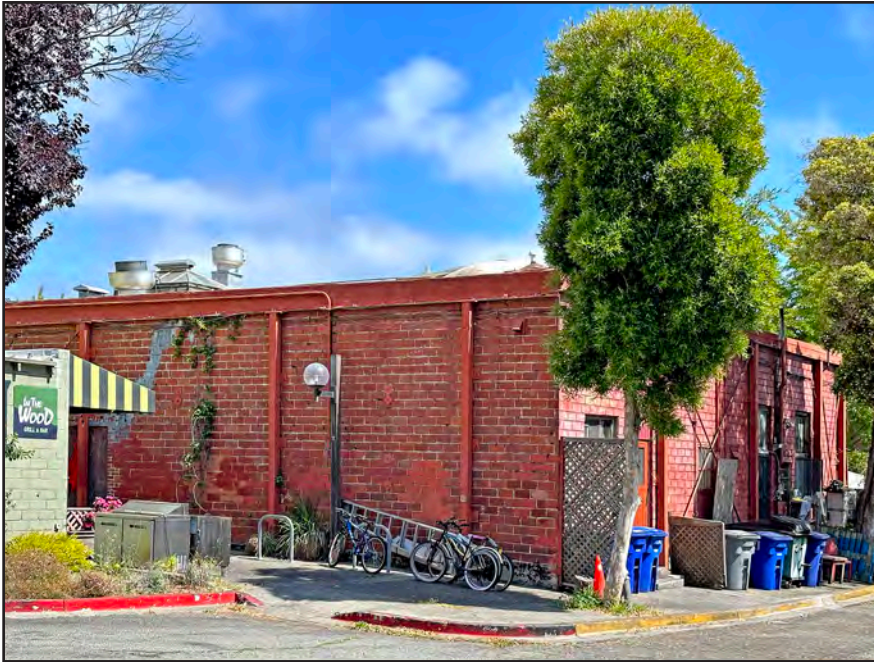
Rear of the Bischoff Shops Building No. 1, seen from the parking lot and showing original construction and later seismic bracing. Anthony Bruce, 2025.
