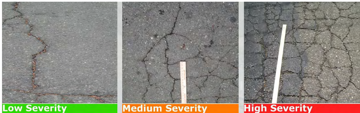
Image 1: Alligator Cracking
