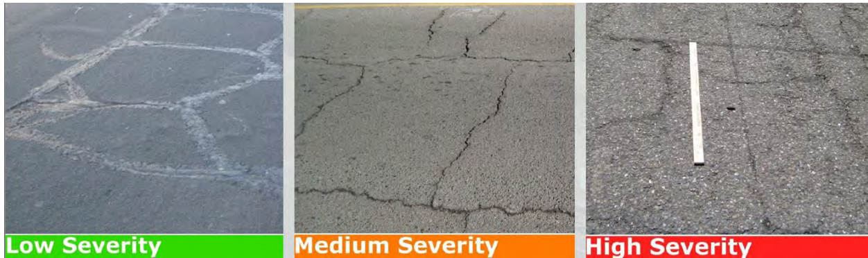
Image 2: Block Cracking
