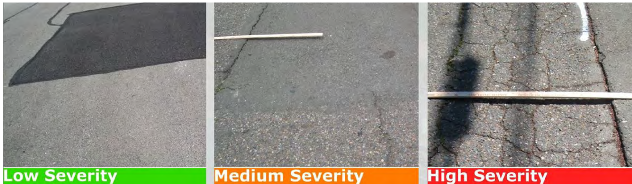
Image 5: Patching and Utility Cut Patching
