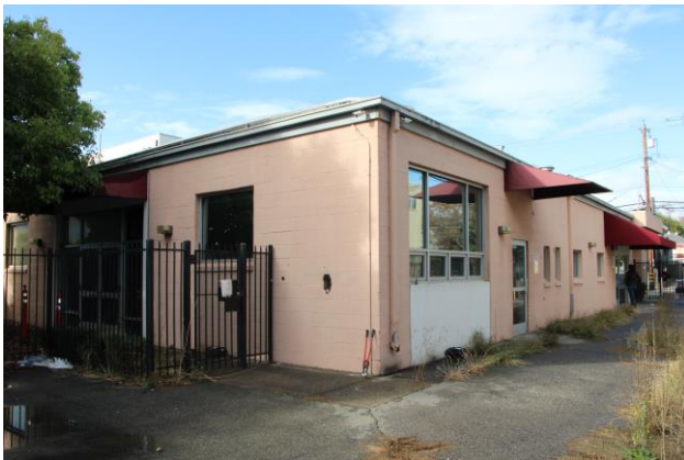
Photo 4: East and South Elevations, View Northwest
