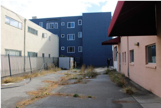
Photo 2: Paved Driveway along Eastern Portion of Property, View South
