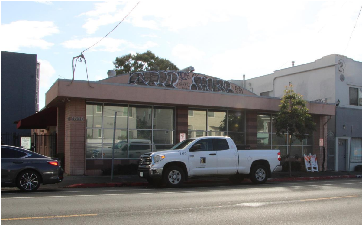
Figure 2 1890 Alcatraz Avenue North and East Elevations, View South
