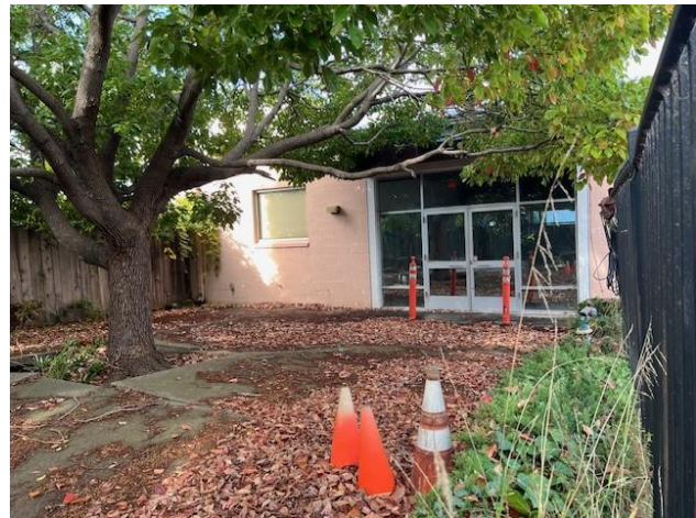
Photo 5: South Elevation and Enclosed Courtyard, View North
