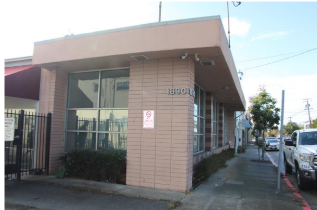
Photo 3: North (Primary) and East Elevations of Extension Along Alcatraz Avenue, View West
