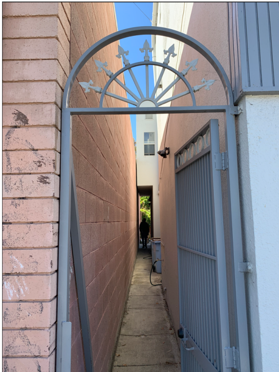
Figure 9. Exterior West Wall
