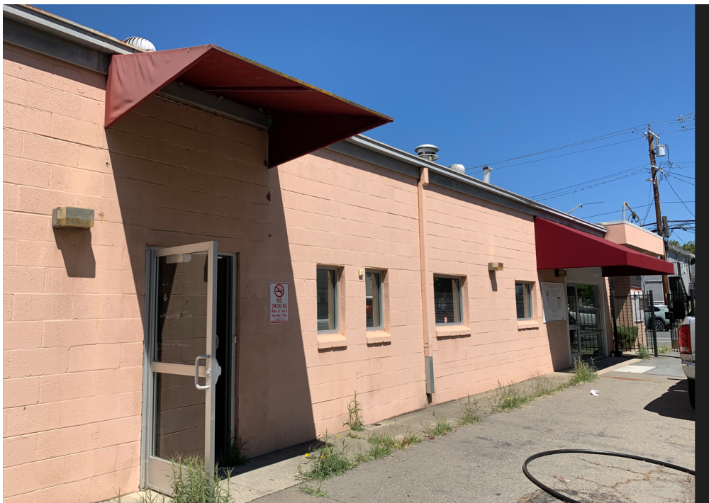
Figure 8. Exterior East Wall
