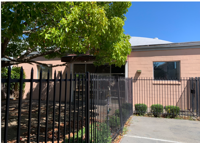
Figure 11. Exterior South Wall
