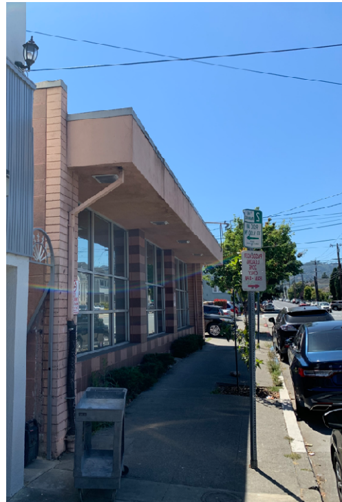
Figure 10. View looking at Front
