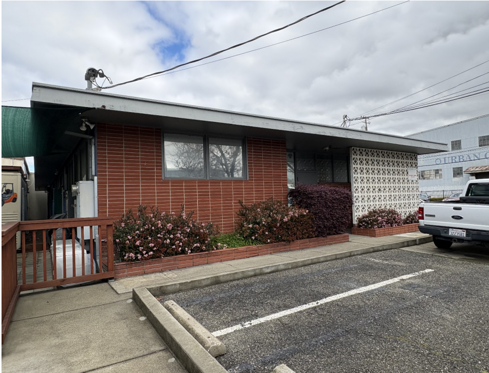
Upper primary (south) facade.
