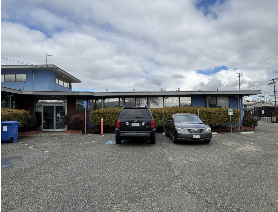
Concrete curb at front (south) of lot.
