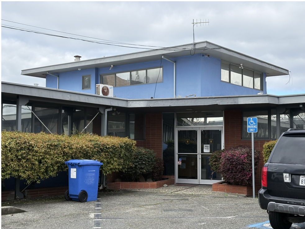
West and primary (south) facade, looking northeast.
