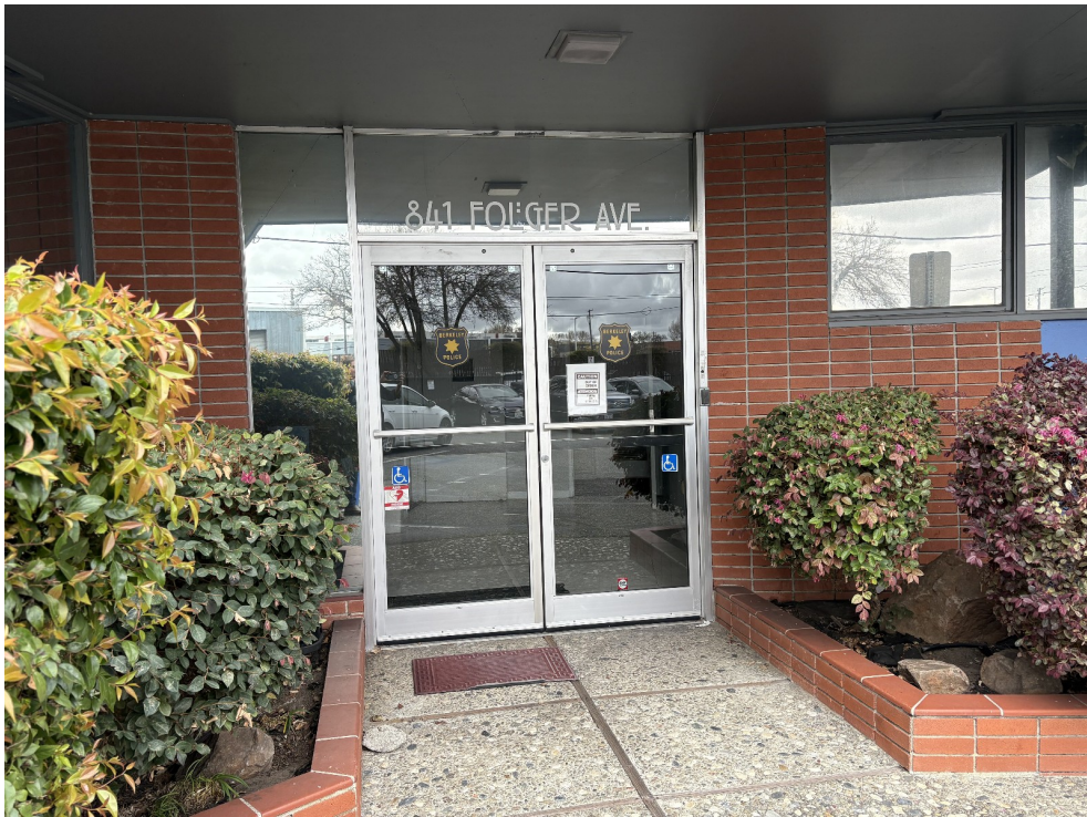
Lower primary (south) facade.
