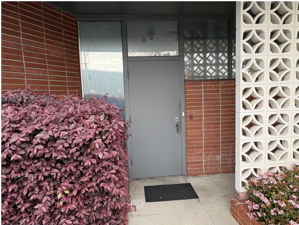
West facade, looking east.
