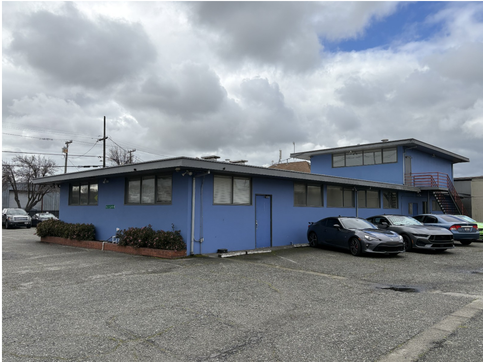
Rear (north) facade, looking south.
