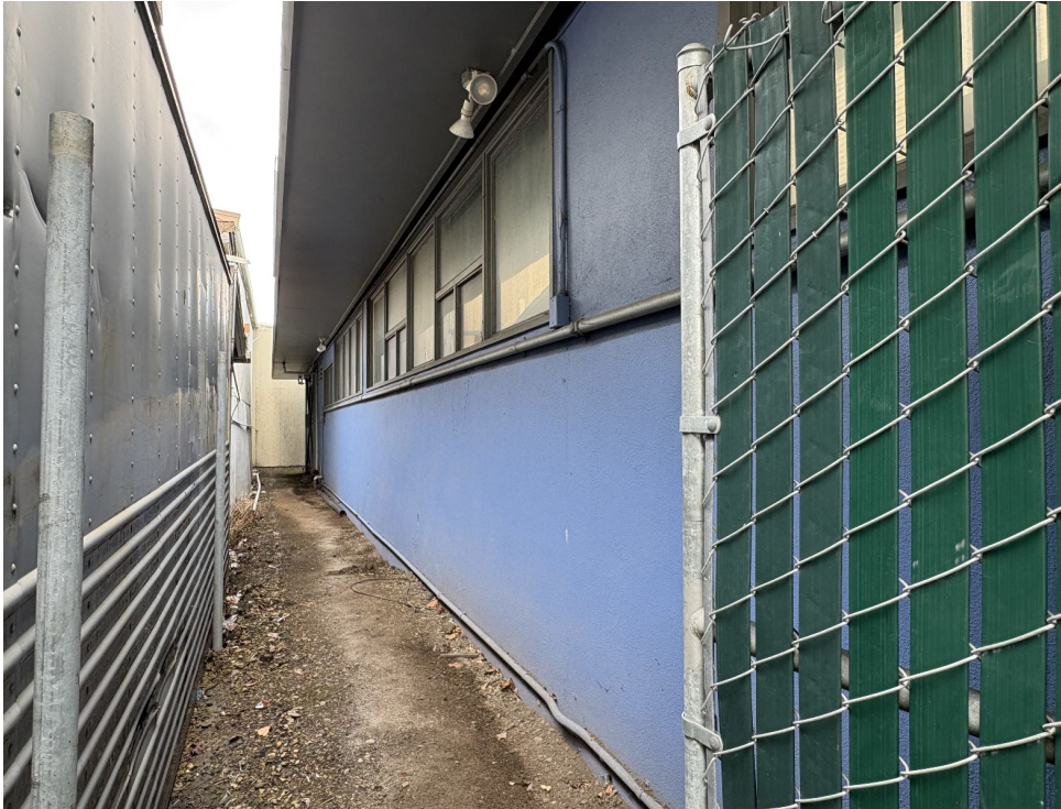
Rear (north) and west facades, looking southeast.
