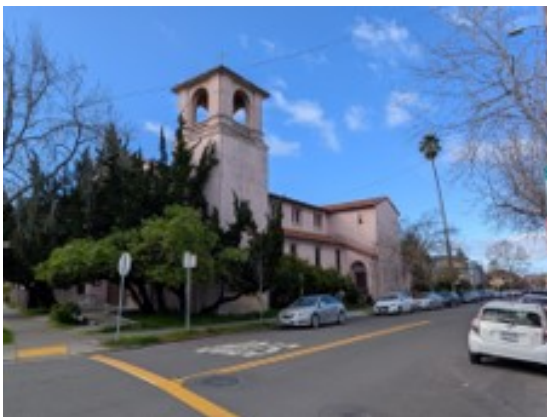
Existing church building
