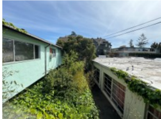
Existing landscape is overgrown and not maintained.
