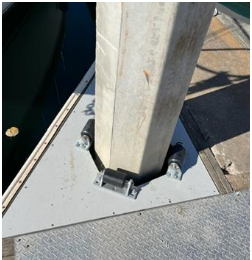
After: New long-life concrete piles
