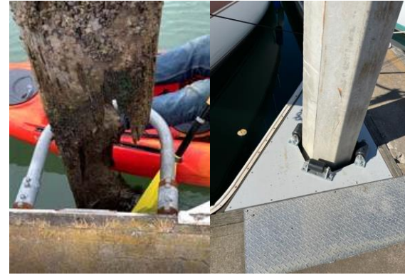
Repair and Improvements to Marina Docks Timber
