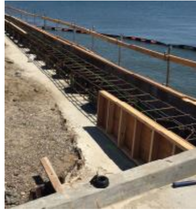
After: New, resilient seawall with sheet pile wall and enforcement structures
