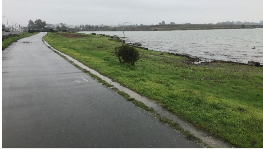
Before: Flood-prone trail
