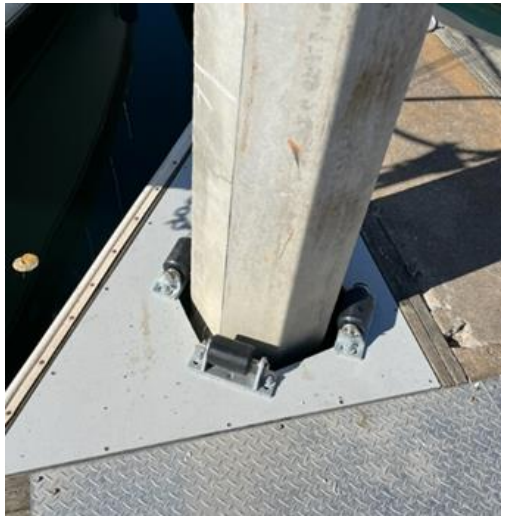
After: New long-life concrete piles
