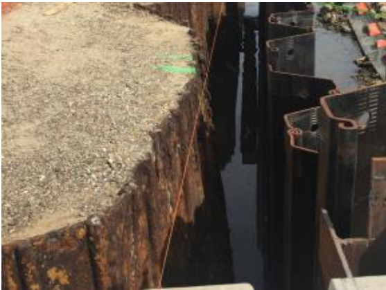
After: New, resilient seawall with sheet pile wall and enforcement structures
