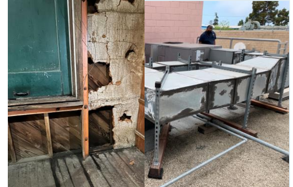
Repair and Improvements to Public Safety Facilities
