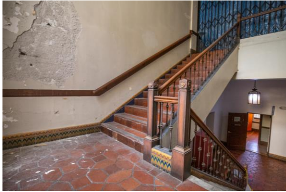
Repair and Improvements to Veterans Building
