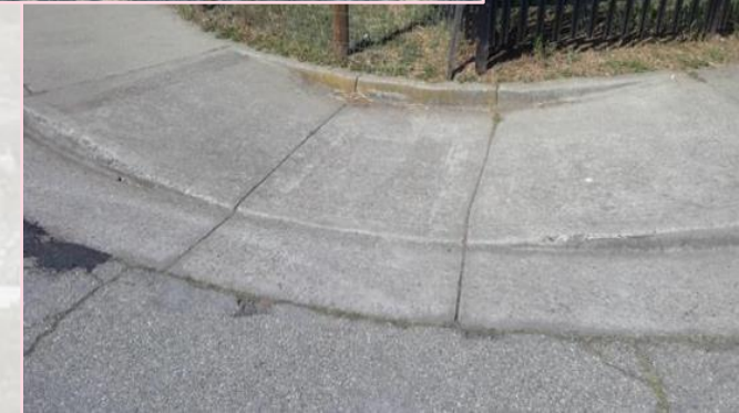
Above Images: Examples of changes in level (elevations) on sidewalks that require improvements
