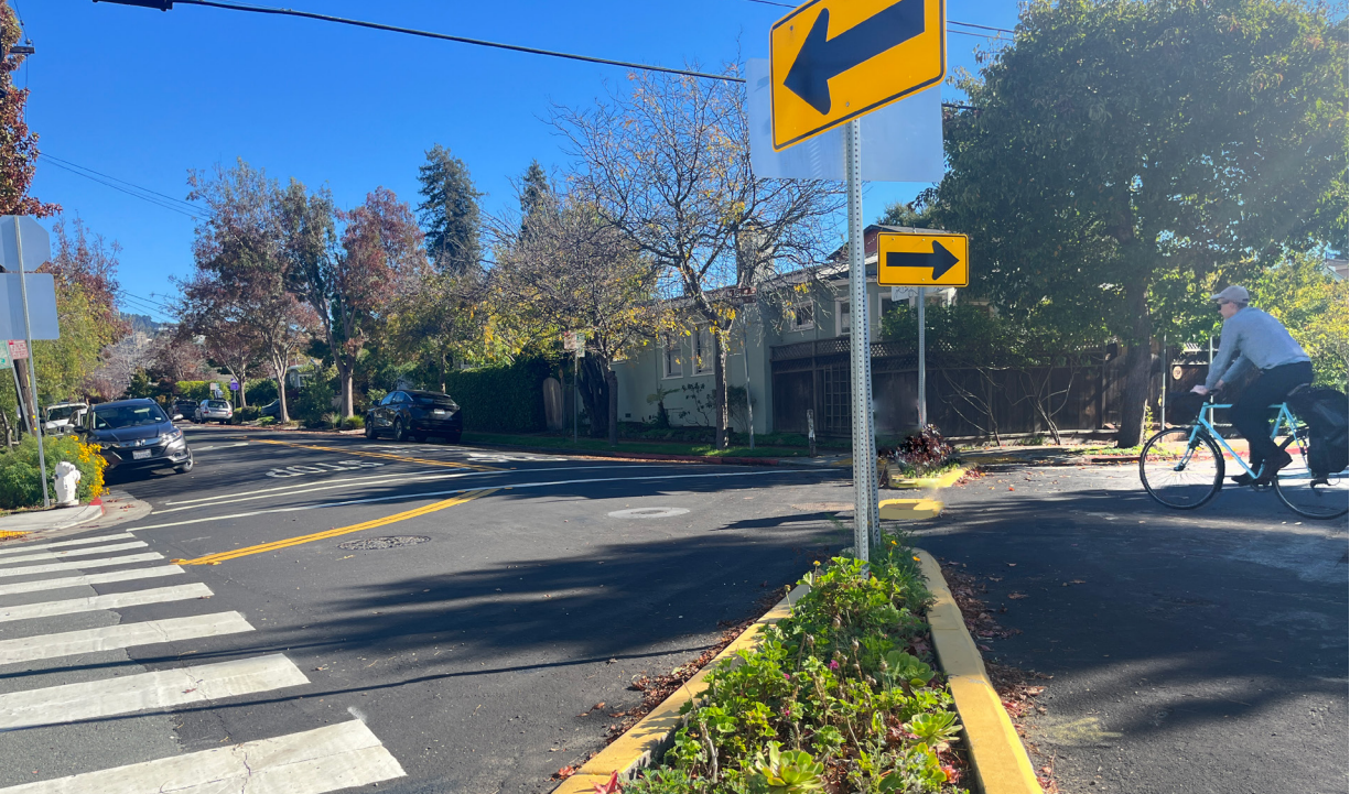
Newer Installation at Virginia and McGee (Source: City of Berkeley)
