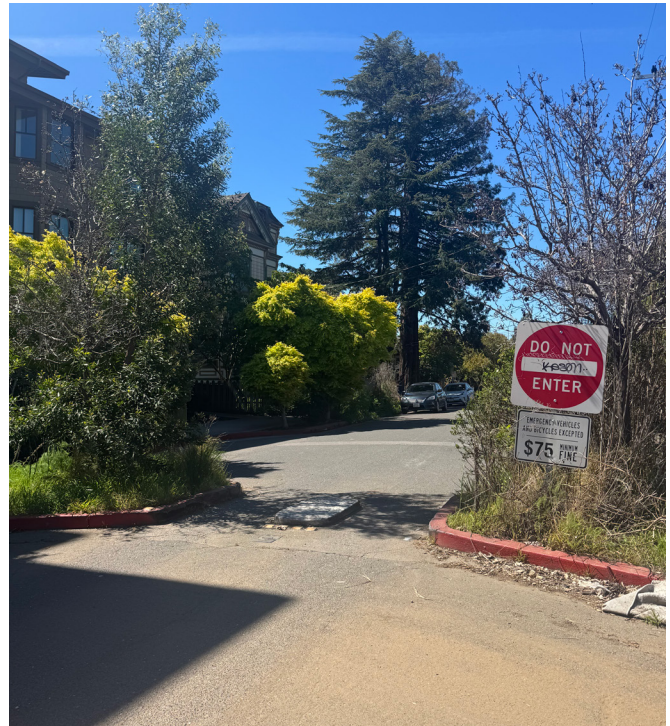
Full Diverter at Berkeley Way and Trader Joe's (Source: City of Berkeley)
