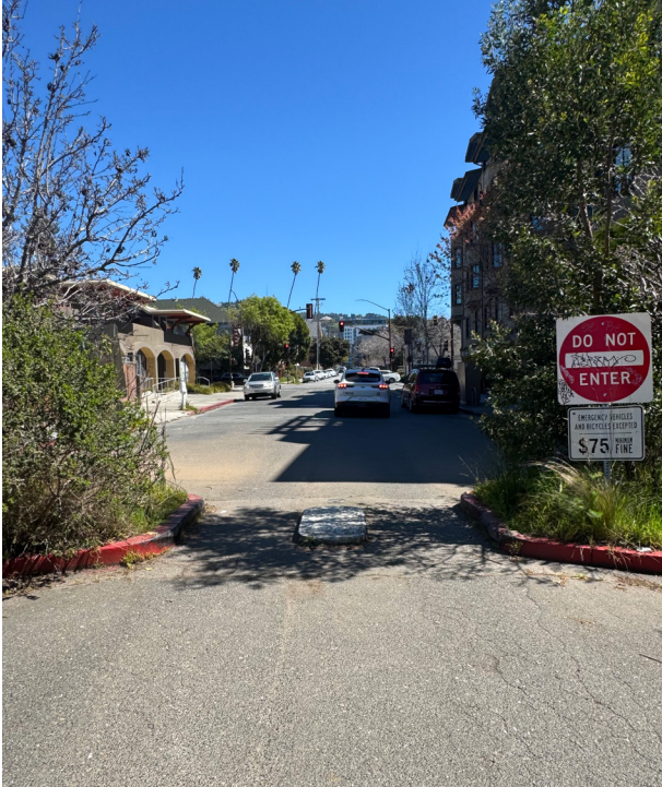
Newer Installation at Berkeley Way and Trader Joe's (Source: City of Berkeley)
