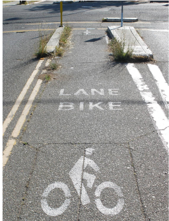
Example of a separated bike lane approaching an intersection.
