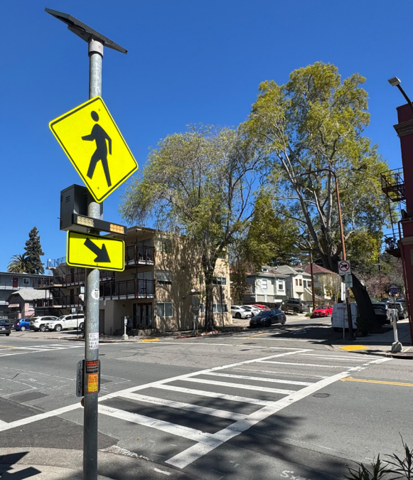
RRFB at MLK Jr. Way and Virginia Avenue (Source: City of Berkeley)
