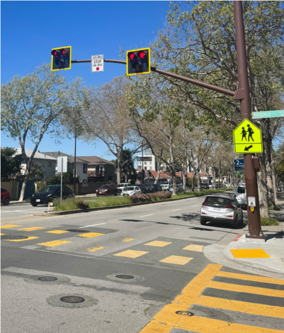
PHB at Virginia Avenue and San Pablo Avenue (Source: City of Berkeley)
