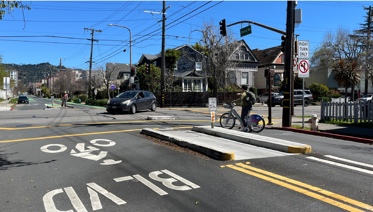
Traffic Signal with Diversion at MLK Jr. Way and Channing Way (Source: City of Berkeley)
