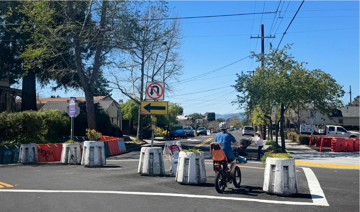
Older Installation at Virginia and Acton (Source: City of Berkeley)
