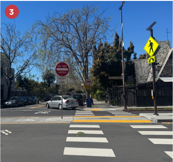
RRFB + MEDIAN CROSSING on Addison Street at MLK Jr. Way.
