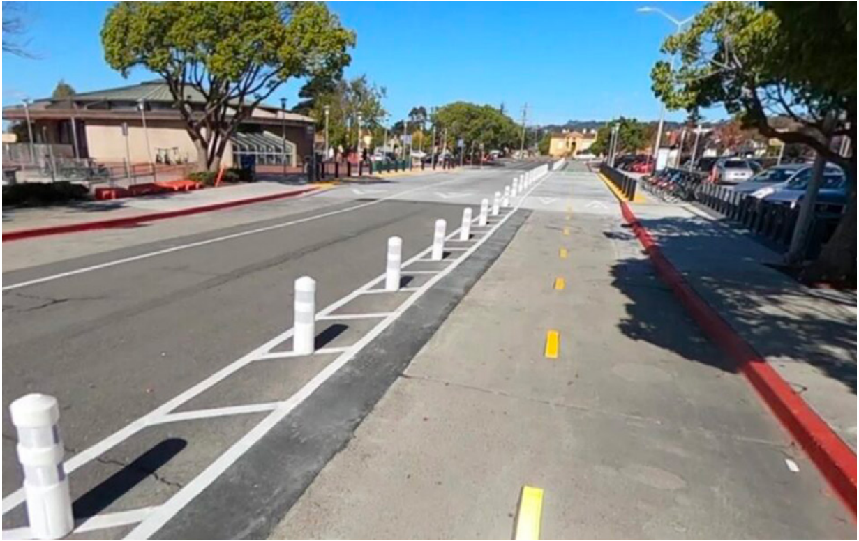
Separated bikeway at North Berkeley BART.
