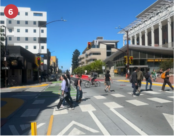
RAISED CROSSING at the intersection of Telegraph Avenue at Bancroft Street.
