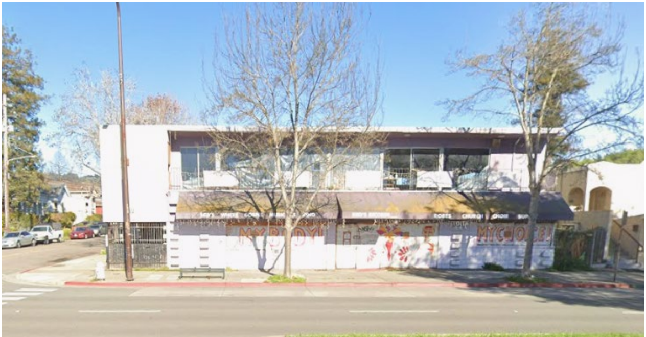
View from Sacramento Street
