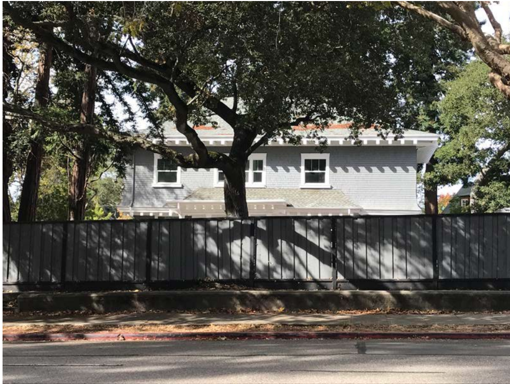
Figure 5: View from Claremont Avenue (east façade) (SAP application packet, 2026)
