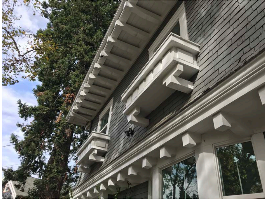
Detail at second story (south facade) showing wood planter boxes and other decorative elements
