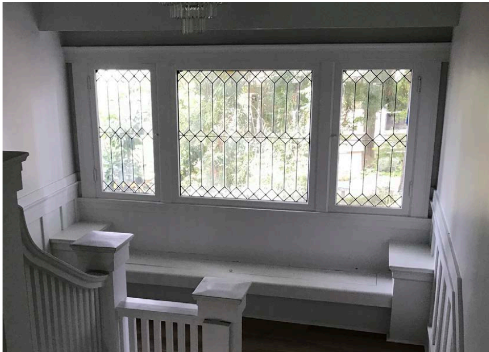
Rear (west) facade bay window from interior to illustrate leaded glass
