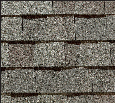
DIMENSIONAL ASPHALT SHINGLE ROOF
