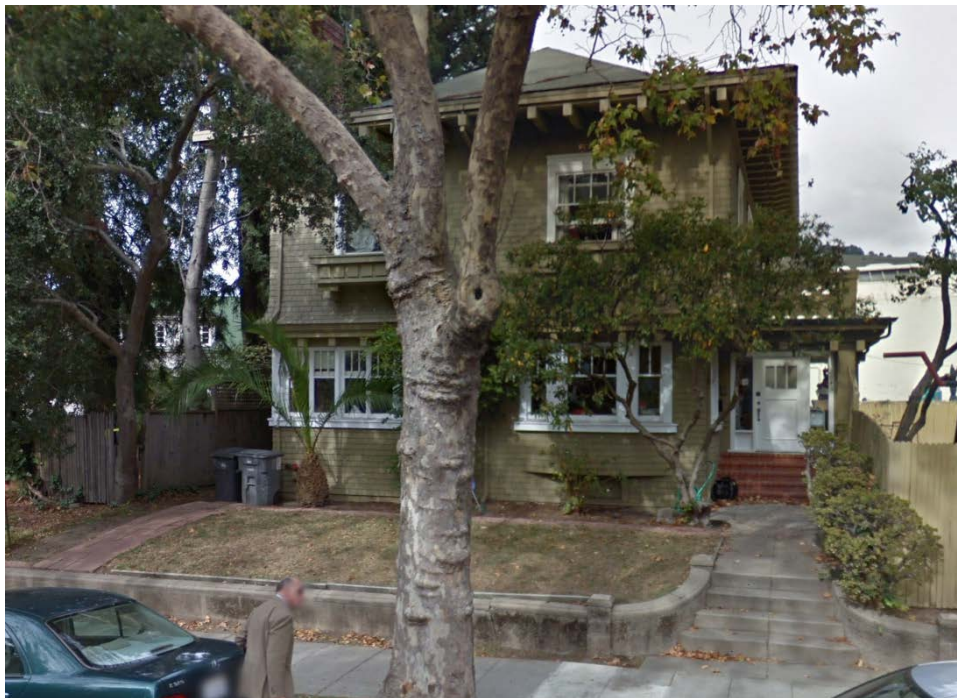
2845 Woolsey Street (south facade), looking north from Woolsey Street, c. 2014 Note original windows and enclosed porch with upper railing intact (Google Streetview)
