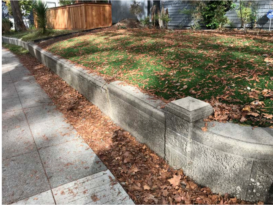
Cast stone perimeter retaining wall along Woolsey Street (south side of property)
