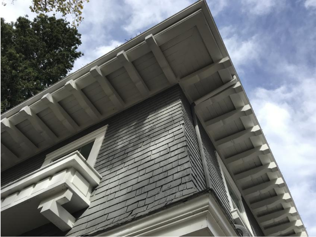
Detail of eaves, southeast corner of house.
