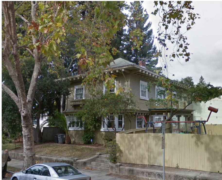
2845 Woolsey Street (south and east facades), looking northwest from Woolsey Street, c. 2014 Note original windows and enclosed porch with upper railing intact. (Google Streetview)
