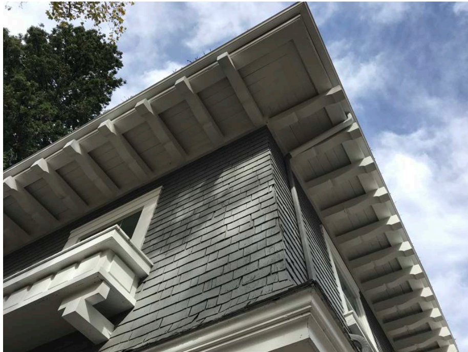
Detail of roofline showing eaves with decorative modillions and other trim
