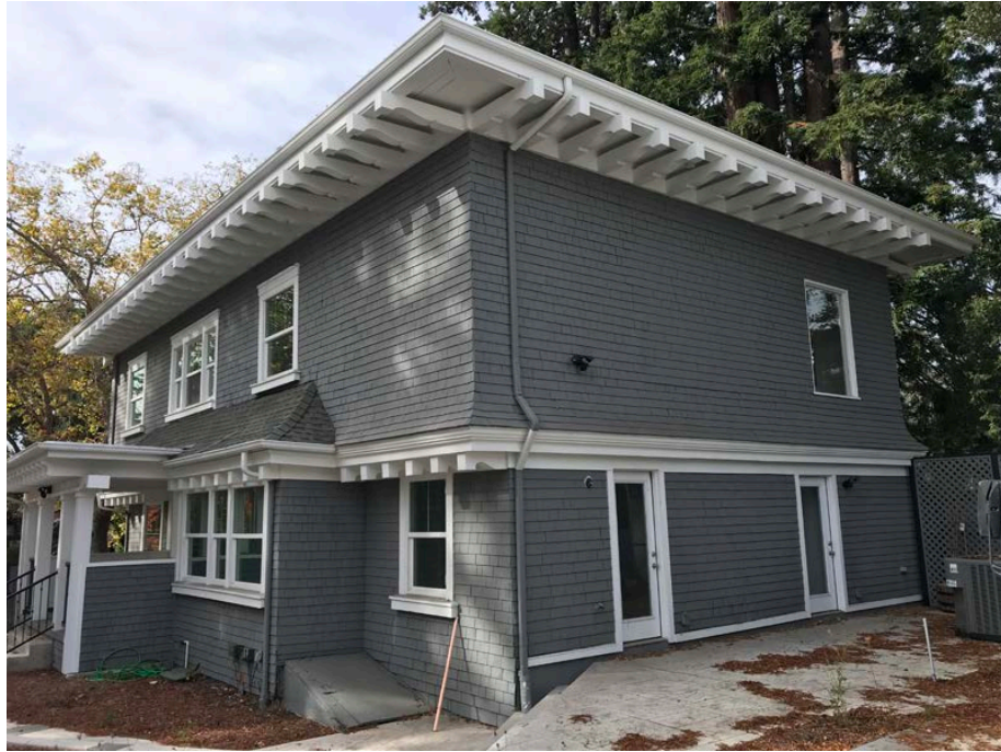
View of primary (east) and north facades, looking southwest from within property
