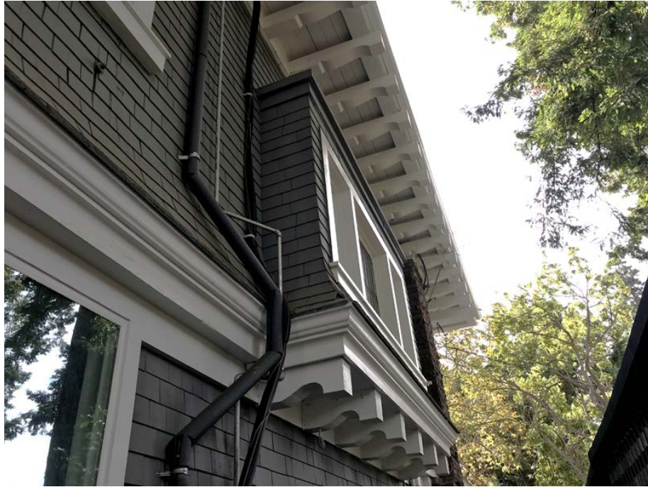
Detail of original bay window with leaded glass on rear (west) facade
