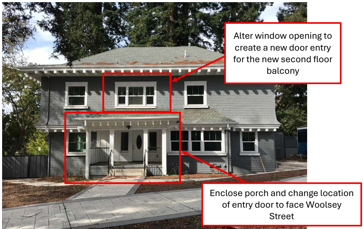
Figure 10: Subject Property, front/east façade looking within property boundaries (SAP application packet, 2026)
