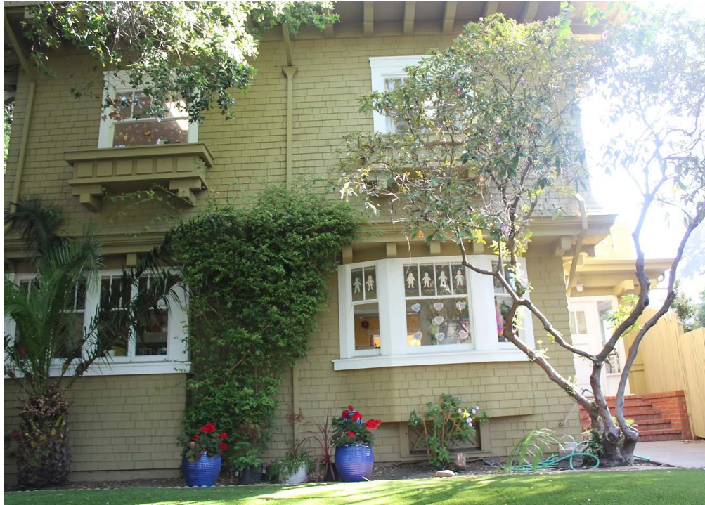
View of Woolsey Street (south facade), recent nursery school era, c. 2000s Note original windows with unequal sash and narrow divided lite configuration on upper sash (Berkeley Architectural Heritage Association)
