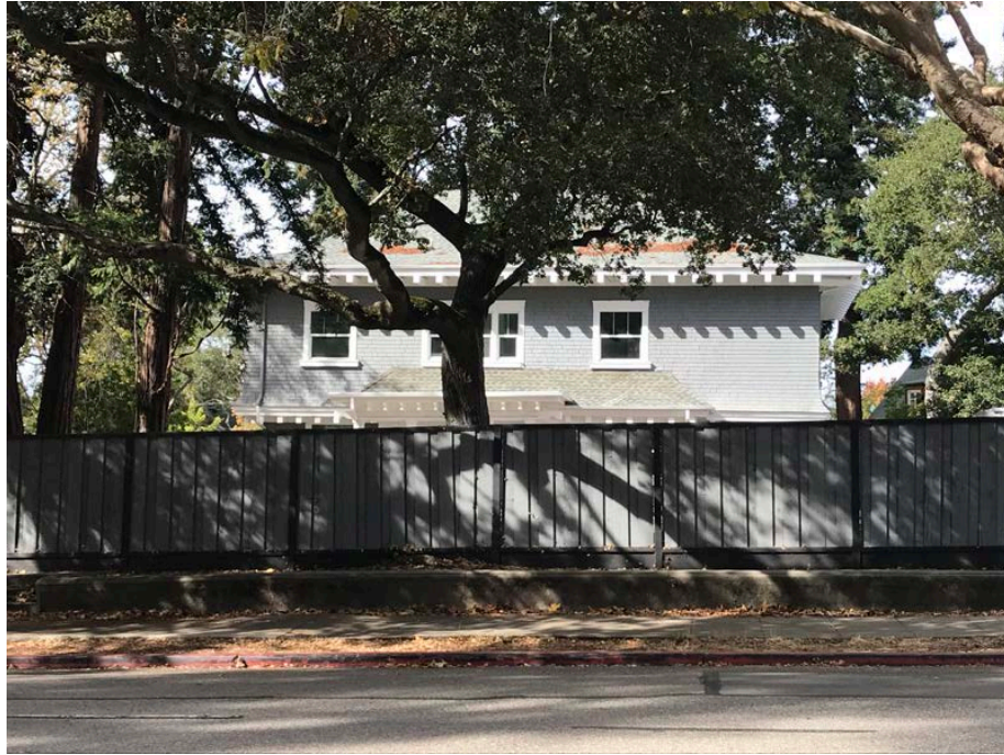
View of primary (east) facade, looking northwest from Claremont Avenue
