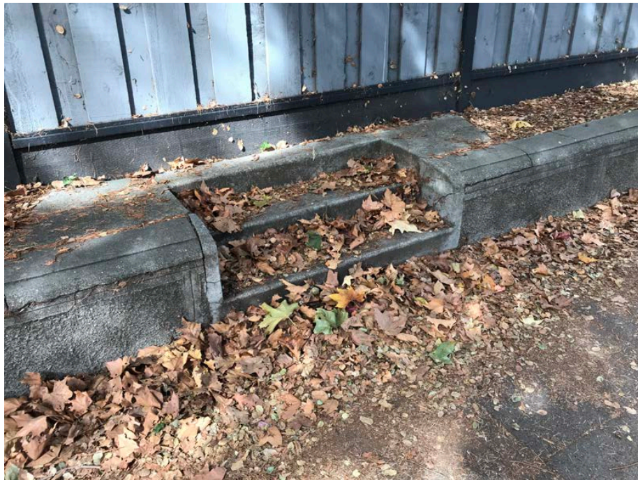
Cast stone perimeter retaining wall along Claremont Avenue (east side of property)
