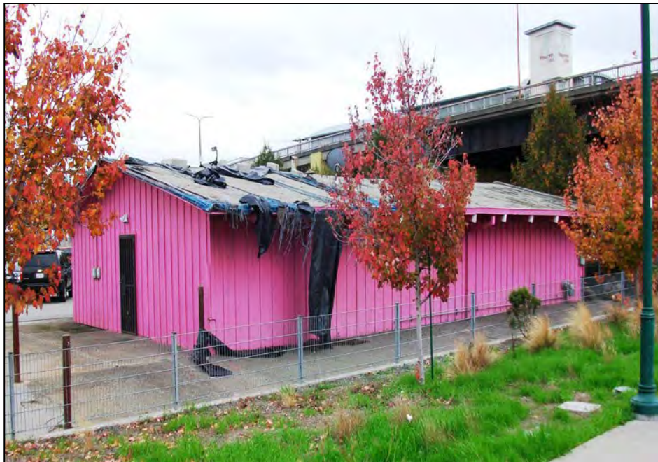
701 University Avenue. North and east façades. View from Berkeley Amtrak Station platform southeast towards University Avenue Overcrossing. 12/18/15.
