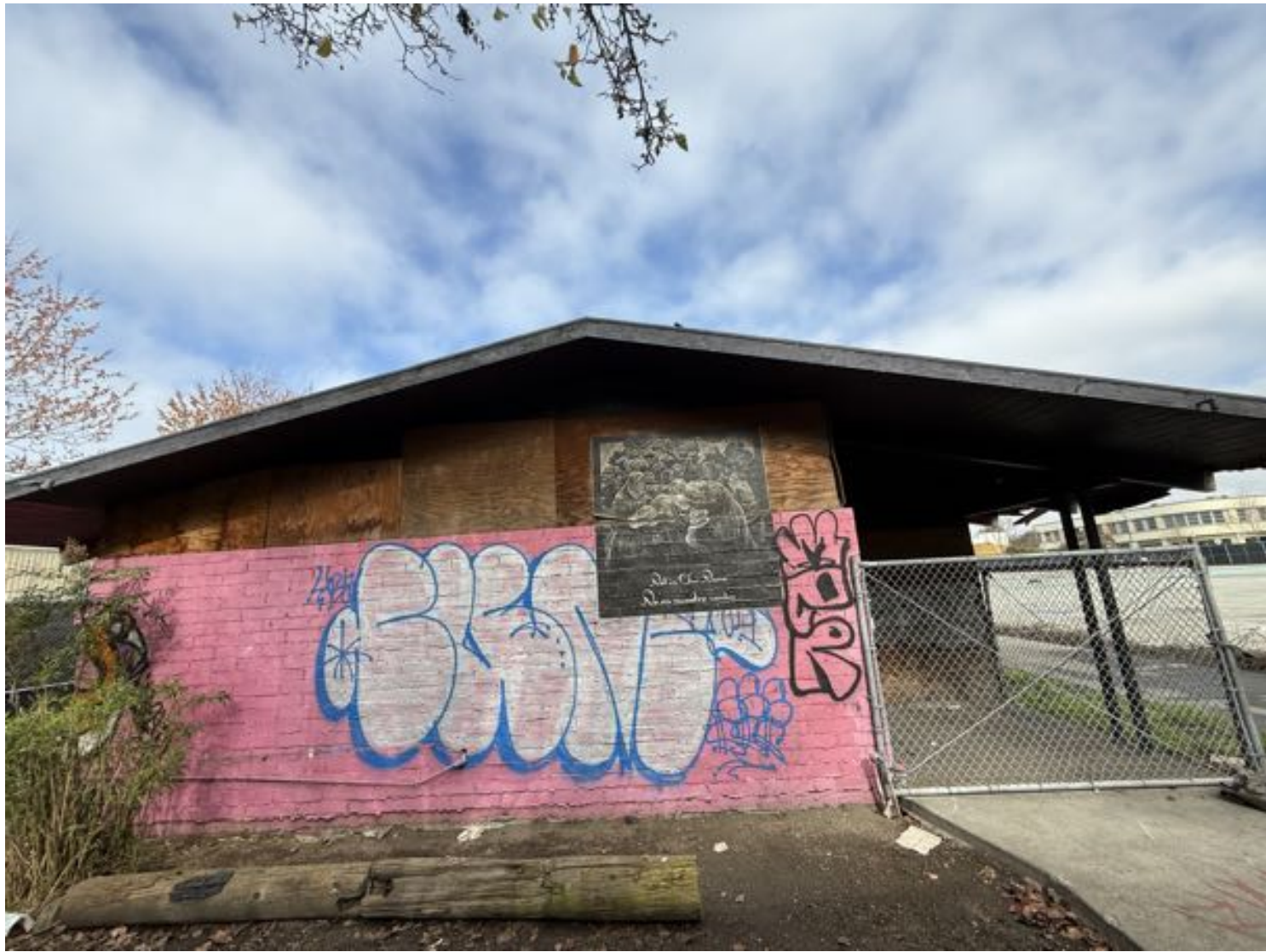
STRUCTURE TO BE DEMOLISHED - SOUTH ELEVATION
