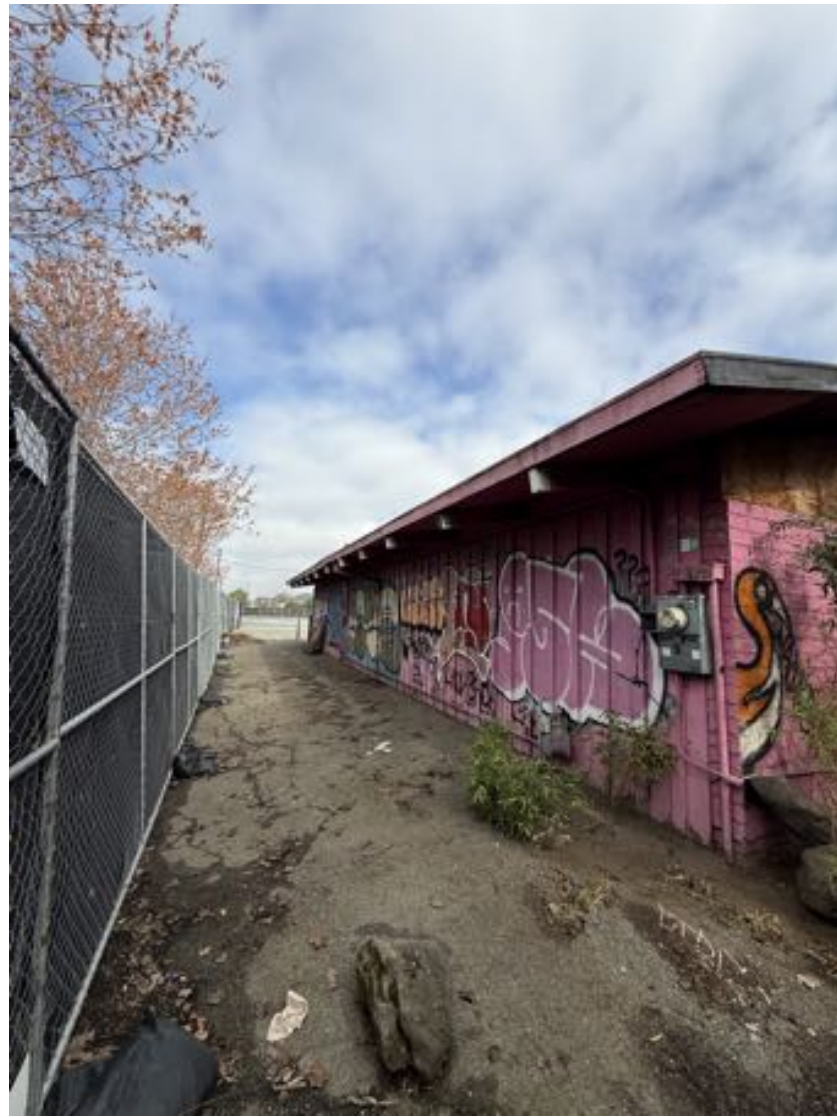
STRUCTURE TO BE DEMOLISHED - WEST ELEVATION
