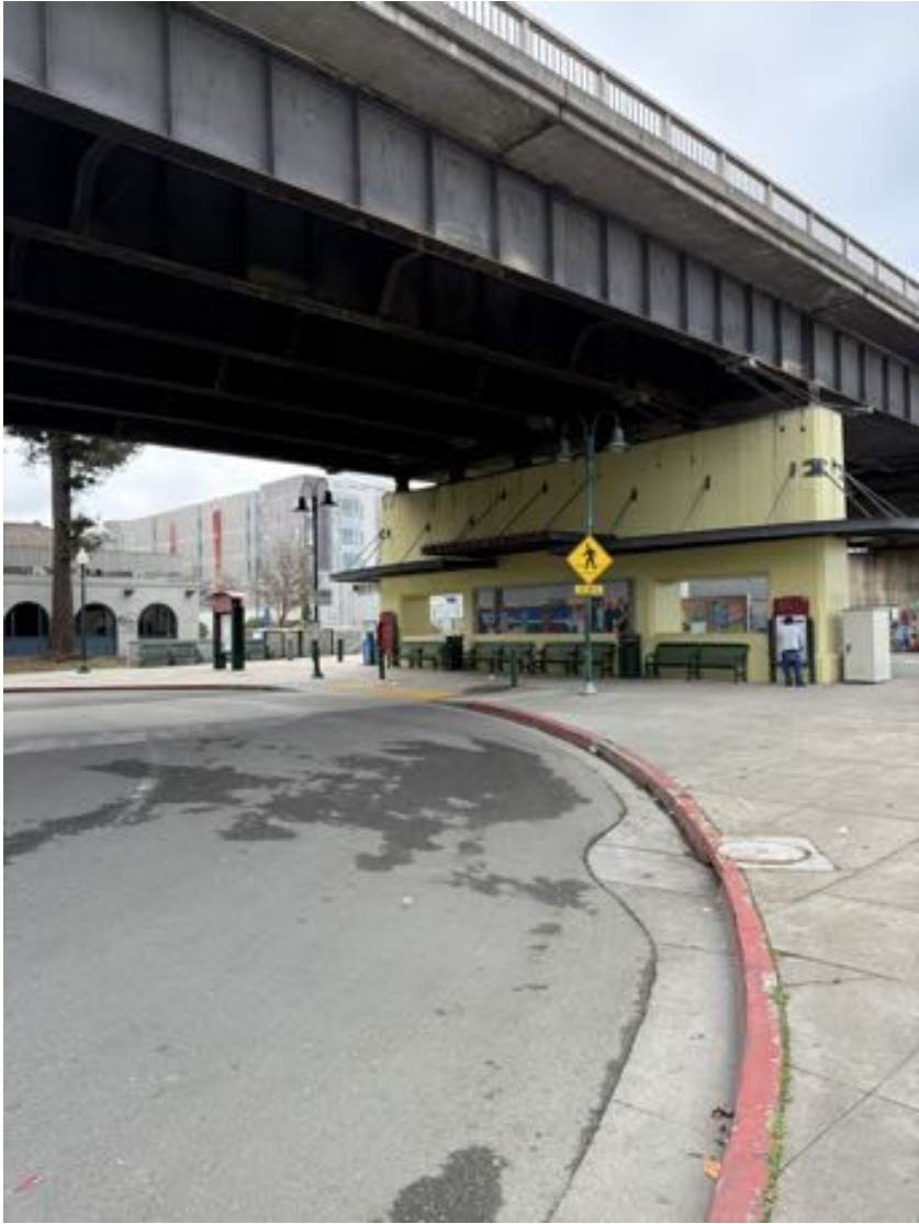
VIEW ALONG UNIVERSITY AVE. TOWARDS WEST
