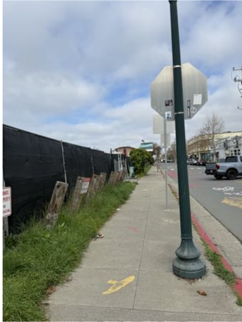
VIEW ALONG 4TH ST. TOWARDS NORTH
