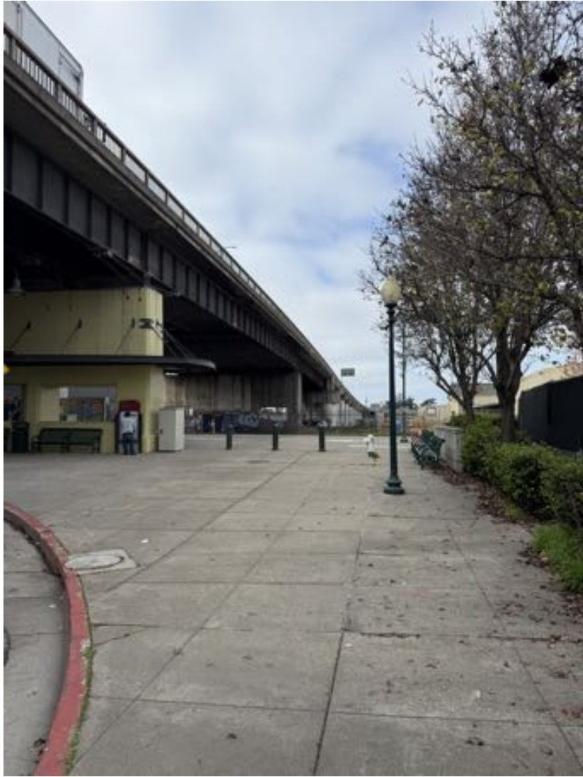
VIEW ALONG UNIVERSITY AVE. TOWARDS WEST
