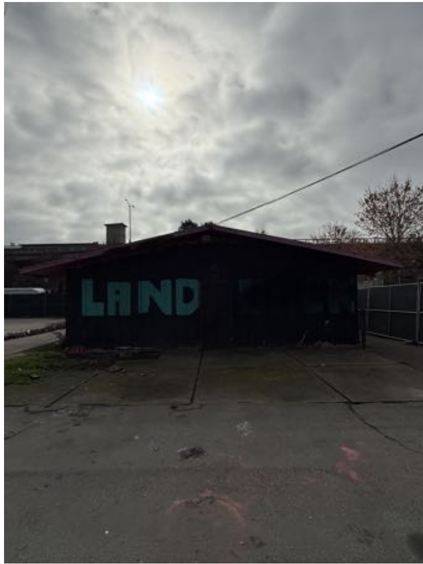
STRUCTURE TO BE DEMOLISHED - NORTH ELEVATION
