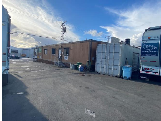
Front (south) elevation, view to northwest
