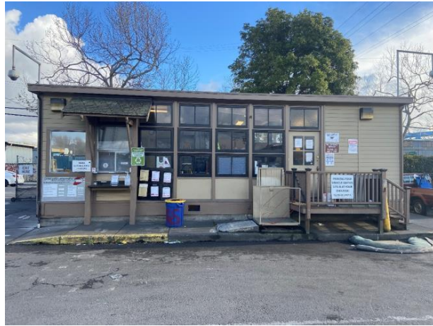
Front (north) elevation, view to south
