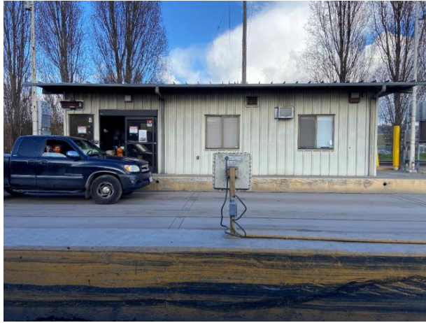
Front (west) elevation, view to east
