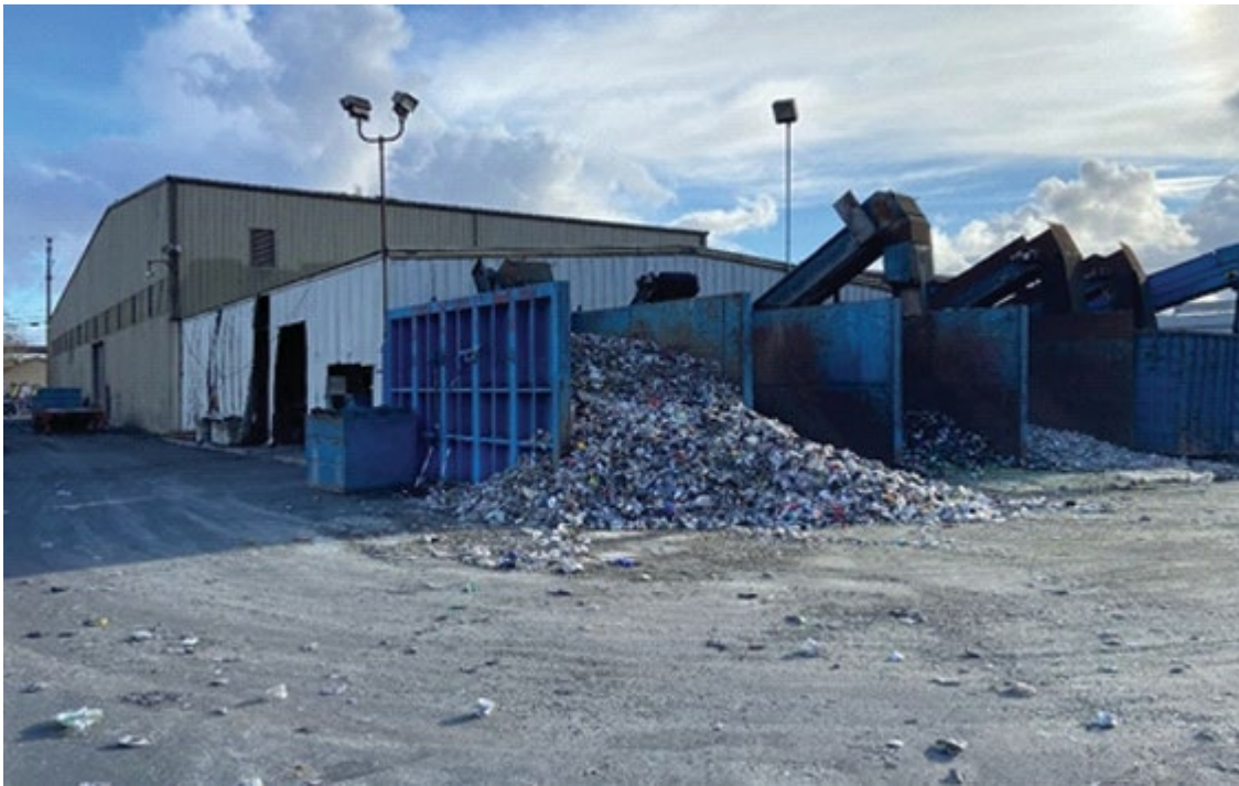
Photo 13: Materials sorting bins and container sorting facility. Built in 1982 - modified/reoriented in the 1990s.
