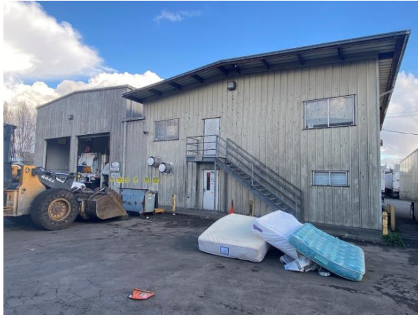
Front (north) elevation, view to southeast
