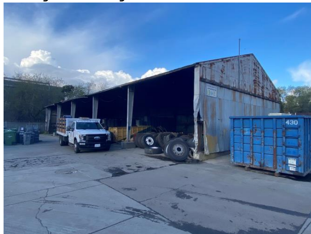
West and south elevations, view to northeast
