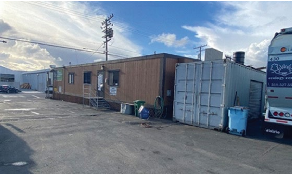
Photo 12: View of Ecology Center Inc. Administrative office. Built c. 2005-2009.
