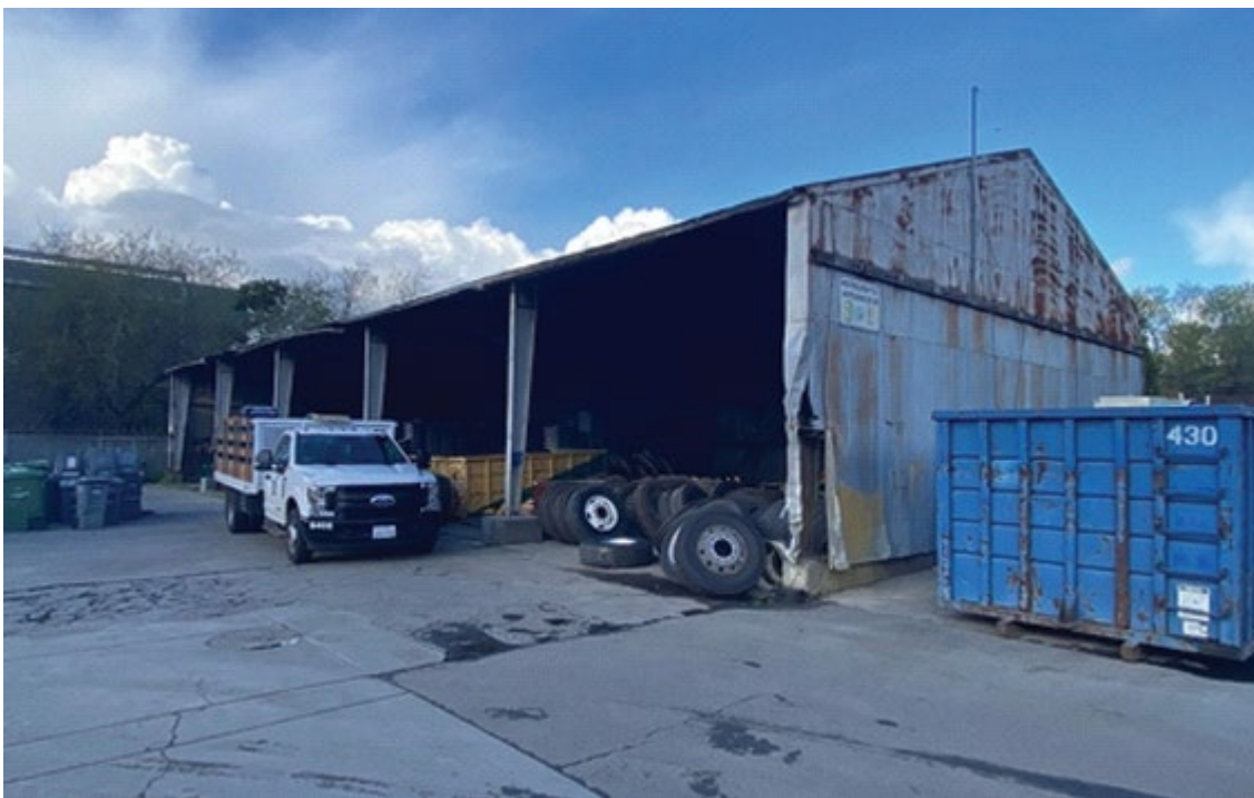
Photo 6: Storage building. Built c. 1955.
