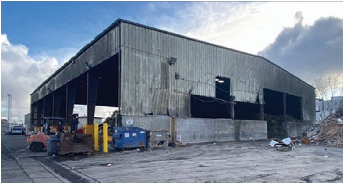
Photo 5: Construction and demolition debris staging area (foreground) and refuse and green waste staging area with transfer station in background. Built 1983.
