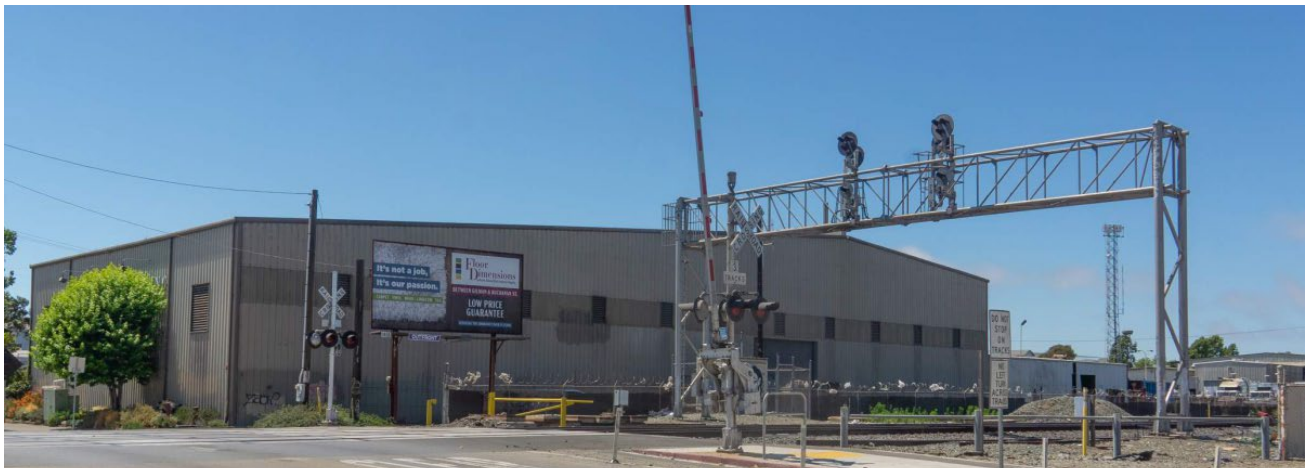
View 3: Existing view from Gilman Street and the Union Pacific Railroad tracks looking northwest toward the project site. (Source: FCS)
