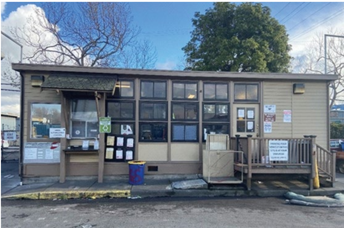
Photo 10: Community Conservation Center Inc.'s office. Built in 1982.
