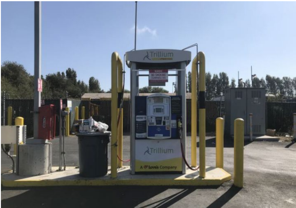
Photo 7: Fueling station within a paved lot. Built date unknown.
