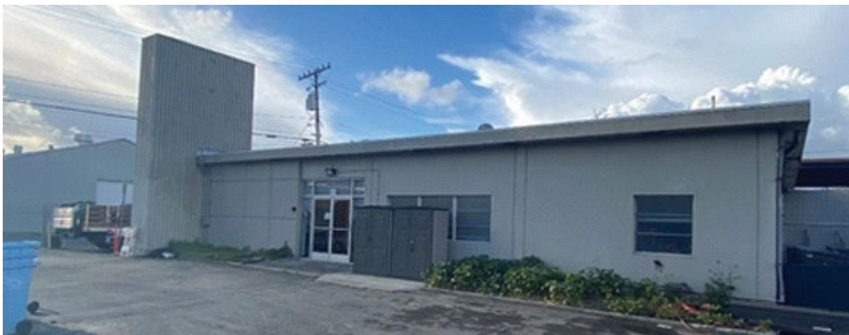
Photo 2: Administrative Building #1, view to northwest. Zero Waste Administrative Building (known as "Airco building." Built in 1955.
