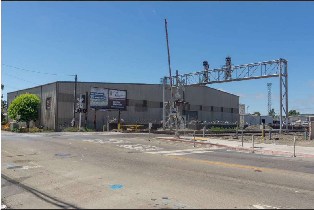
Photograph A: View 4 Existing - View from Gilman Street and the Union Pacific Railroad tracks looking northwest toward the project site.
