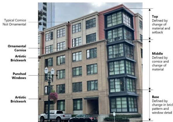
Figure 10. Example of Ornamental Façade
