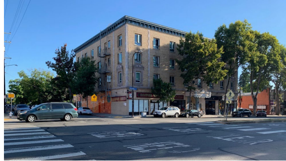
University intersection looking northeast.
