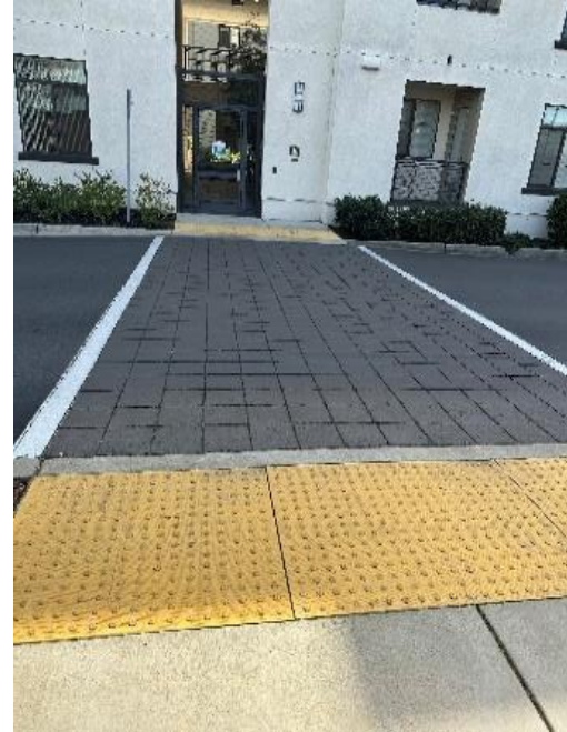
Figure 3. Elevated Walkway Crossing Photo by AWP
