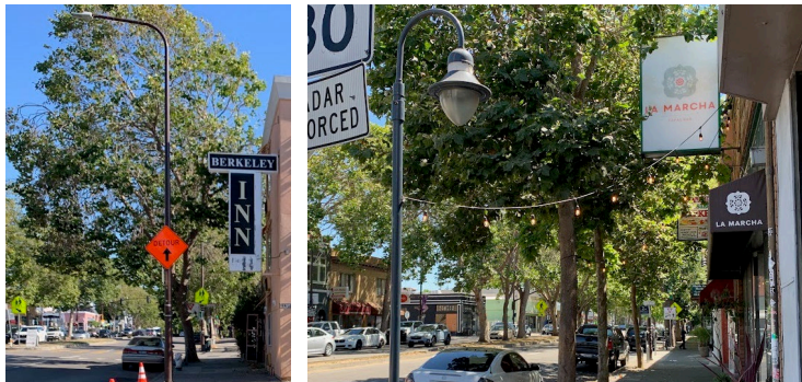
Figure 24. Existing roadway and pedestrian lighting.
