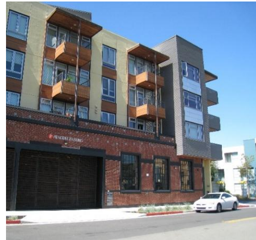
Figure 4. Parking Garage Entry Photo by AWP
