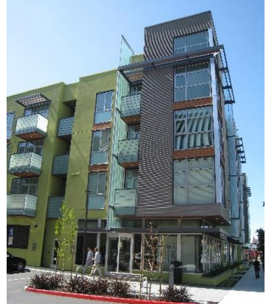
Figure 8. Building Corner with Façade Articulation Photo by AWP
