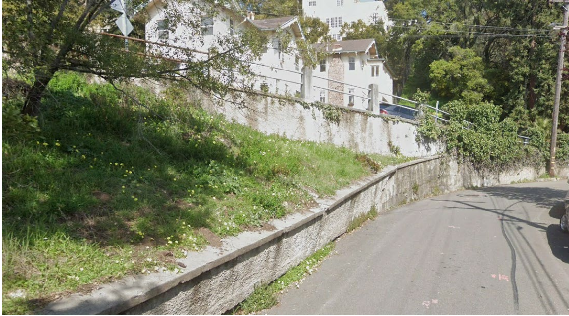
Figure 1 Daley's Scenic Park Tract Wall at Hilgard Avenue in March 2025, facing south; Source: Google Earth
