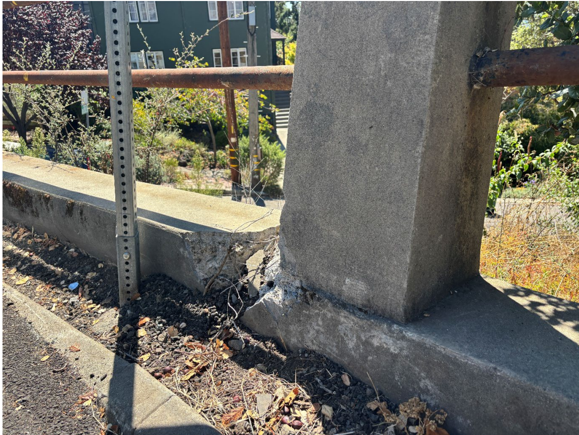
Figure 3 Daley's Scenic Park Tract Wall detail at La Loma Avenue, current view, facing south; Source: Staff Site Visit, September 2026
