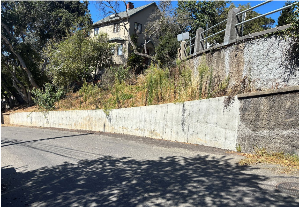
Daley's Scenic Park Tract Wall at Hilgard Avenue, facing north; Source: Staff Site Visit, September 2026
