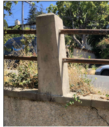
INTERIOR PILASTER REPLACEMENT EXAMPLE
