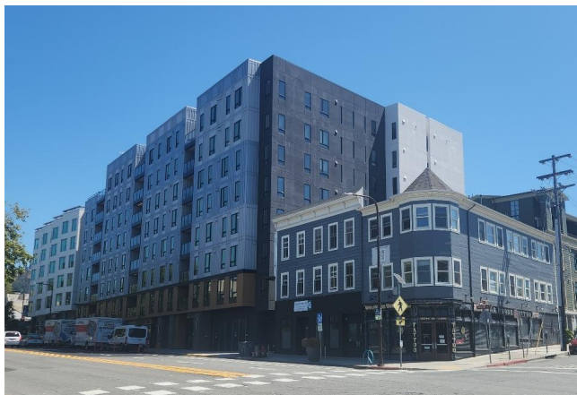
Figure 6: Mixed-use buildings immediately south of the subject property. Looking northeast from the intersection of Parker Street and Telegraph Avenue. 2599 Telegraph Avenue (built 1880), at the corner, is a City of Berkeley Landmark.
