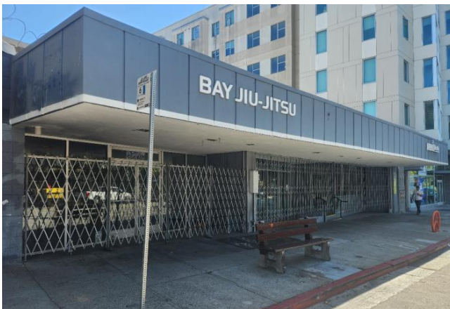
Figure 2: Oblique view of storefront at the primary façade. Looking southeast.
