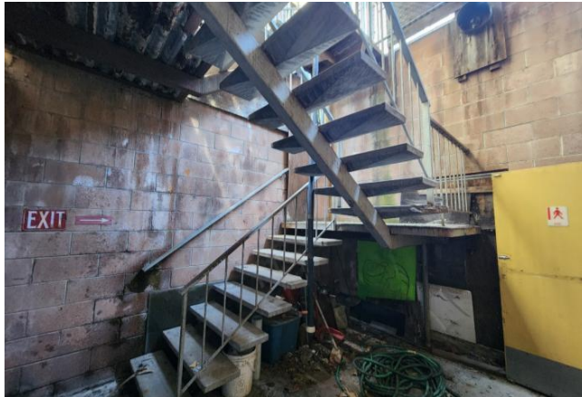
Figure 4: Oblique view of exposed stairwell at southeast corner. Looking northwest.
