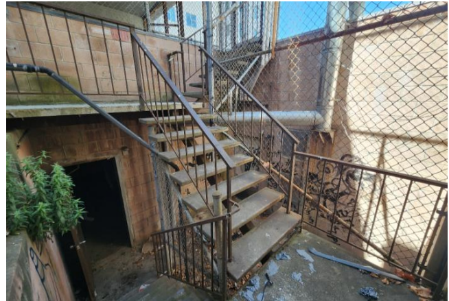
Figure 5: Oblique view of exposed stairwell at northeast corner. Looking southwest.
