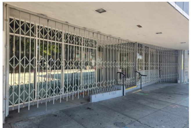
Figure 3: Storefronts at the center and south (right) end of the primary façade. Note the entrance to the south (right) storefront is set within a north-facing wall at the south (right) end of the central storefront, at the center of the image. Looking southeast.
