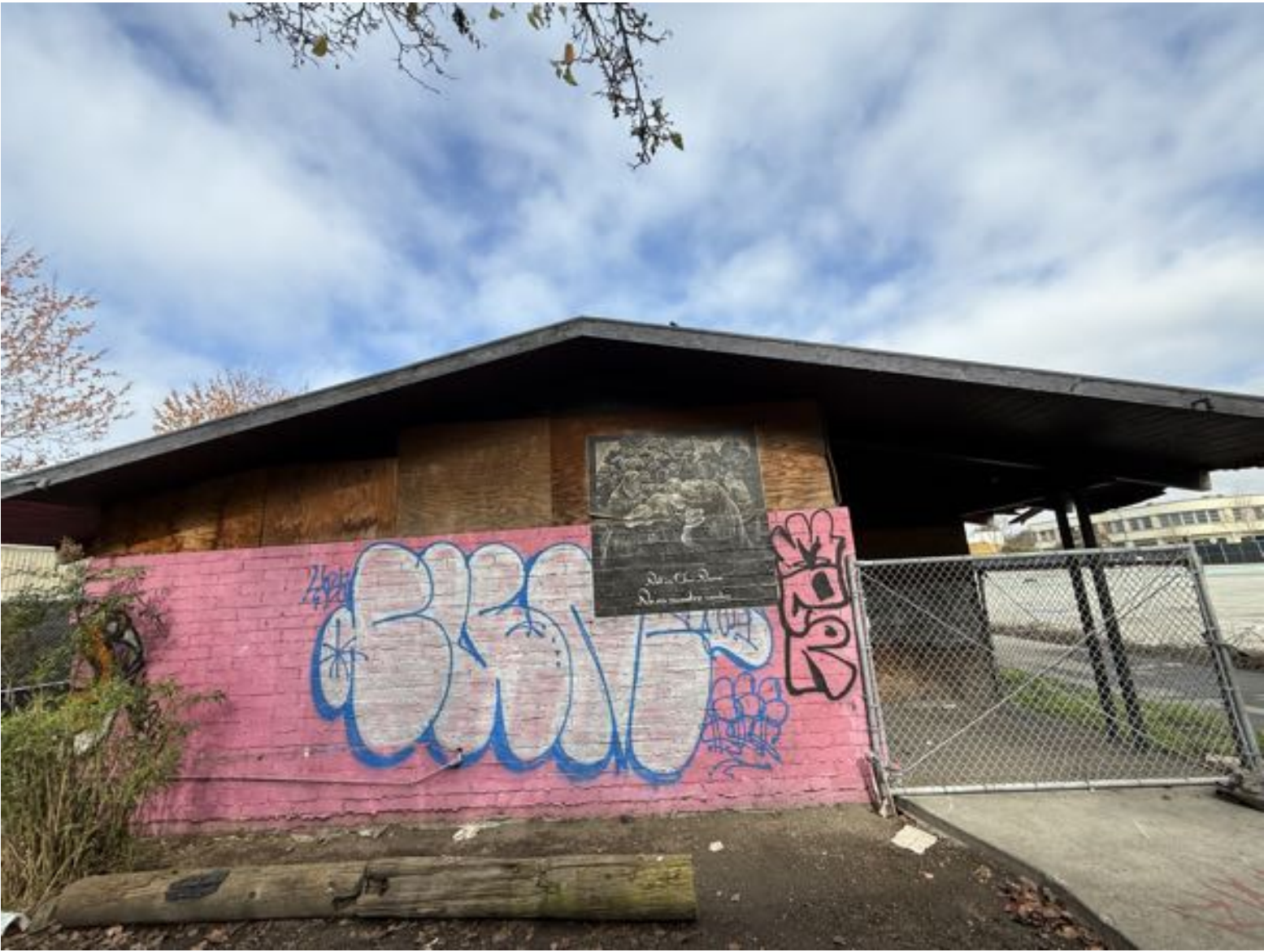
STRUCTURE TO BE DEMOLISHED - SOUTH ELEVATION
