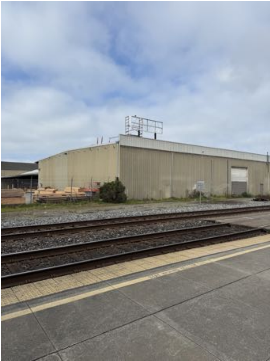
VIEW OF TRAIN TRACKS ALONG 3RD STREET
