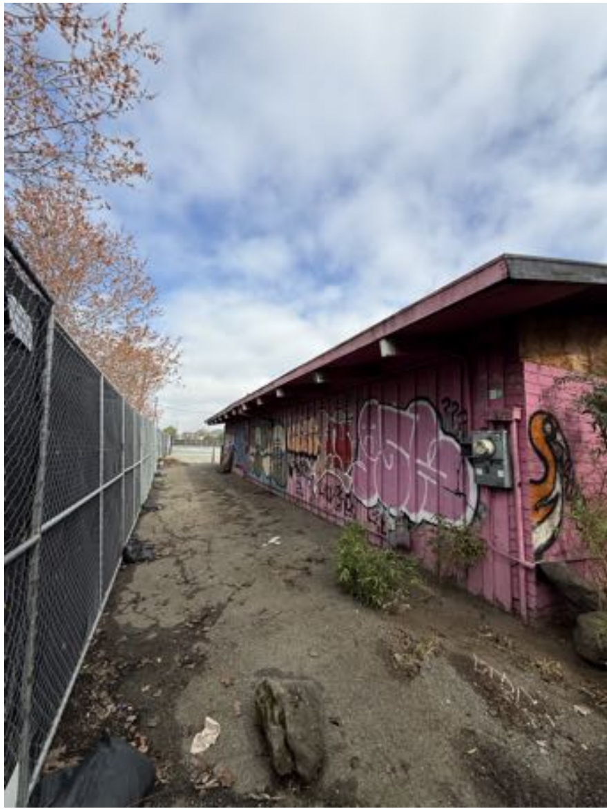
STRUCTURE TO BE DEMOLISHED - WEST ELEVATION
