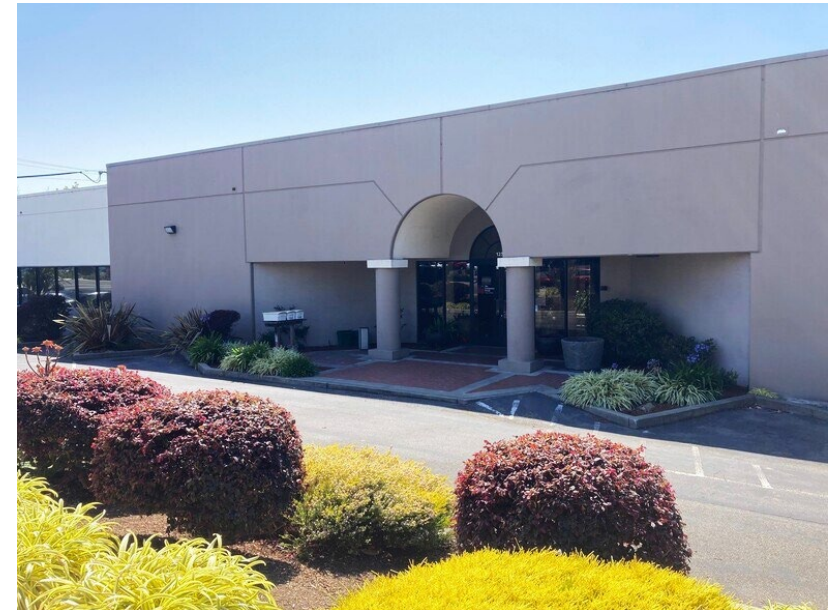
1250 Ninth Street – New Fire HQ
