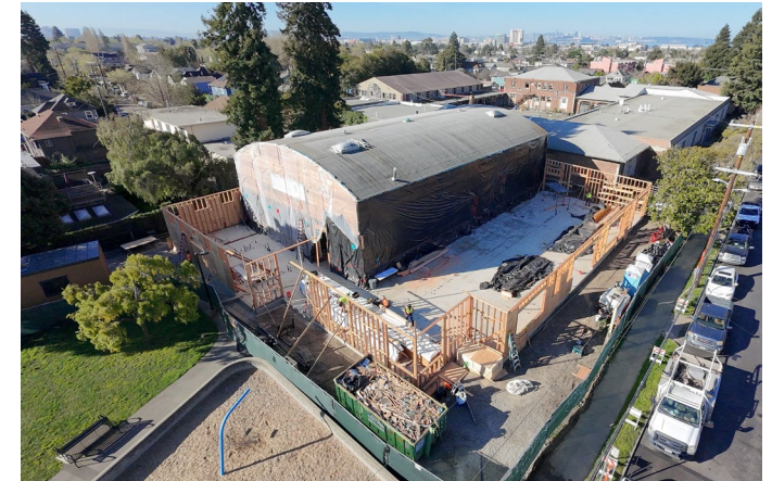
MLK Jr. Youth Services Center (under construction)
