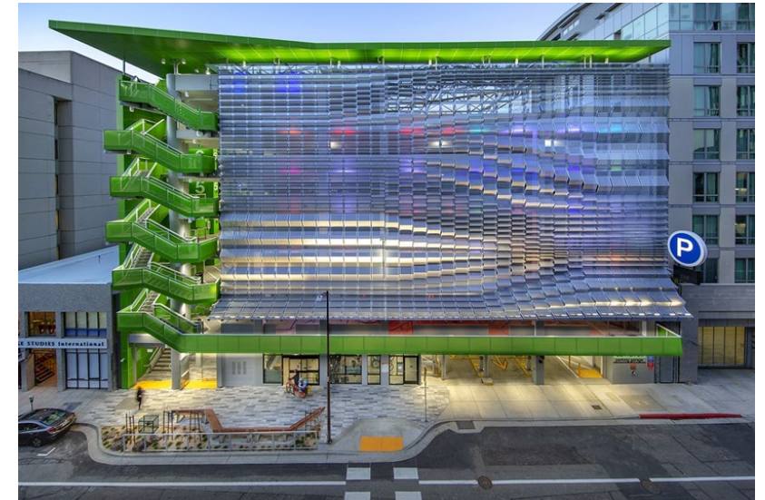
Center Street Garage
