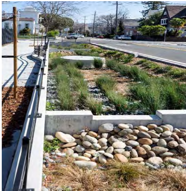
Green infrastructure installation at Woolsey Street
