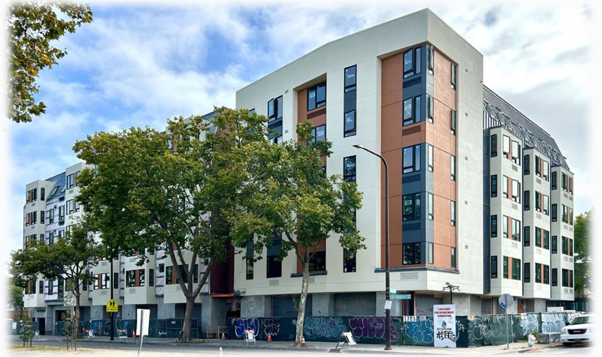
The Catalyst – BUSD Workforce Housing - 1701 San Pablo Ave, 90% complete
