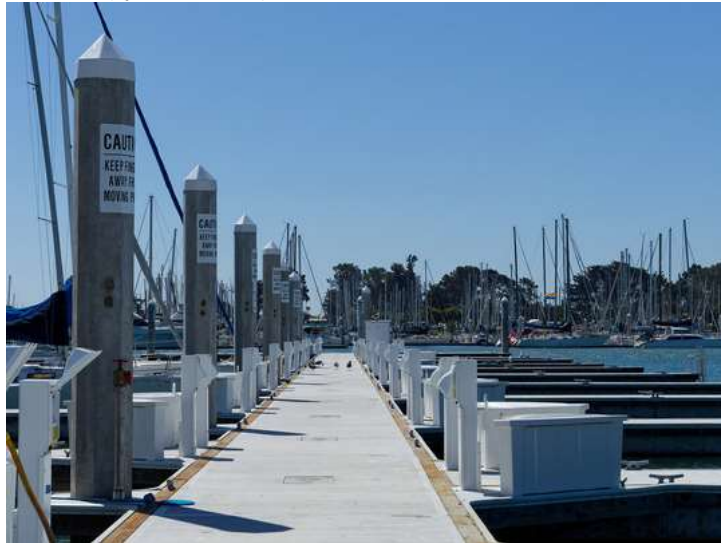
Replacement of D&E Dock
