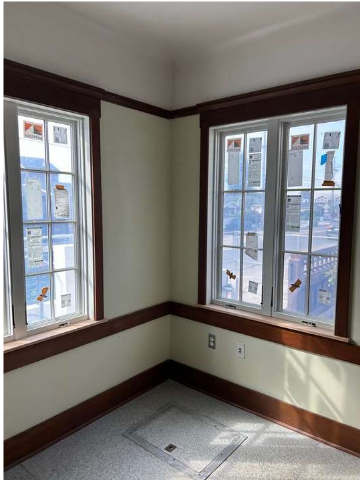
New windows installed at Fire Station No. 6
