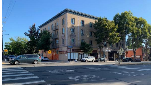
University intersection looking northeast.
