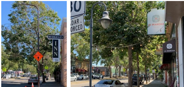
Figure 24. Existing roadway and pedestrian lighting.
