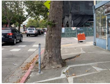
Figure 27. Many existing sidewalks are in poor condition.
