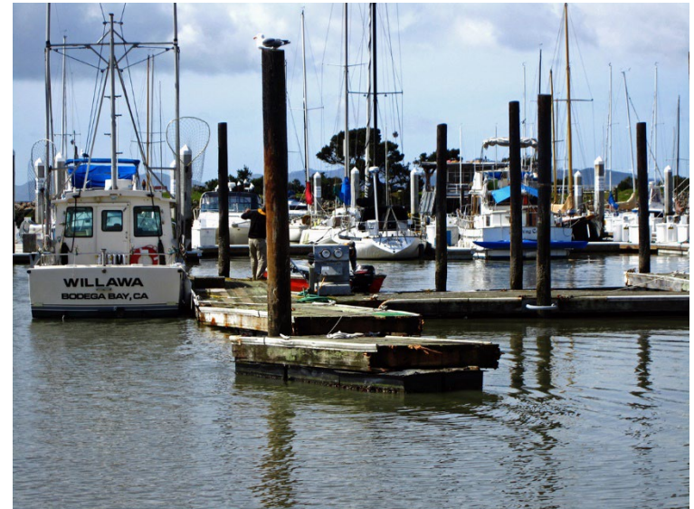
A look back: A broken dock in the marina after the March 11, 2011, tsunami entered the bay. Credit: Betsy Dorsett
