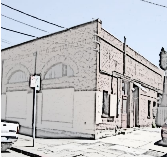
Exhibit 7. Example of unreinforced masonry construction
