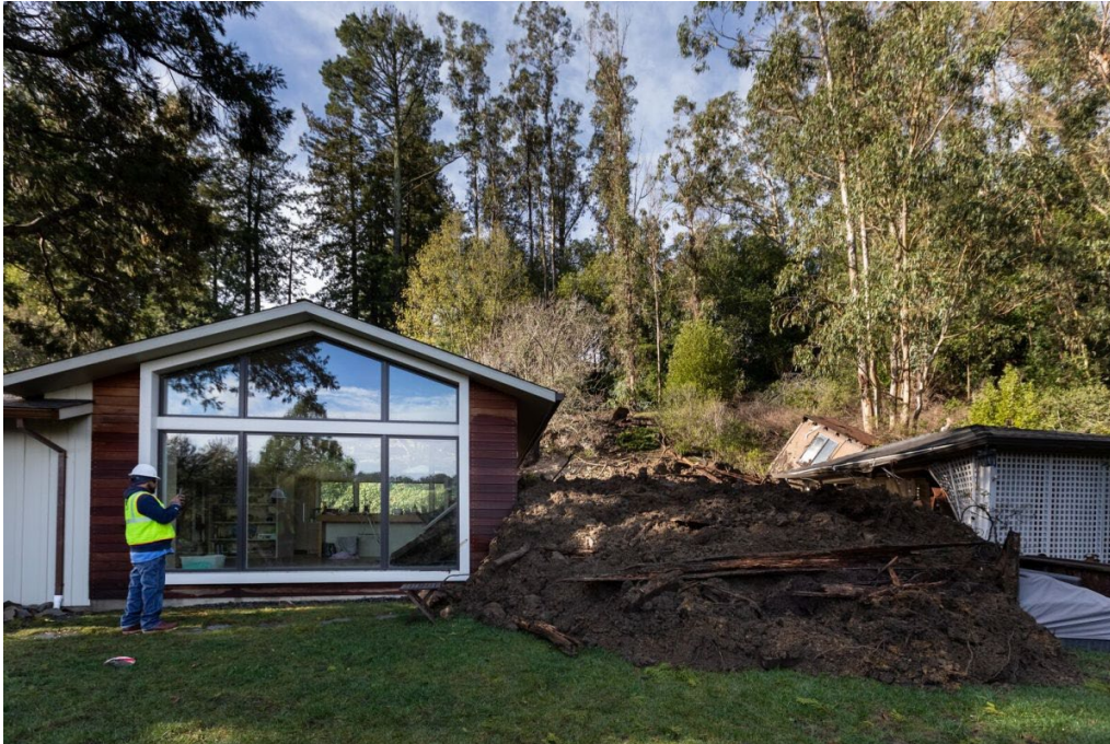
The debris flow landslide hit a home on Middlefield Road on its way down the hill from The Spiral on Jan. 16, 2023. Credit: Kelly Sullivan
